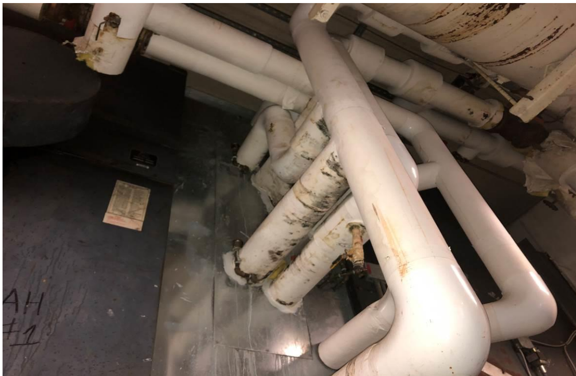
Mold – Mechanical Room
