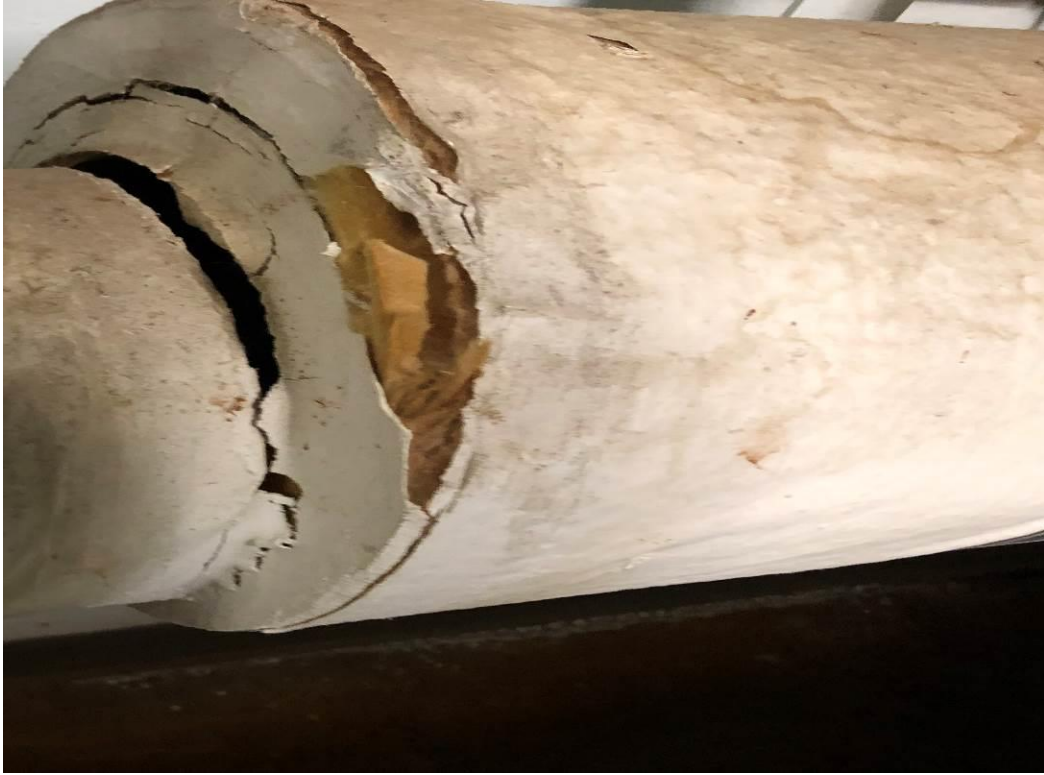
ACM in Seam Sealant on Fiberglass Pipe Fitting Above Ceiling 1 st Floor
