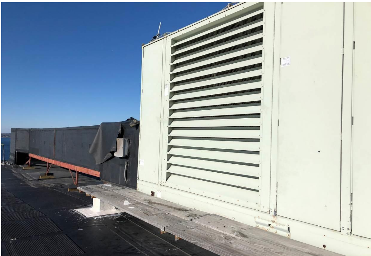
Roof Top Unit – No ACM Detected on Components
