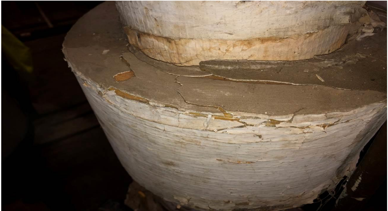
ACM Containing Gray Seam Sealant on Fiberglass Fitting- Mechanical Room
