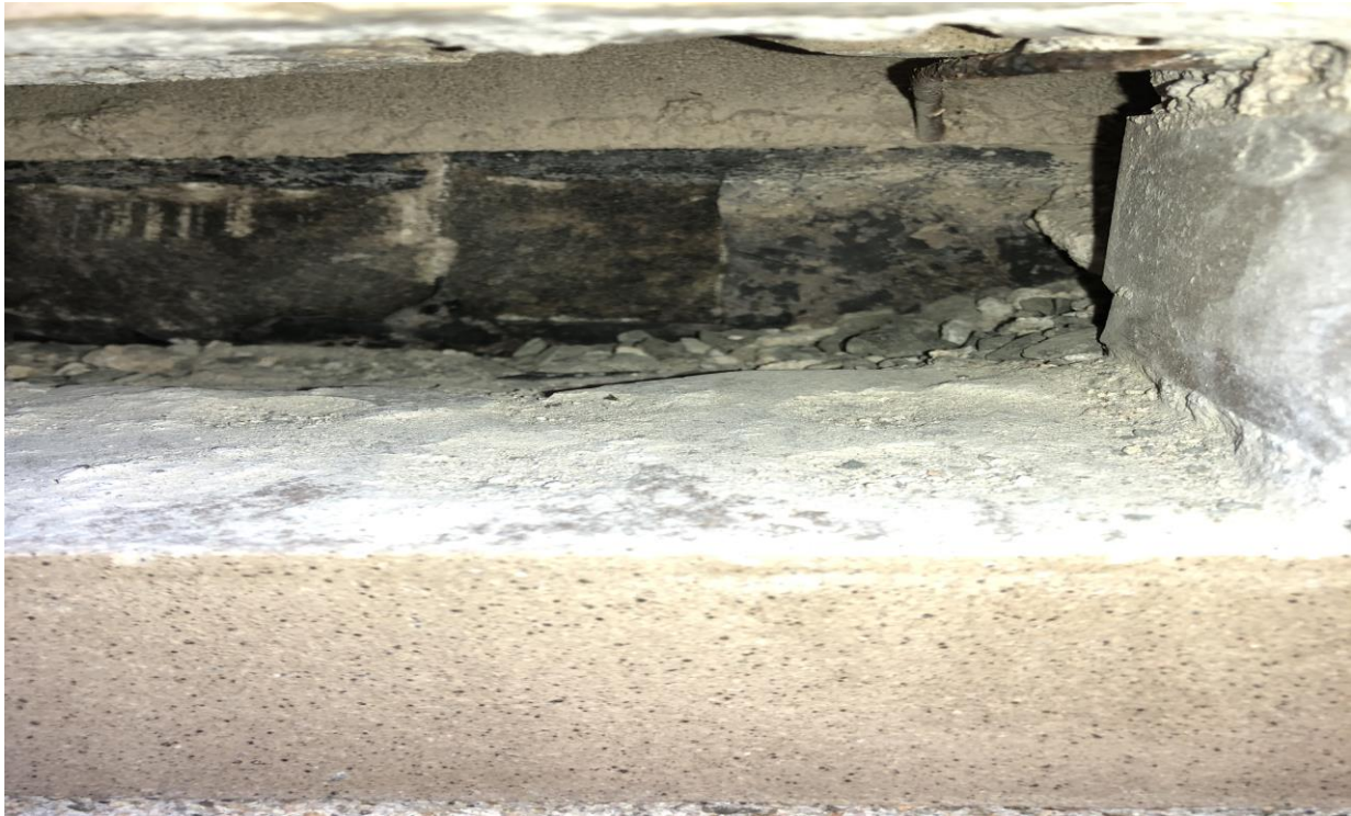
Behind Brick Cut – ACM Gray Mastic Located Behind the Flashing
