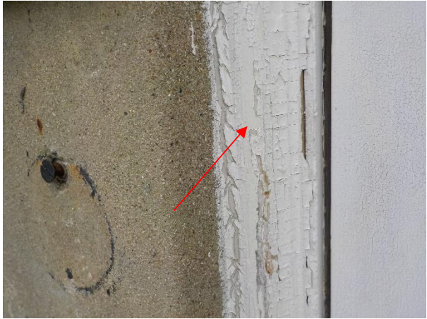
Photo #1- HA 06: Asbestos-Containing (<1% Chrysotile) Exterior White Window Caulking (Building 9).
