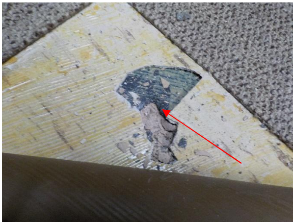
Photo #3- HA 19: 3 Layers of Asbestos-Containing (2% Chrysotile) Vinyl Floor Tiles: 12"x12" White Floor Tile with Red Streaks, Green Floor Tile and Tan Floor Tile with Non-Asbestos-Containing Mastics (Building 9).
