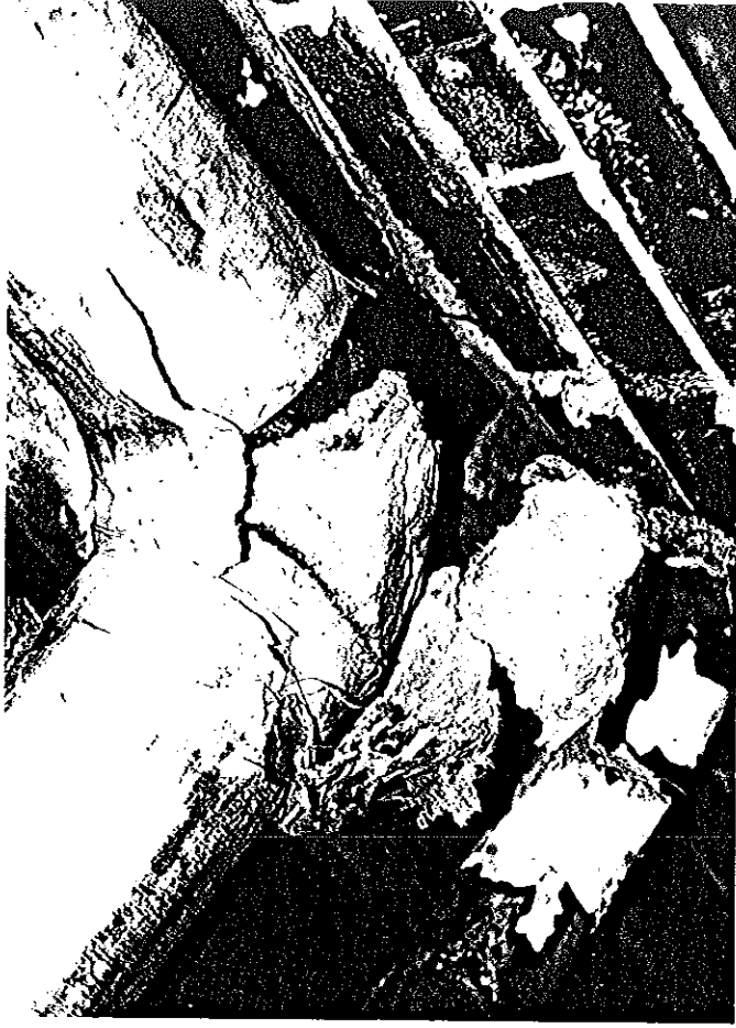
Damaged thermal Insulation in Building 1 basement
