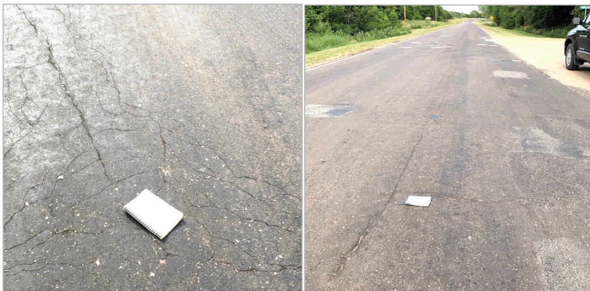
Left – Low to moderate severity fatigue cracking. Right – Typical roadway distress photograph, low severity transverse and longitudinal cracking severity, and low severity patch deterioration.
