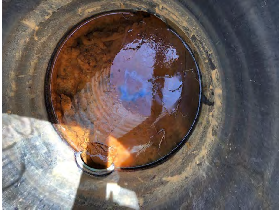
Figure 7: Photograph of biological materials in manhole for relief well RW-67A
