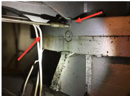
EXISTING GREASE LUBRICATION SYSTEM (UNIT 4 SHOW, UNIT 5 SIMILAR)
