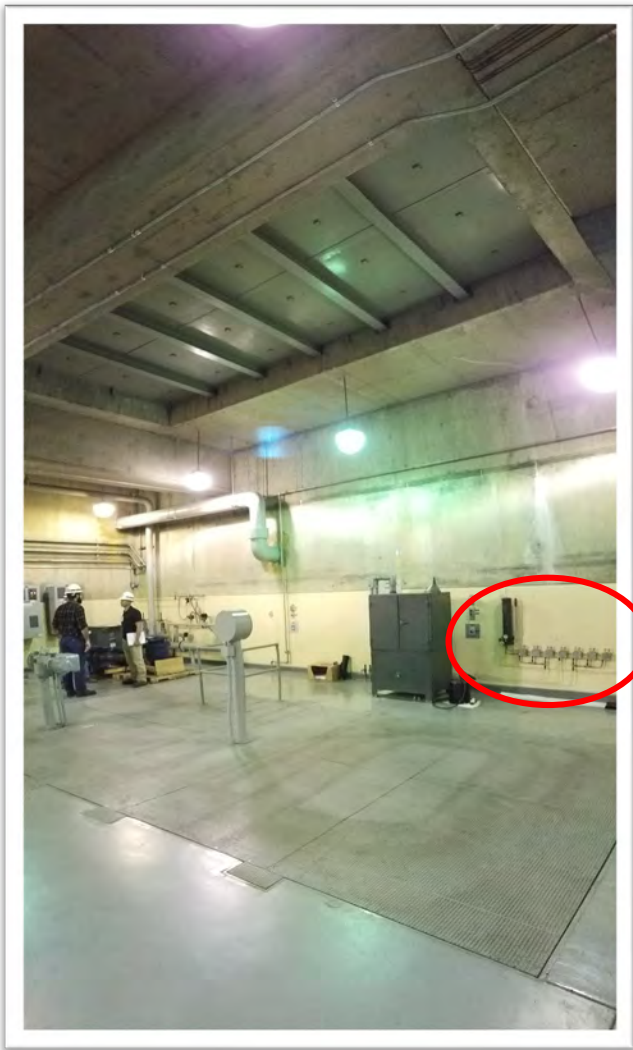
EXISTING GREASE LUBRICATION SYSTEM (UNIT 4 SHOW, UNIT 5 SIMILAR)
