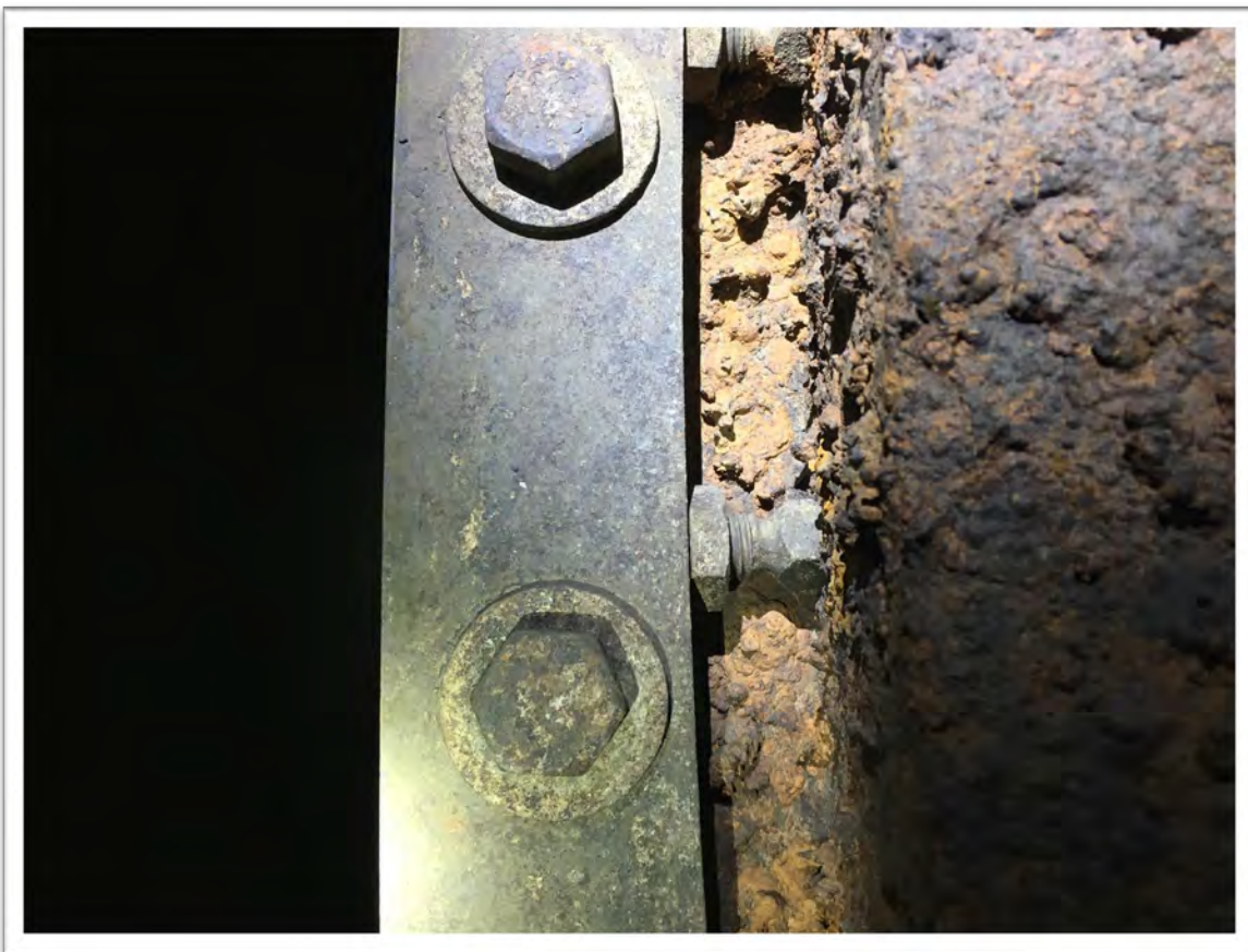
CLOSE-UP OF VALVE DISC BRONZE SEAL
