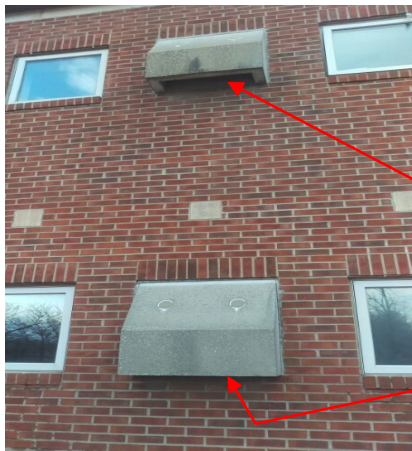
Dryer exhaust cover concrete
