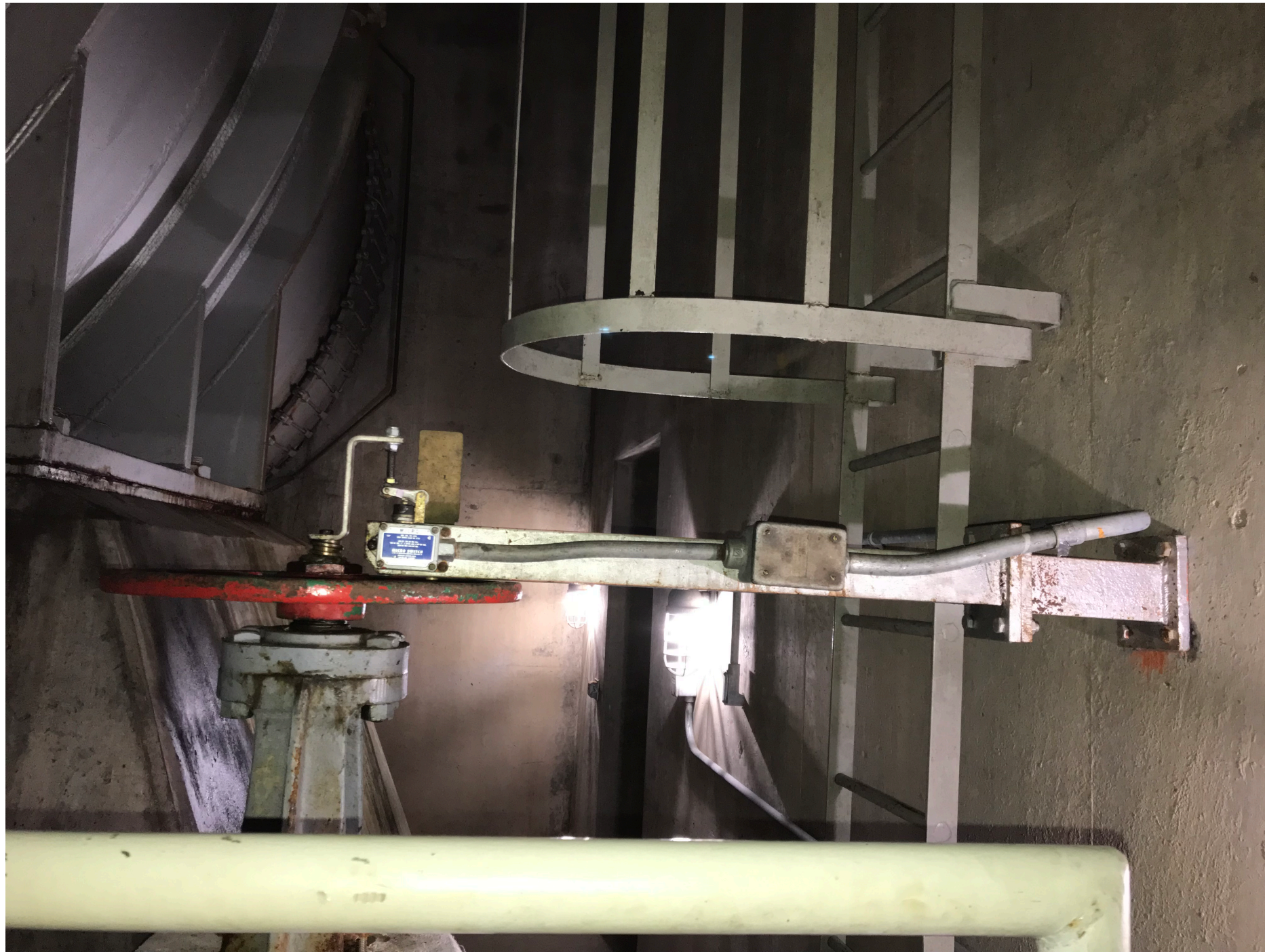
UNIT 4 Spiral Case Drain Valve Limit Switch & Conduit
