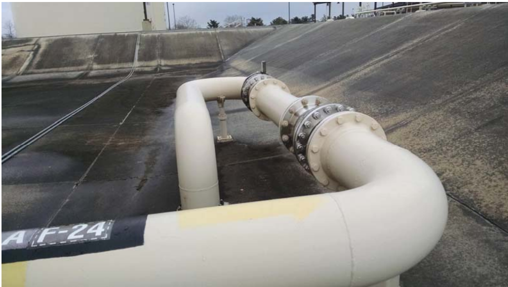
E.11 Piping Associated with Shell Nozzle D
