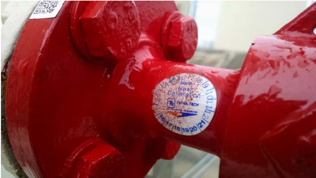
E.19 TRV Calibration Stickers Current
