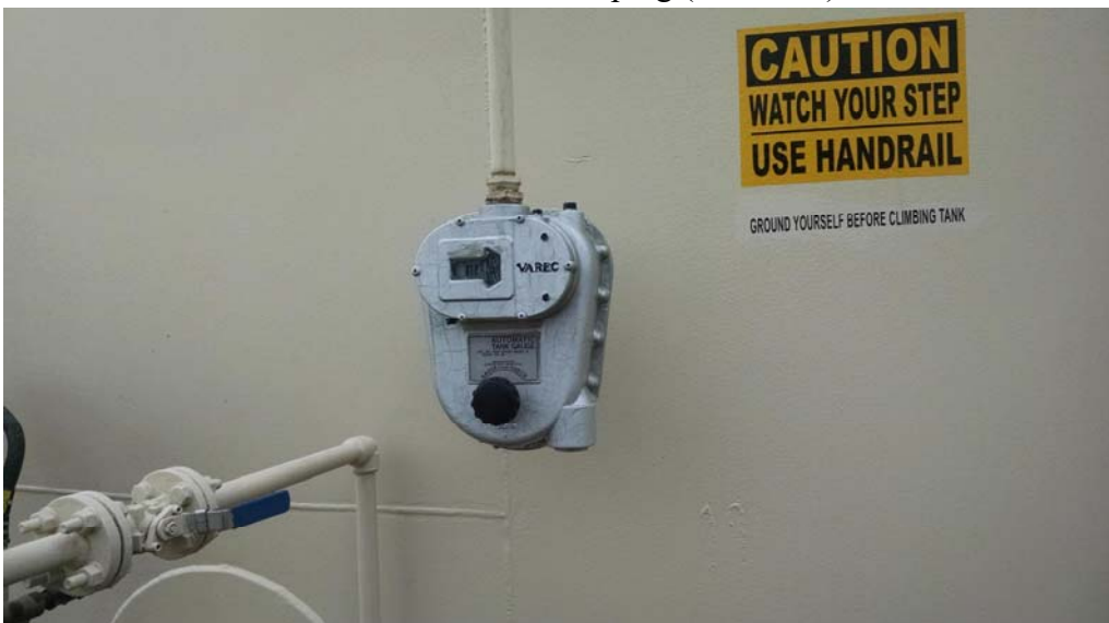
E.15 Mechanical Tank Level Gauge
