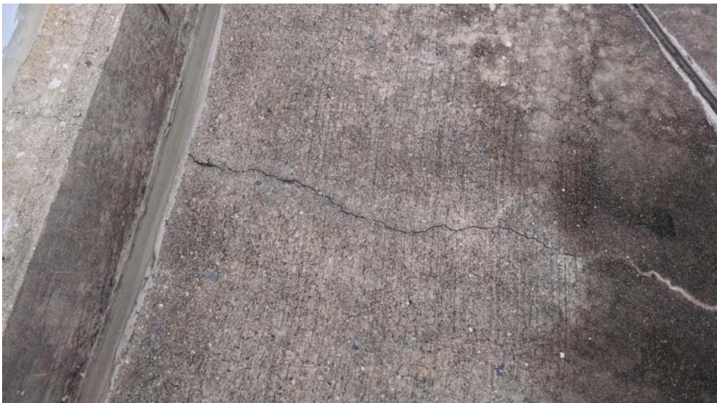
E.21 Crack in Containment Floor (Typical)
