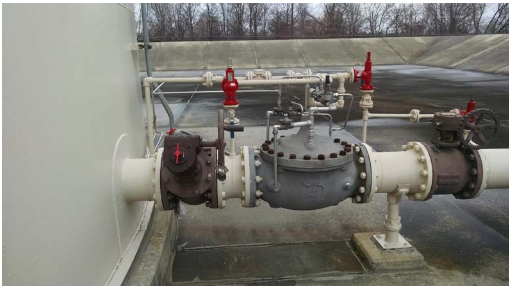
E.24 Shell Nozzle G, 10" Tank Receipt
