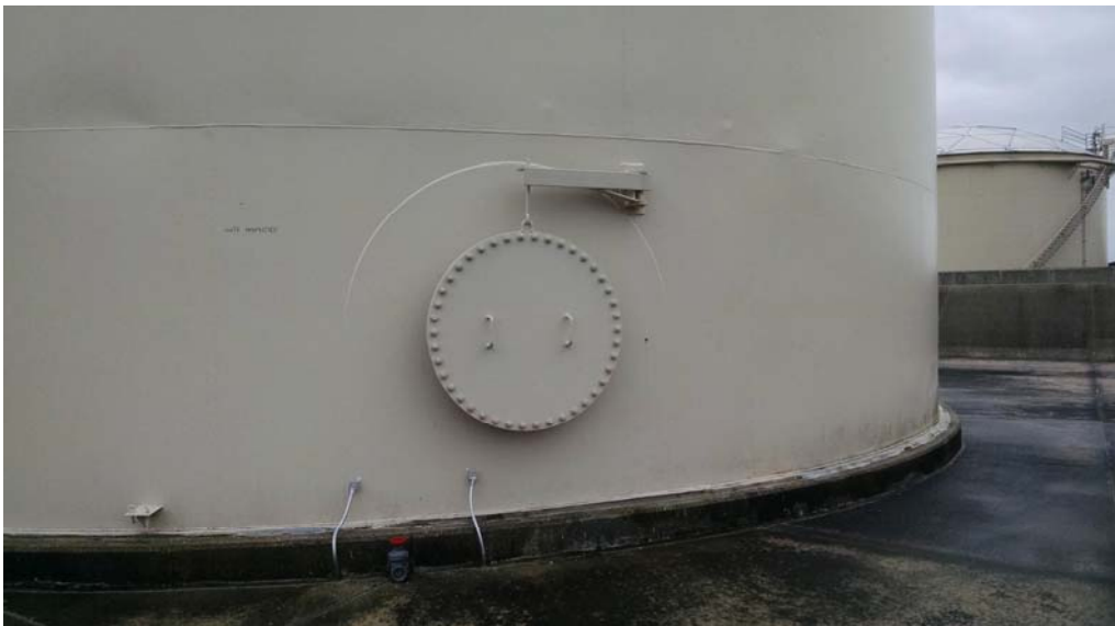
E.30 Shell Nozzle N, 36" Manhole
