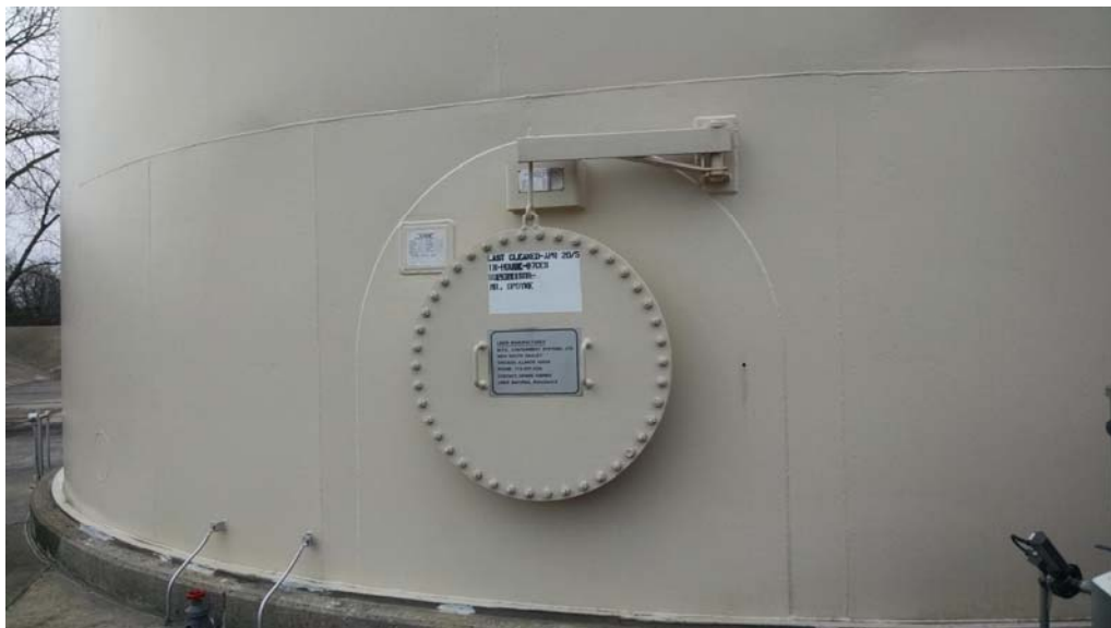
E.2 Shell Nozzle A, 36" Manhole
