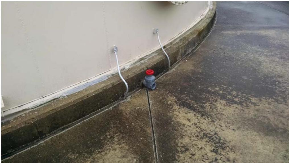
E.29 Tank Grounding and Leak Detection Port
