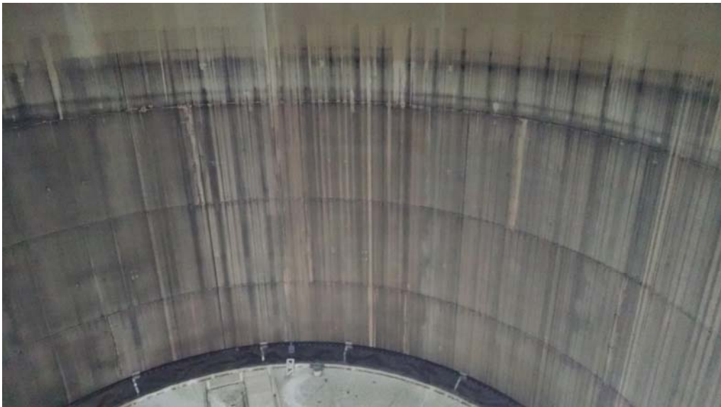
E.47 Heavy Rubber Streaking on Shell
