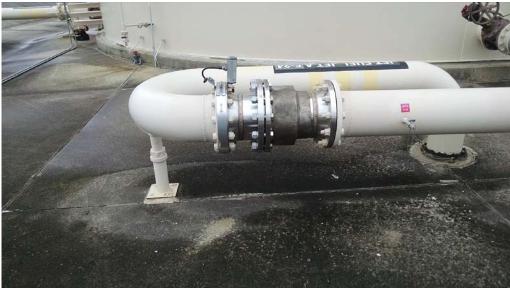
E.26 Expansion Joint (Nozzle G)
