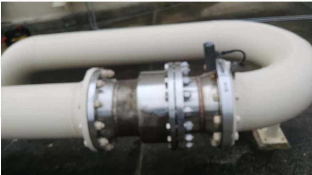
E.12 Expansion Joint Nozzle D
