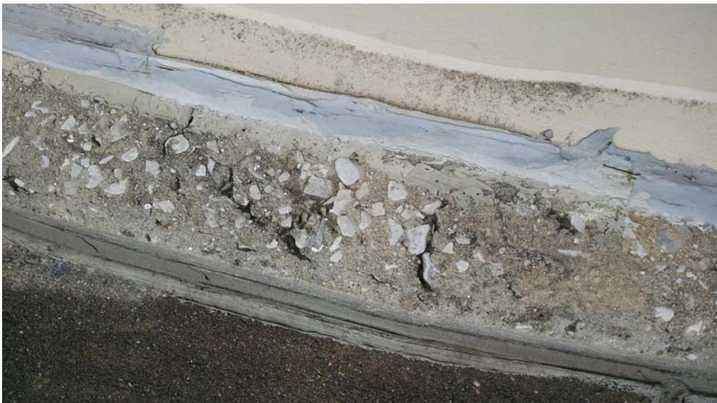
E.18 Crack in Concrete Foundation
