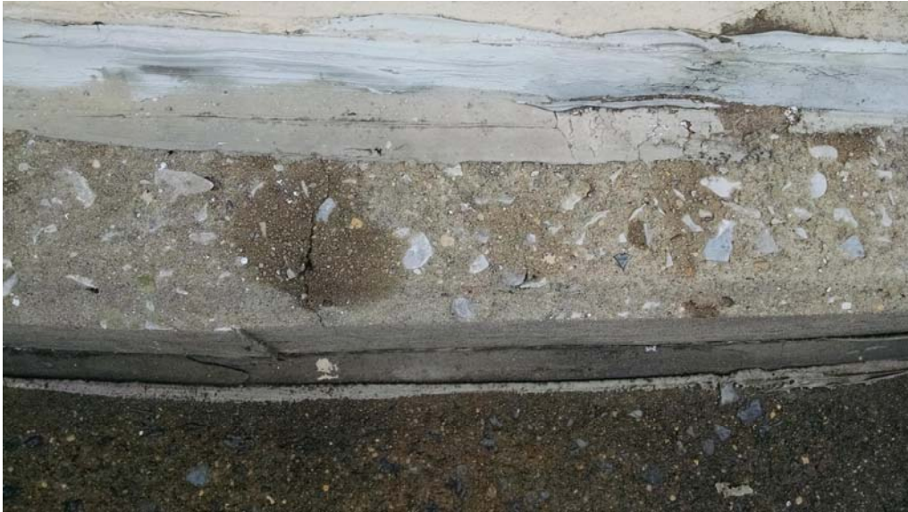
E.17 Crack in Concrete Foundation
