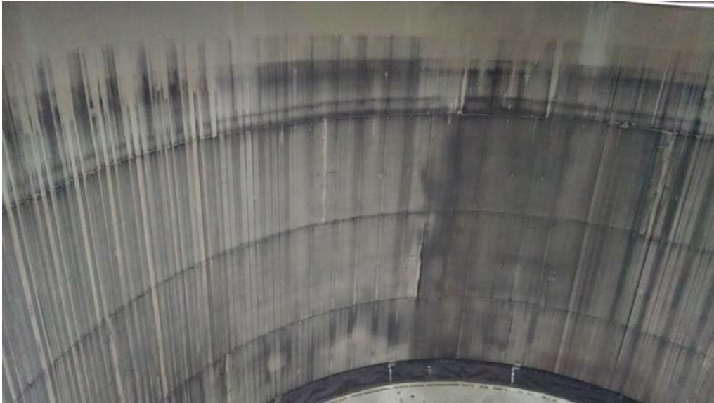
E.46 Heavy Rubber Streaking on Shell
