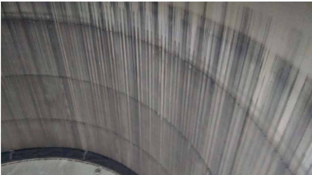
E.48 Heavy Rubber Streaking on Shell
