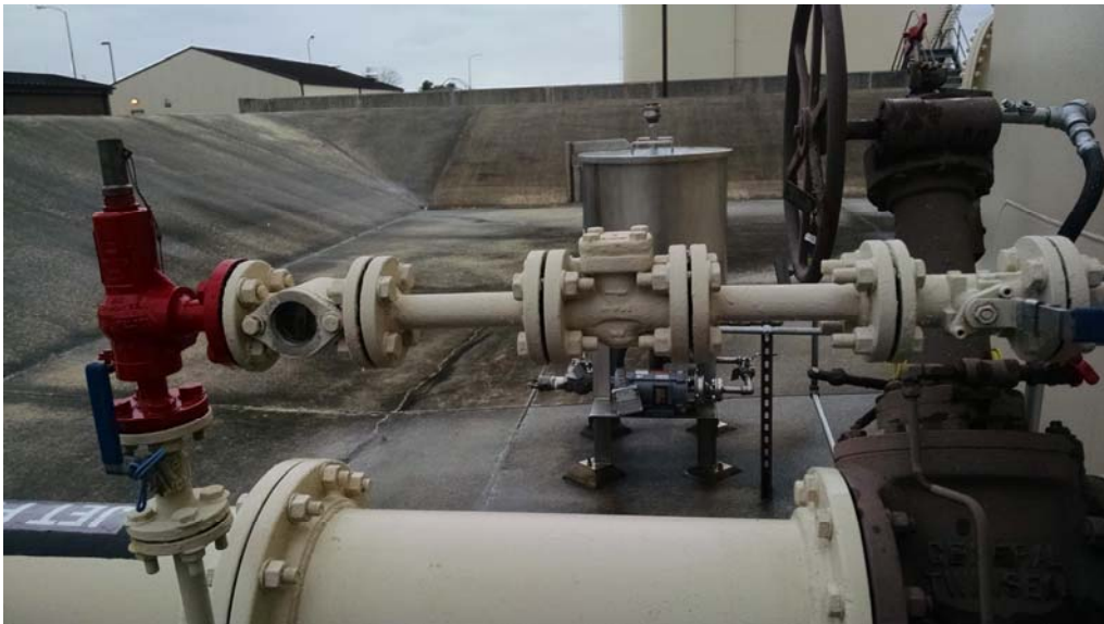
E.14 Thermal Relief Piping (Nozzle D)
