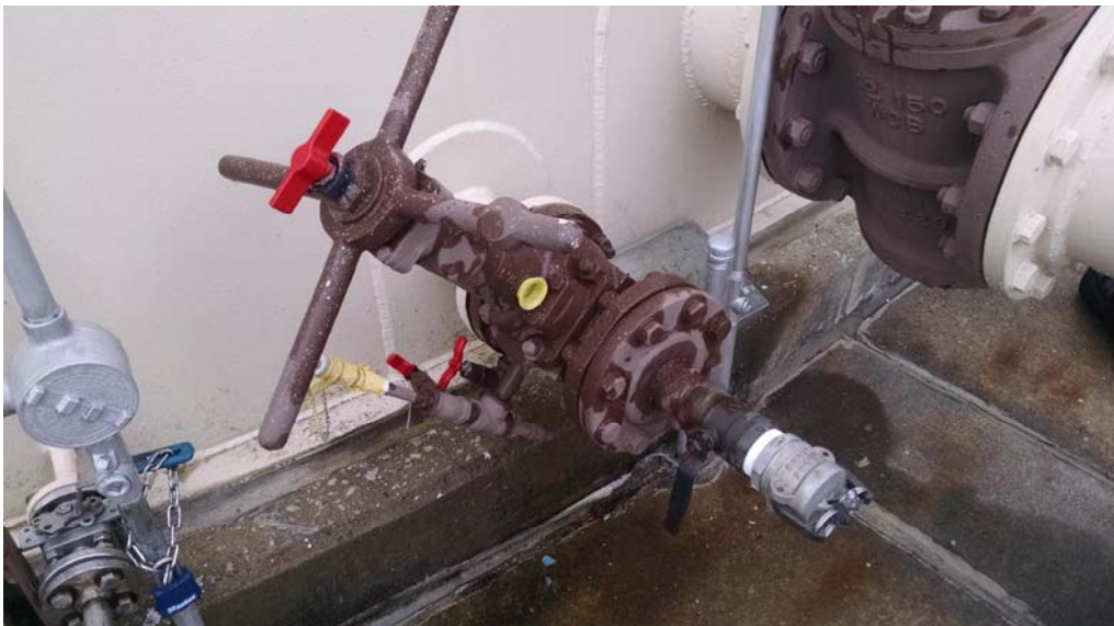
E.9 Shell Nozzle C, 4" Low Point Suction
