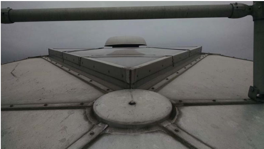
E.41 Fixed Roof (Geodesic Dome)
