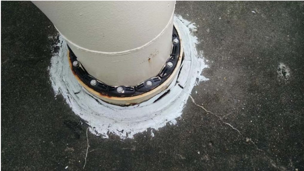
E.13 Piping Penetration into Containment Floor
