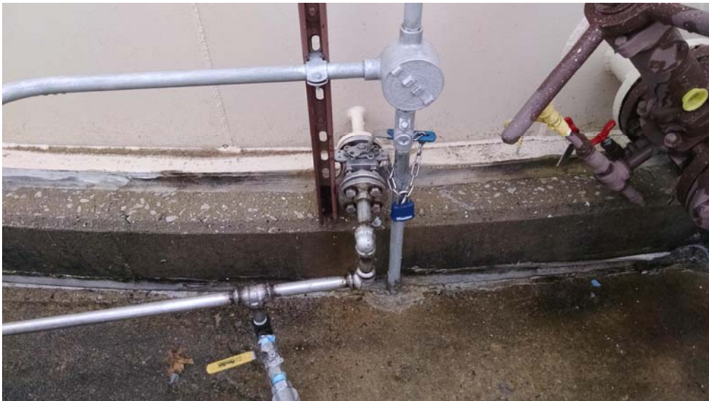
E.8 Shell Nozzle B, 1" Water Draw
