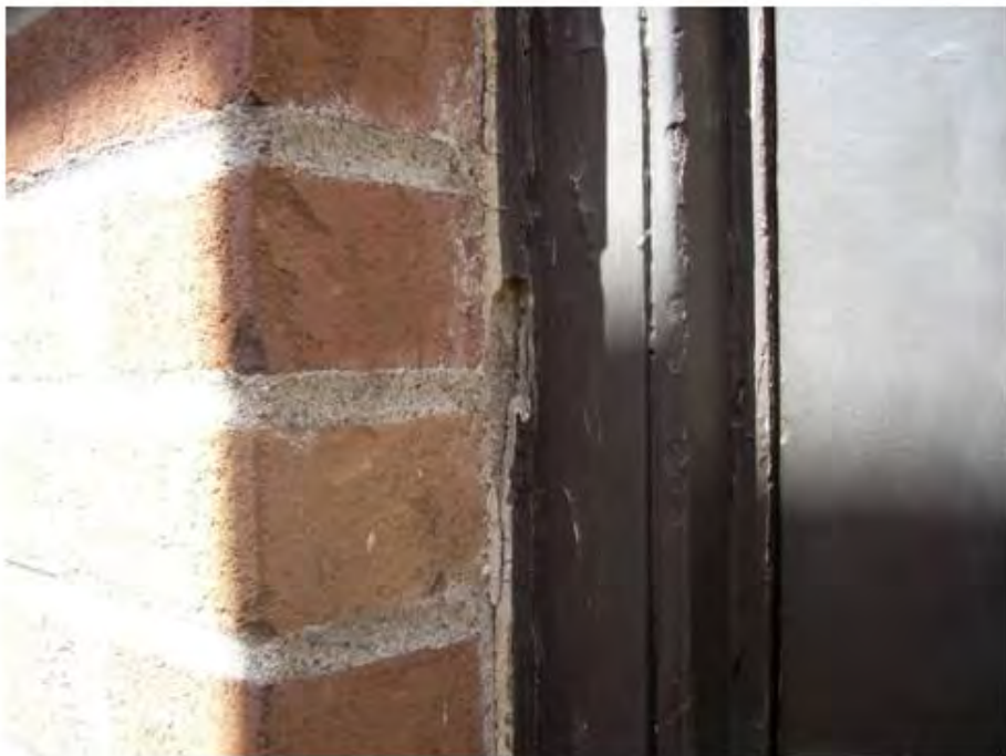
Door Frame Caulking, Sample 71A
