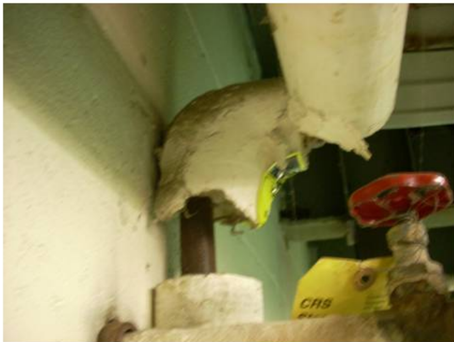
Fitting Insulation, Sample 18A
