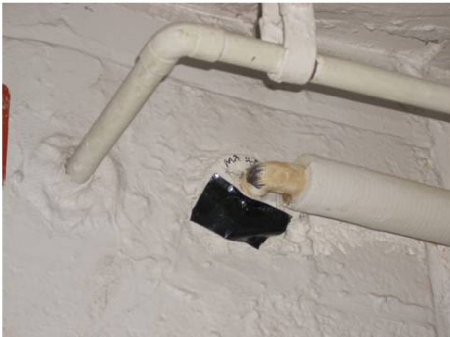
Pipe Insulation, Sample 4
