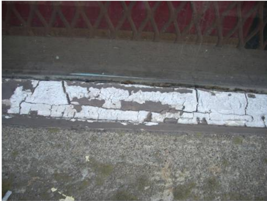
Exterior Window Caulking, Sample 13B
