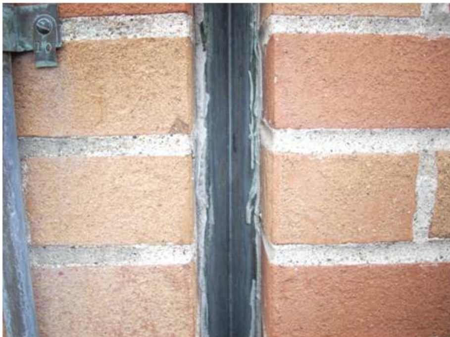
Expansion Joint Caulking, Sample 22A
