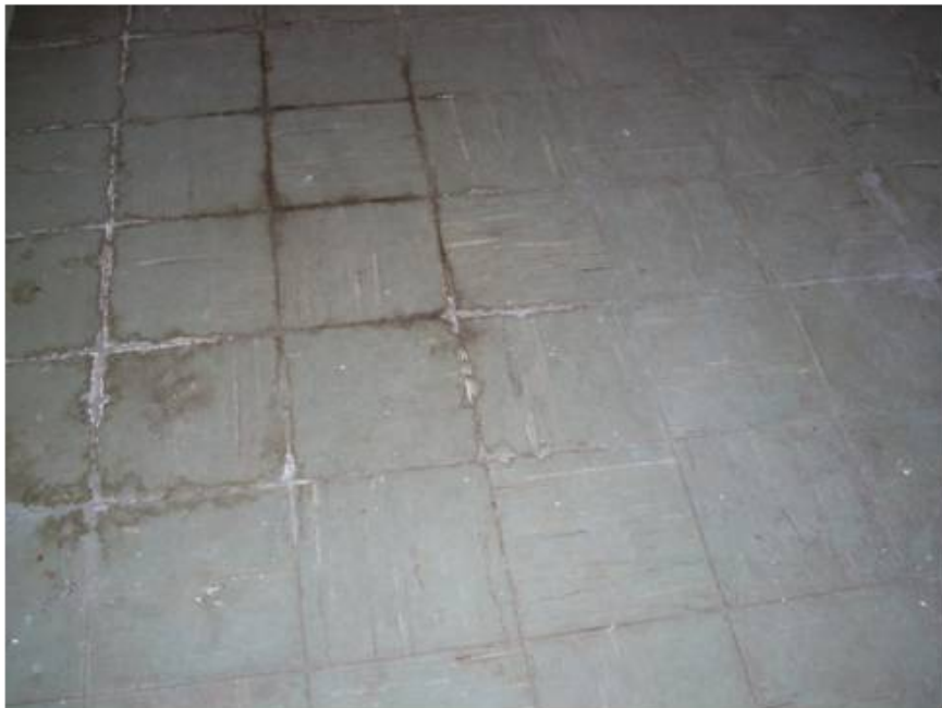
12"x12" Green Floor Tile and Mastic, Samples 4A and 5A
