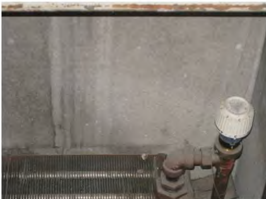
Transite Heater Panel, Sample 13A
