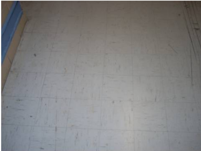
9"x9" White Floor Tile and Mastic, Samples 23A and 24A
