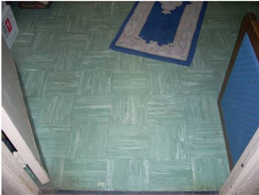
Mastic Associated with 9"x9" Green Floor Tile, Sample 27A
