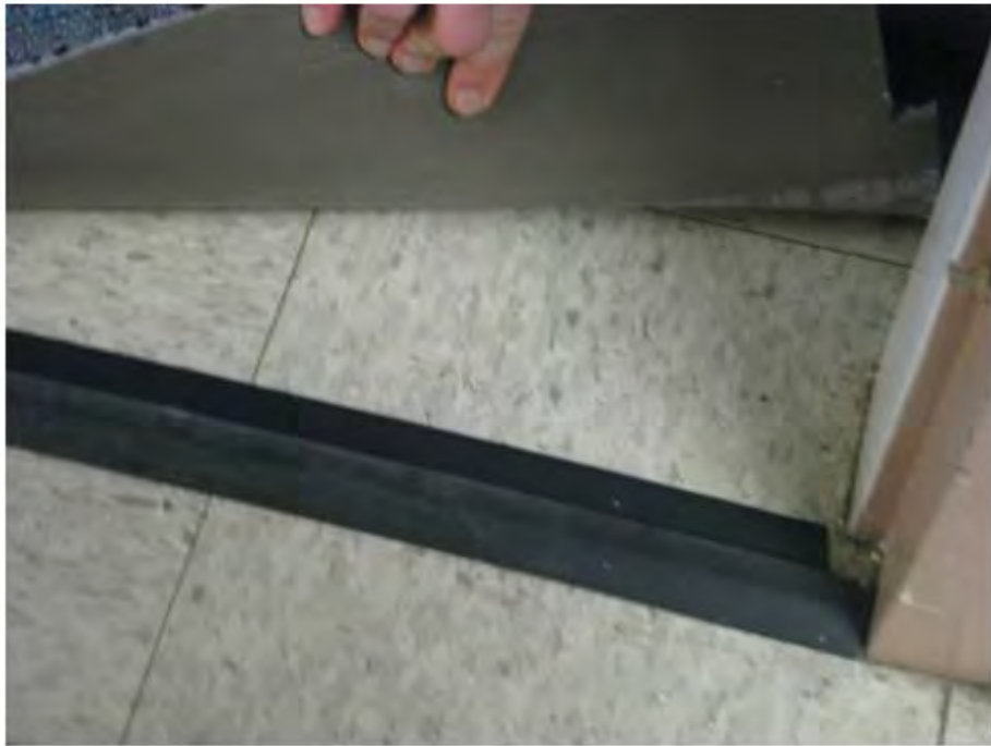
12"x12" Floor Tile and Mastic (5 th Floor Old), Samples 41A and 42A
