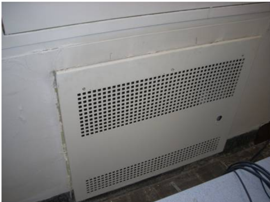
Transite Covering Inside Radiator, Sample 16A
