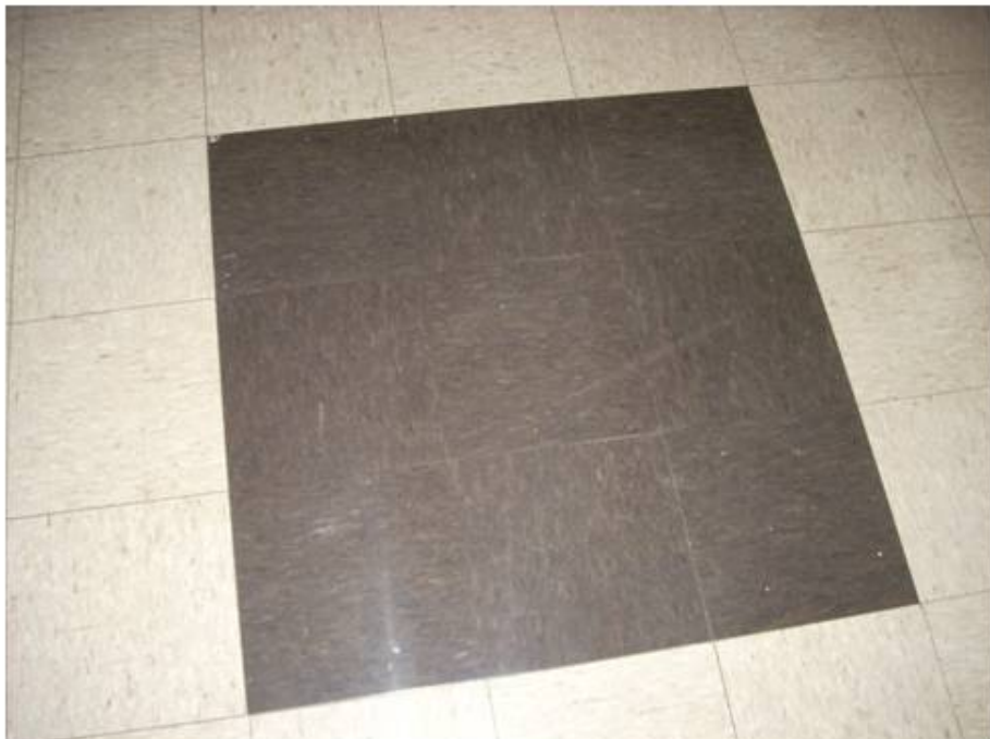
12"x12" Black Floor Tile and Mastic, Samples 13A and 14A
