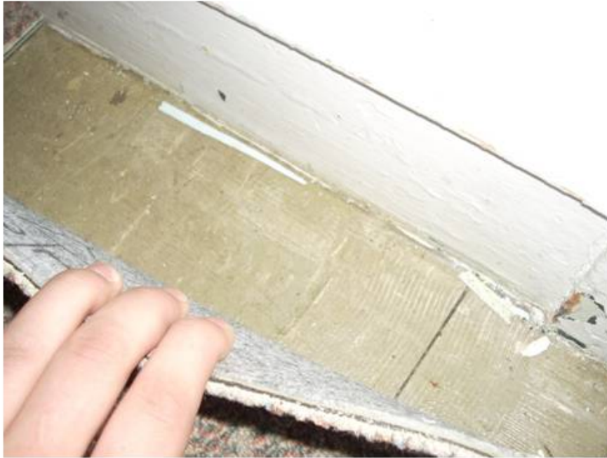
12"x12" Green Floor Tile and Mastic Underneath Carpet, Samples 17A and 18A
