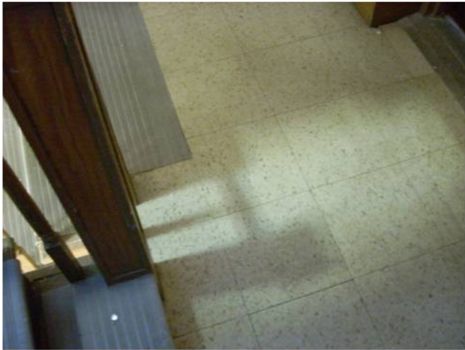
12"x12" Beige Floor Tile and Mastic, Samples 3A and 4C
