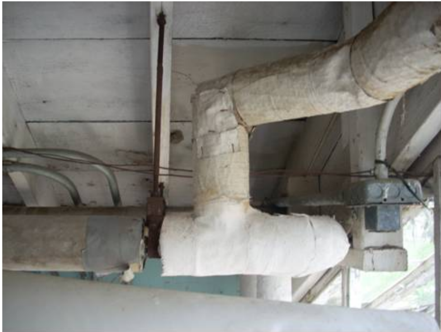
Pipe Insulation, Sample 1A Elbow Insulation, Sample 2A
