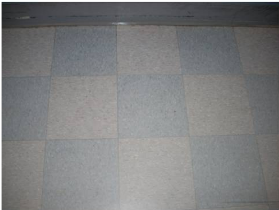
Mastic Associated with 12"x12" Blue/Gray Floor Tile, Sample 11B
