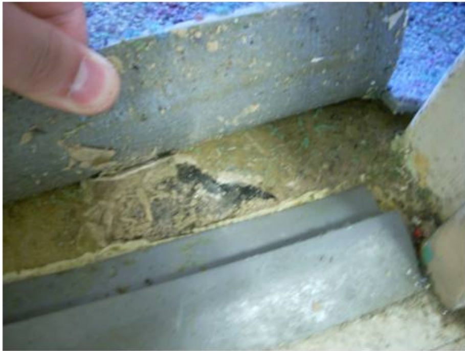
12"x12" Floor Tile Underneath Carpet, Sample 44A
