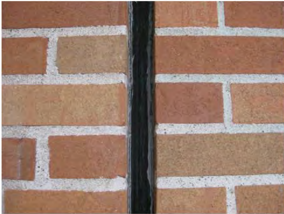
Expansion Joint Caulk, Sample 72A
