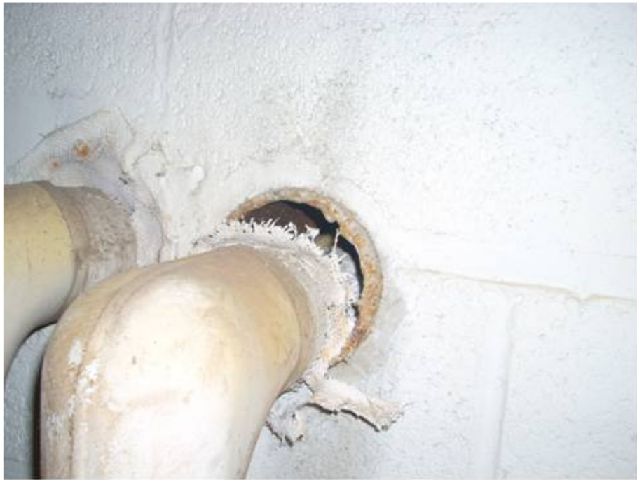
Pipe Insulation Inside Wall Cavity, Sample 1
