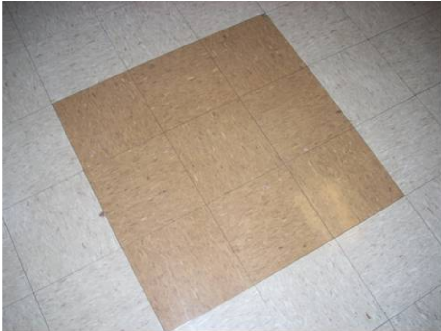
12"x12" Orange Floor Tile and Mastic, Samples 15A and 16A
