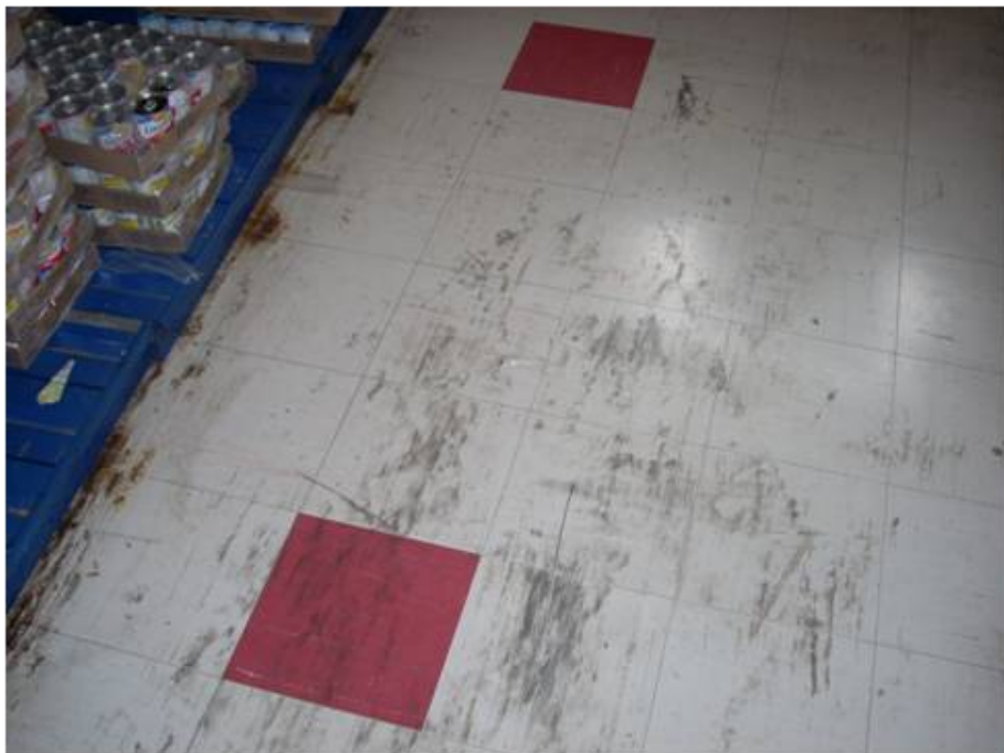
12"x12" Red Floor Tile and Mastic, Samples 35A and 36A 12"x12" Bright White Floor Tile and Mastic, Samples 37A and 38A
