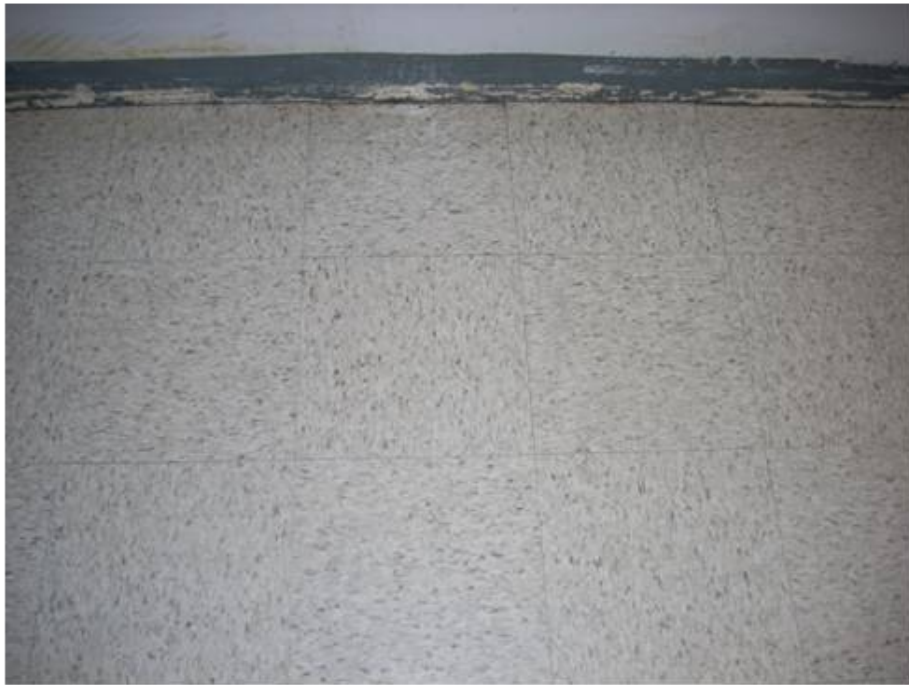
Mastic Associated with 12"x12" Shelter White Floor Tile, Sample 2A
