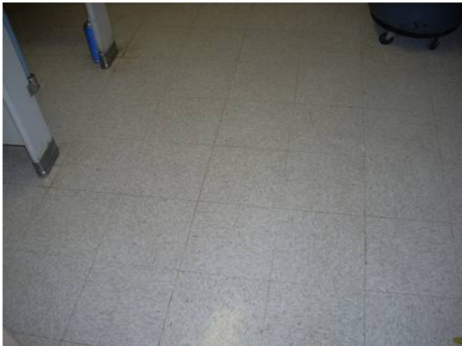
Mastic Associated with 12"x12" White with Gray Streaks Floor Tile, Sample 10C
