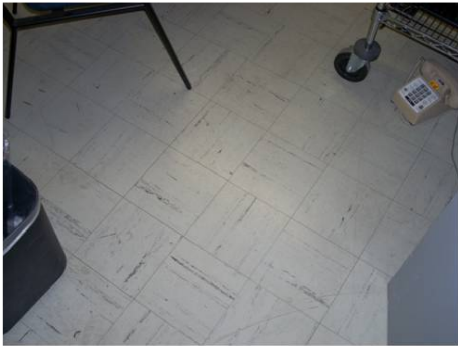
9"x9" White Floor Tile and Mastic, Samples 6A and 7A
