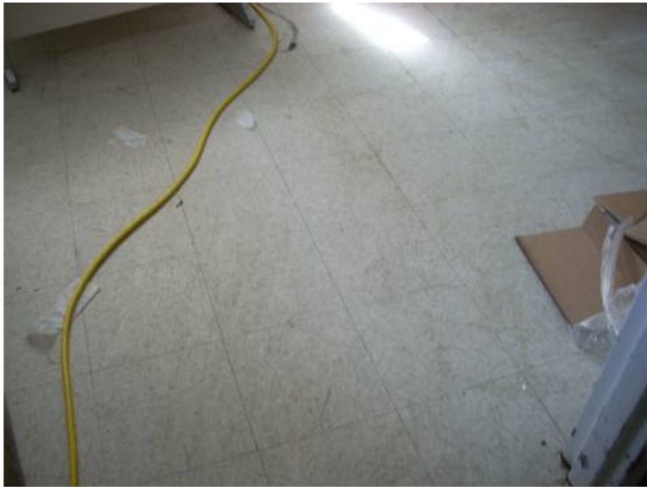
12"x12" Basement Floor Tile and Mastic, Samples 49A and 50A
