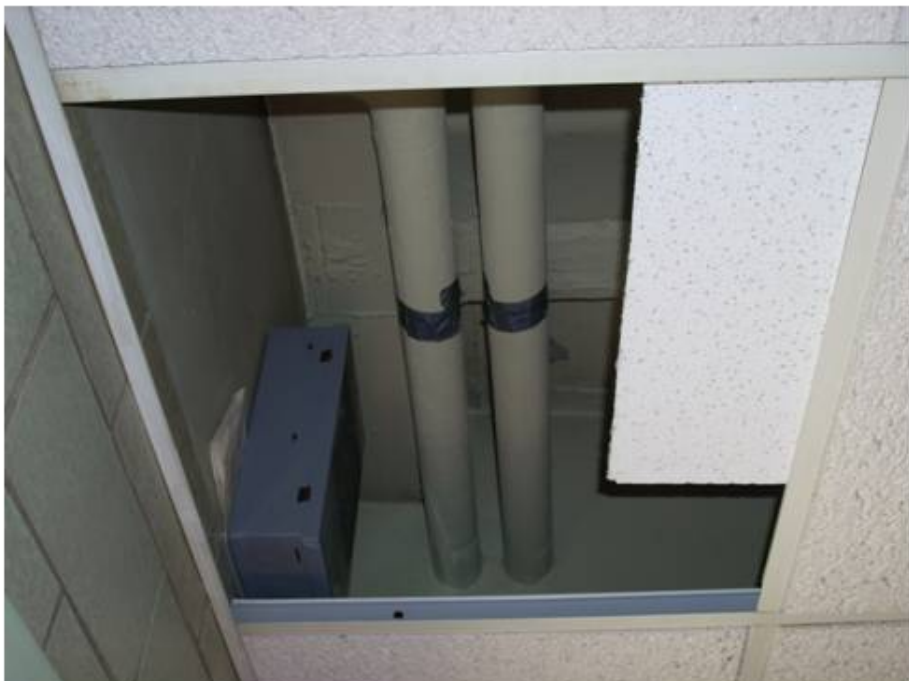
4" Pipe Insulation Above Ceiling, Sample 23A
