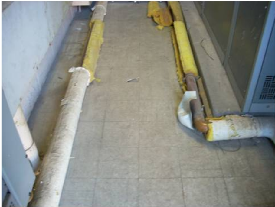
9"x9" Gray Floor Tile and Mastic, Samples 1A and 2A
