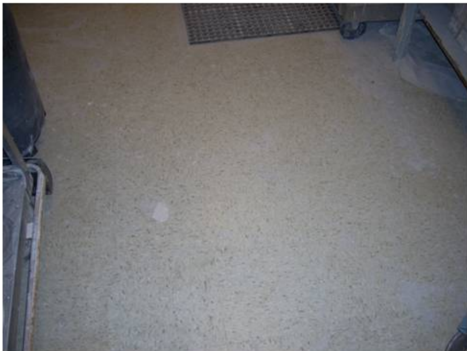
Mastic Associated with 12"x12" Light Green with Brown Spots Floor Tile, Sample, 47A
