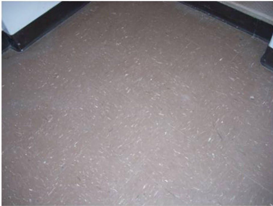
12"x12" Brown Floor Tile and Mastic, Samples 20A and 21A
