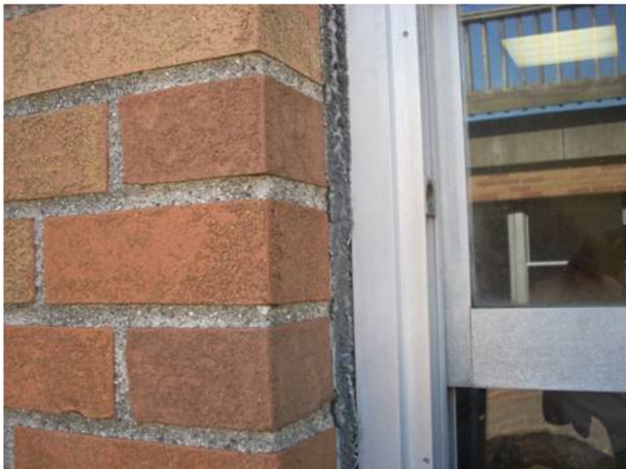
Exterior Window Caulk, Sample 11A
