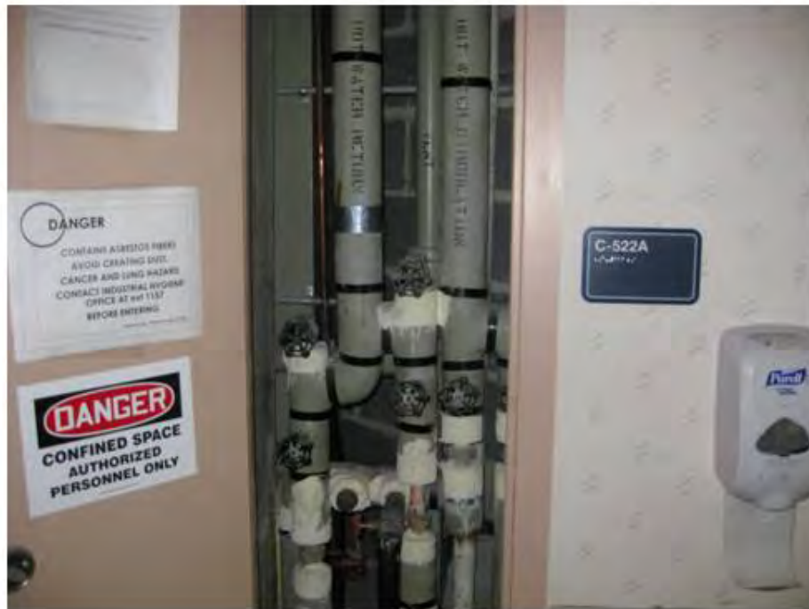
4" Pipe Insulation, Sample 17A
