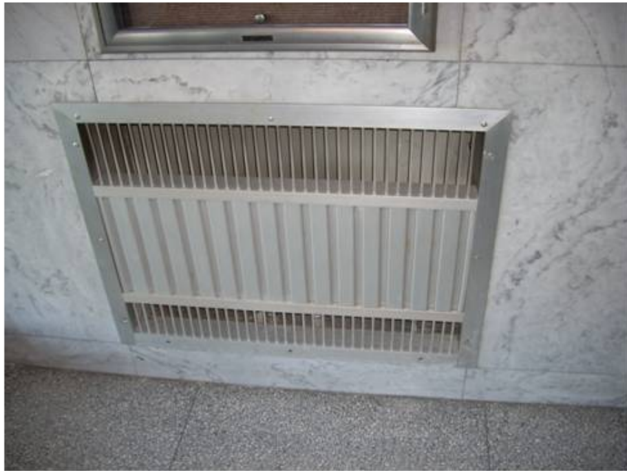
Transite Covering Inside Heater, Sample 18A
