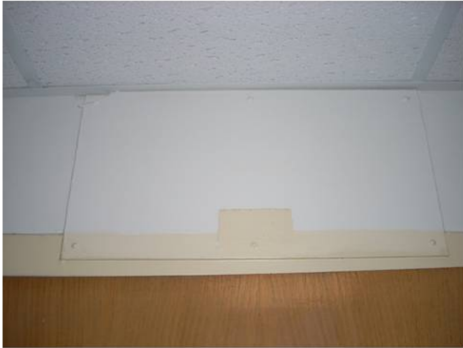
Transite Panel Above Door – Identified in previous survey and verified in the field
