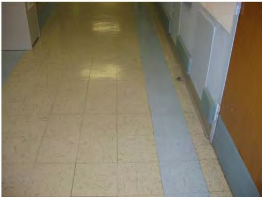
12"x12" Floor Tile and Mastic (5 th Floor New), Samples 39A and 40A
