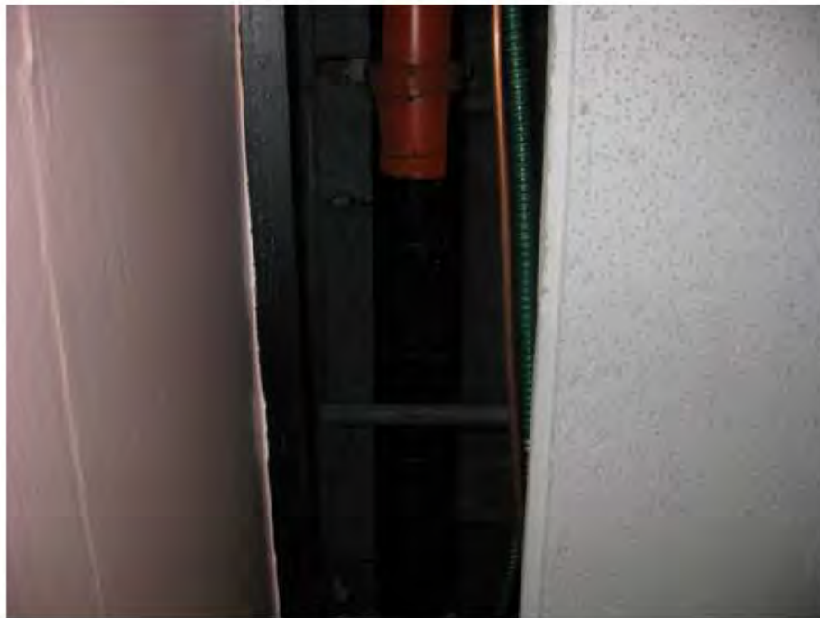
Black Cork Pipe Insulation, Sample 22A
