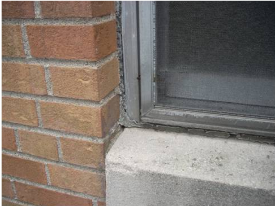
Exterior Window Caulking, Sample 44A
