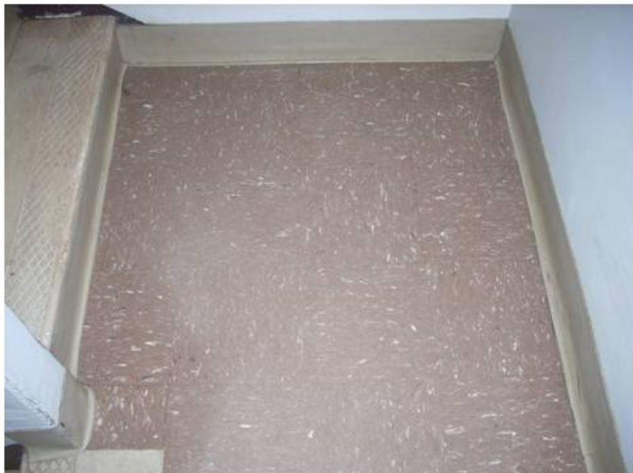
12"x12" Brown Floor Tile and Mastic, Samples 14A, 15A
