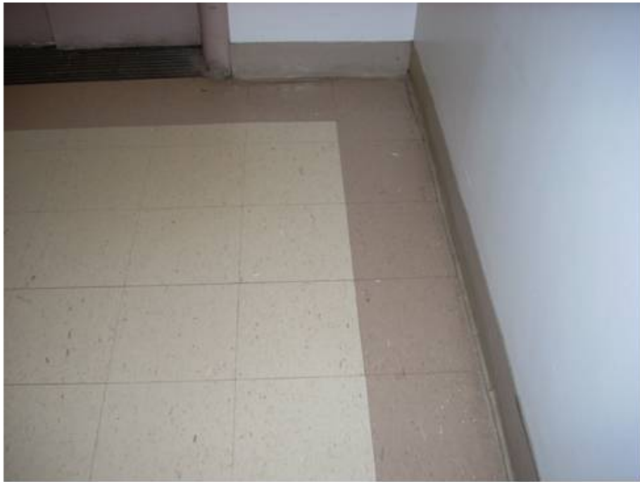
Mastic Associated with 12"x12" Tan and Brown Floor Tile, Samples 8A and 28A
