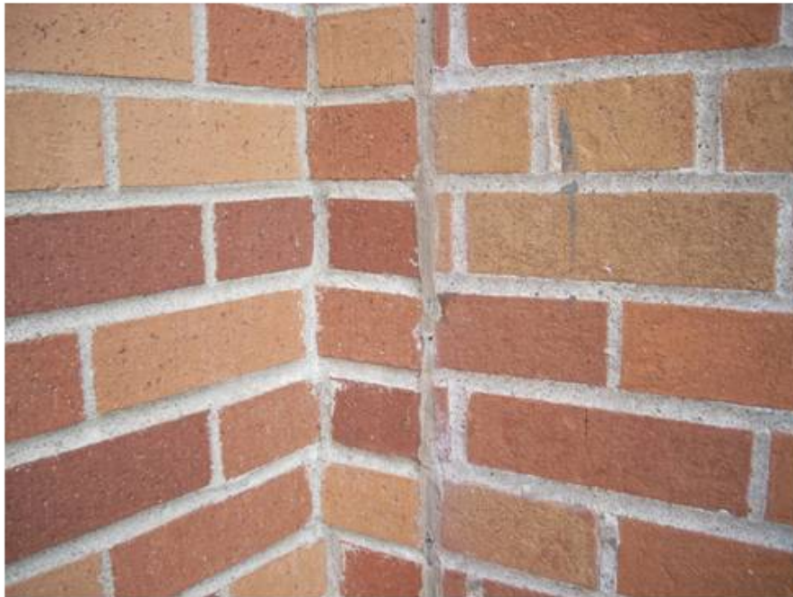
Exterior Expansion Joint, Sample 31B
