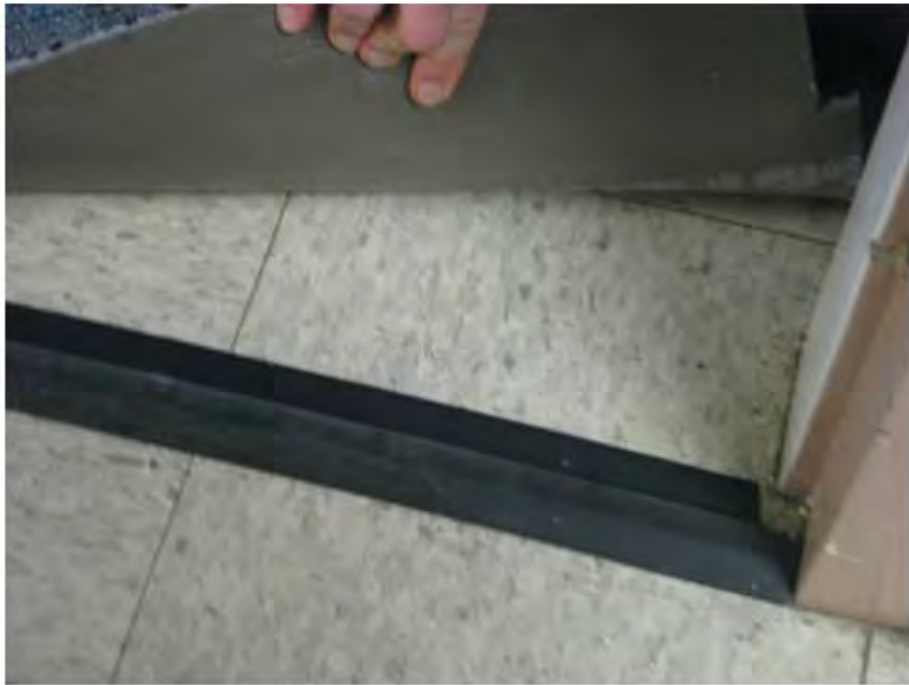
2 nd Layer of Floor Tile and Mastic under 12"x12" Floor Tile and Mastic (5 th Floor Old), Samples 64 and 65
