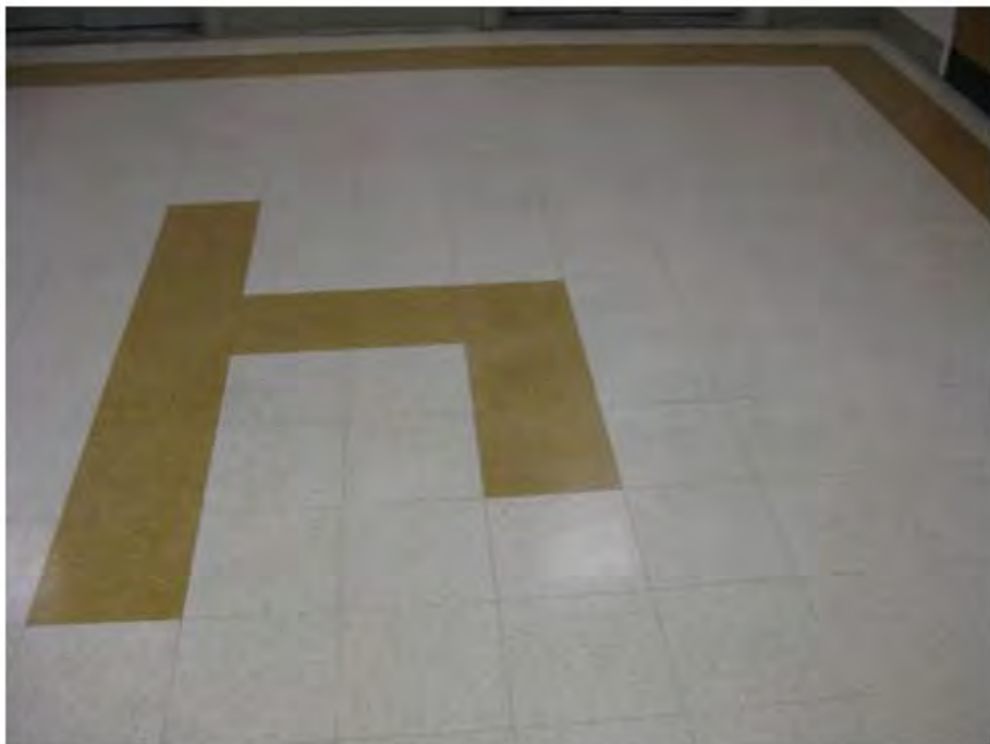
12"x12" Floor Tile and Mastic (4 th Floor Old), Samples 45A and 46A
