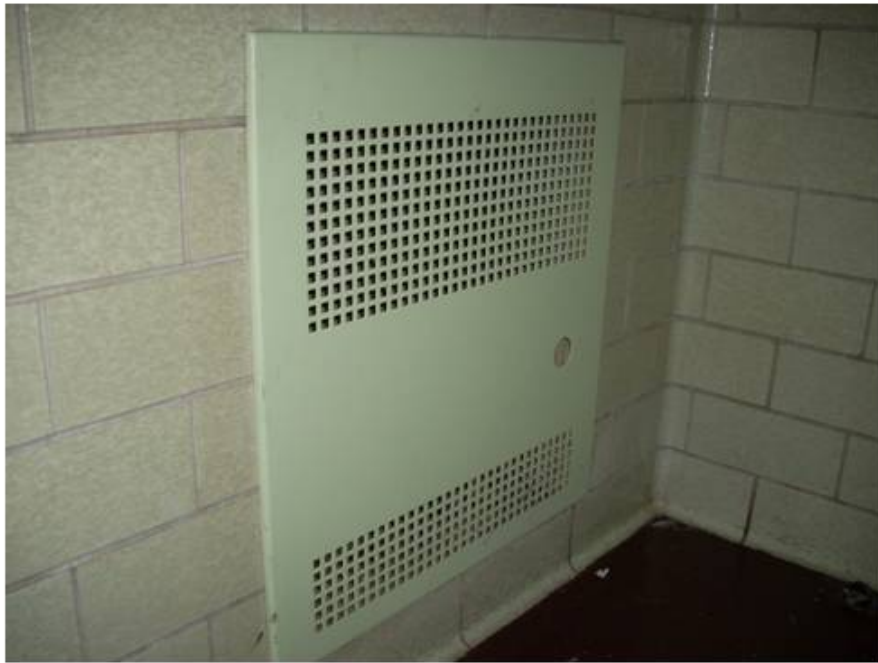
Transite Panel Set into Walls at Radiator
