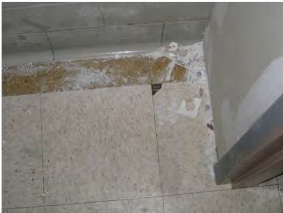
12"x12" Floor Tile and Mastic (6 th Floor Old), Samples 31A and 32A
