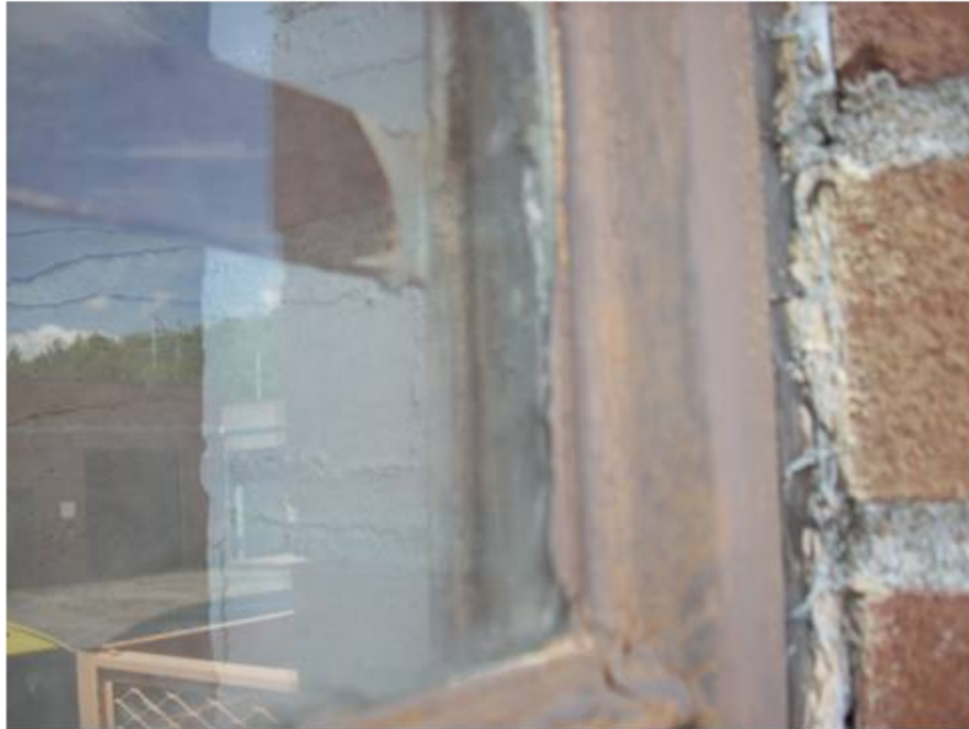
Interior Window Caulk (taken from outside), Sample 14A
