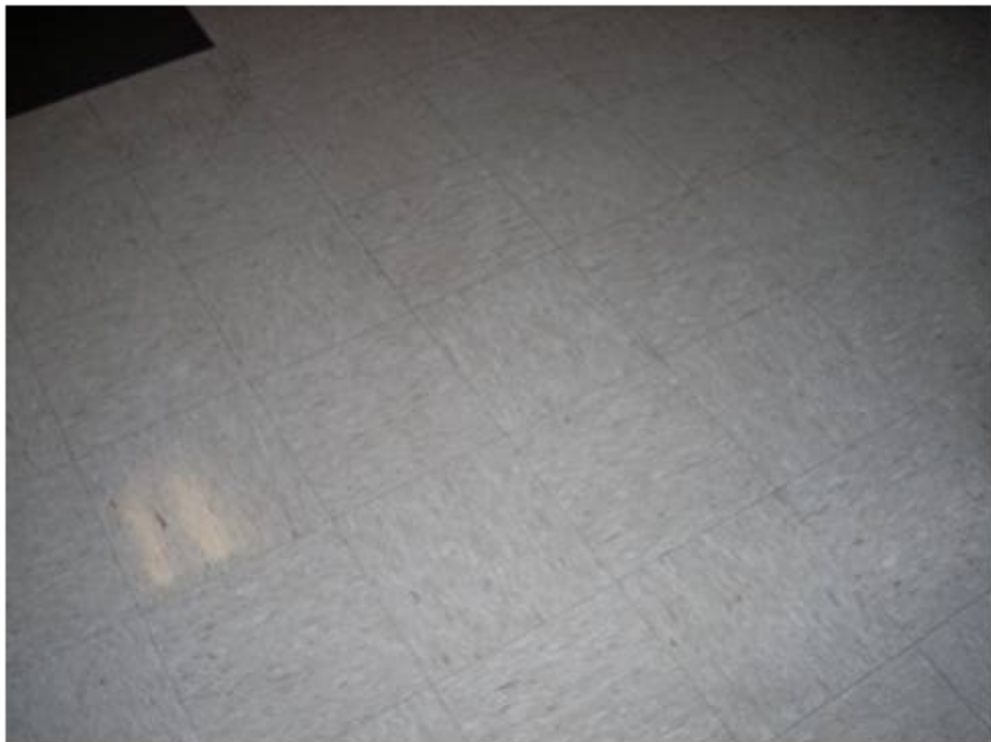
12"x12" Light Brown Floor Tile and Mastic, Samples 17A and 18A
