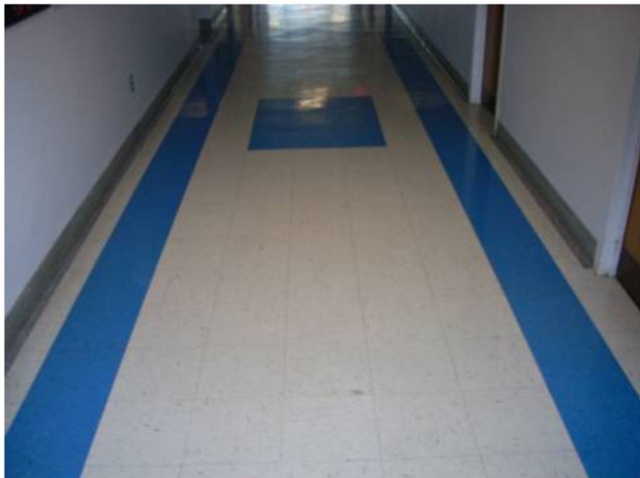
12"x12" Tan Floor Tile and Mastic, Samples 19A, 20A
