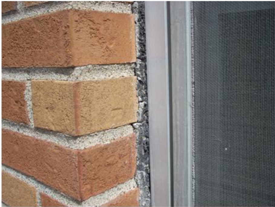
Exterior Window Caulk, Sample 28A
