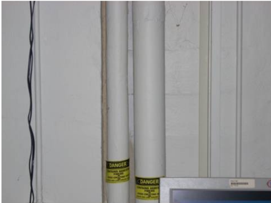
Pipe Insulation, Sample 2C
