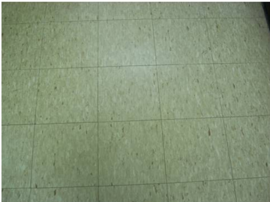
Mastic Associated with 12"x12" Beige Floor Tile, Sample 4A
