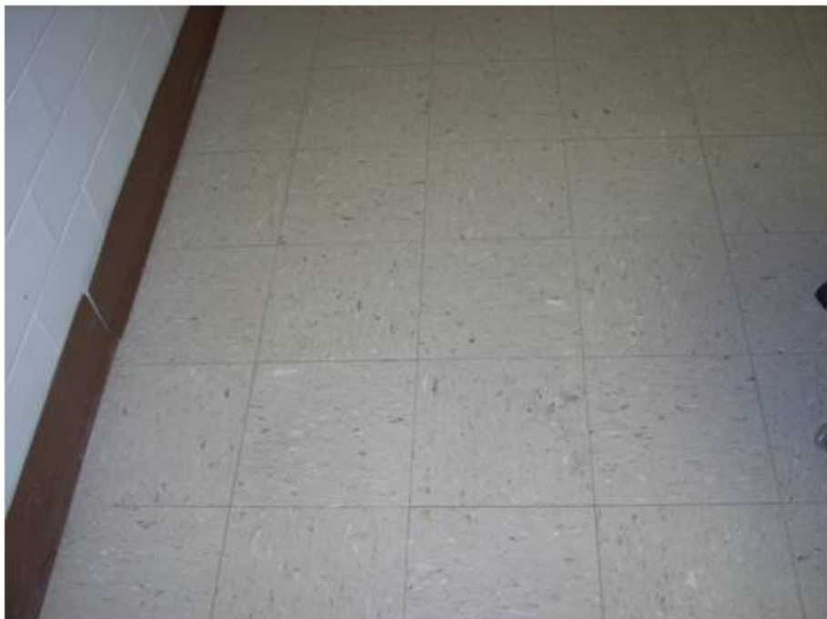
12"x12" Light Brown Floor Tile and Mastic, Samples 29A and 30A
