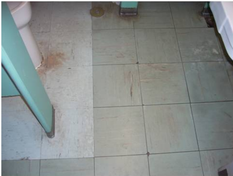
12"x12" Green Floor Tile and Mastic, Samples 25A and 26A
