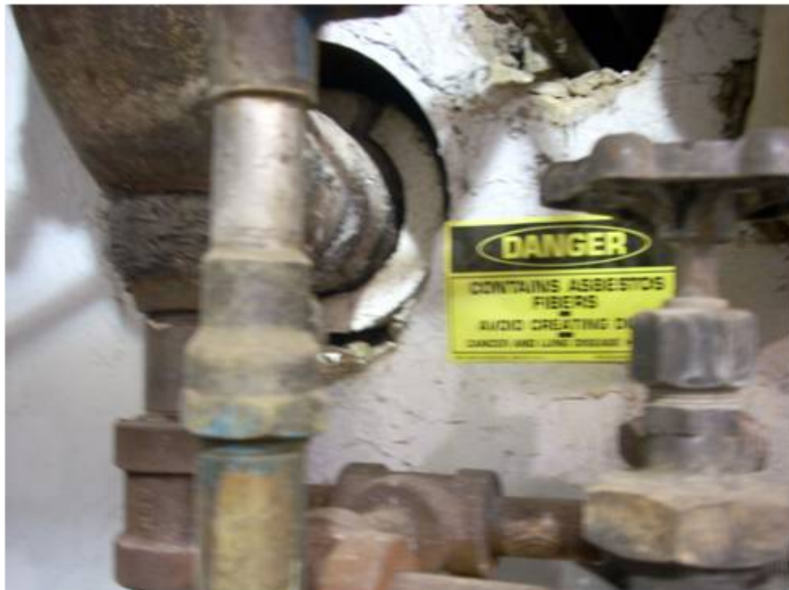
Pipe Insulation Inside Wall Cavity, Sample 20A
