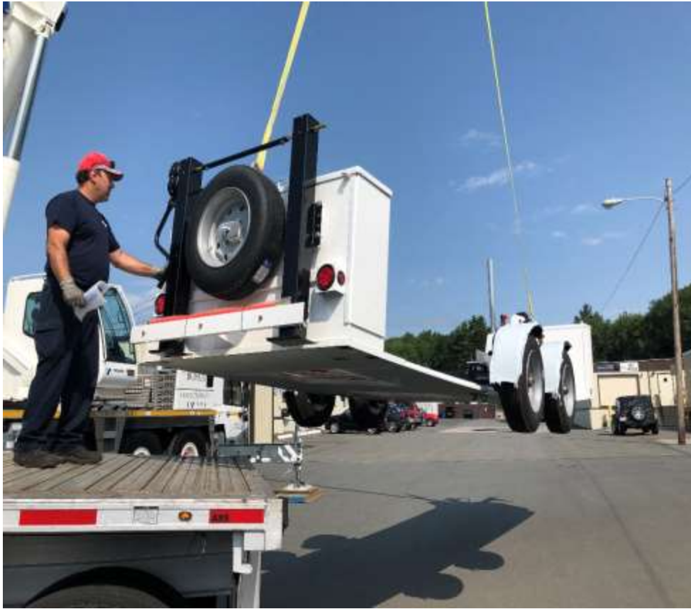
Figure 5. Crane Hoisting & Barrier Unloading
