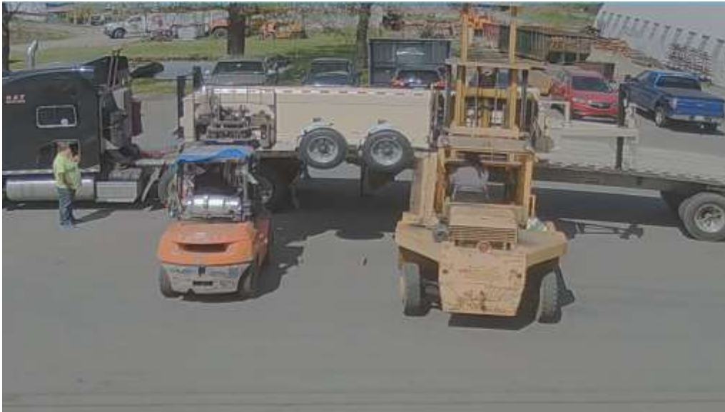
Figure 24. Utilizing Two Forklifts for offloading barrier
