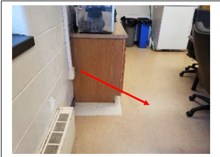
15. ACBM tan 12" floor tile on ACBM black mastic in breakroom 003.
