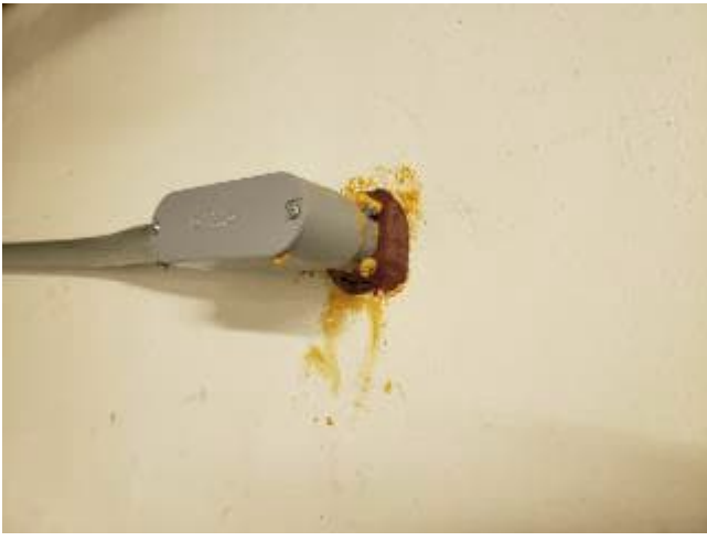
7. Garage Bay G5, red putty around pipe penetration. No asbestos detected.
