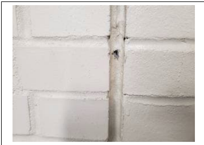
2. Building seam caulking present in the main entry area, no asbestos detected.
