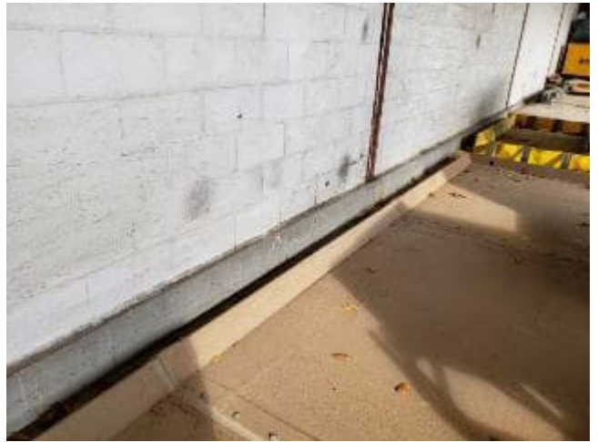
10. Building 28, textured paint and caulking, no asbestos detected.
