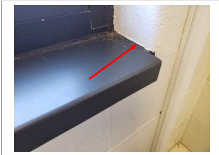
16. Breakroom 003, brown window caulking. No asbestos detected.
