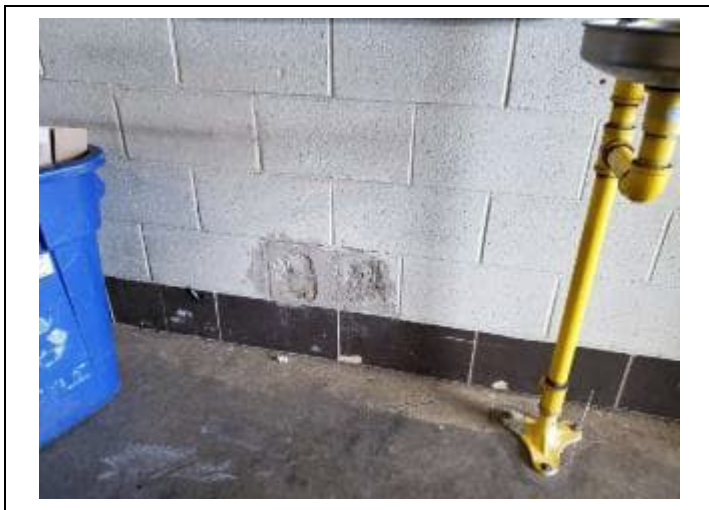
19. Maintenance area 017, white patch caulking along north wall. No asbestos detected.
