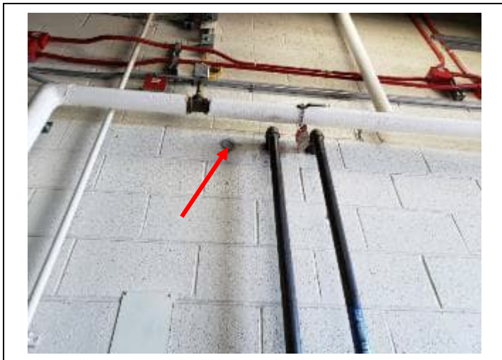
21. Maintenance area 017, grey putty around pipe penetrations. No asbestos detected.
