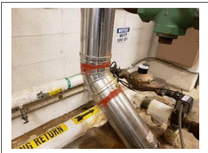
5. Mechanical Room, red caulking on furnace vent pipe. No asbestos detected.
