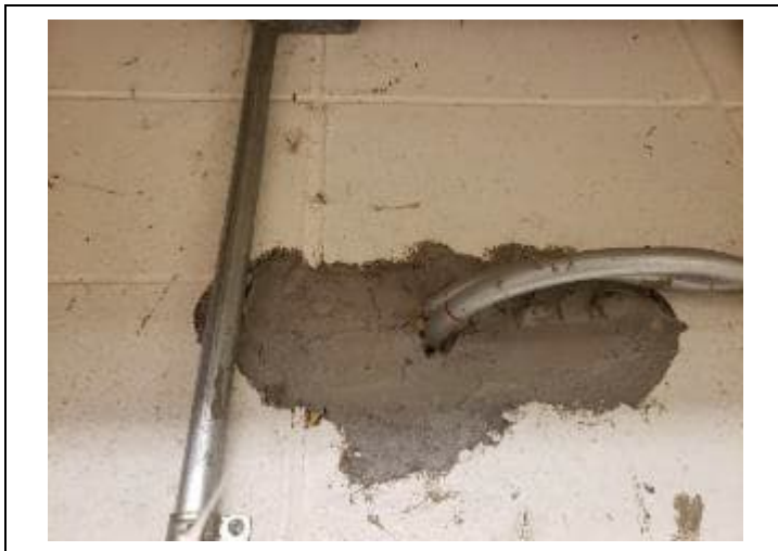
4. Mechanical Room, grey putty around pipe penetration above door. No asbestos detected.
