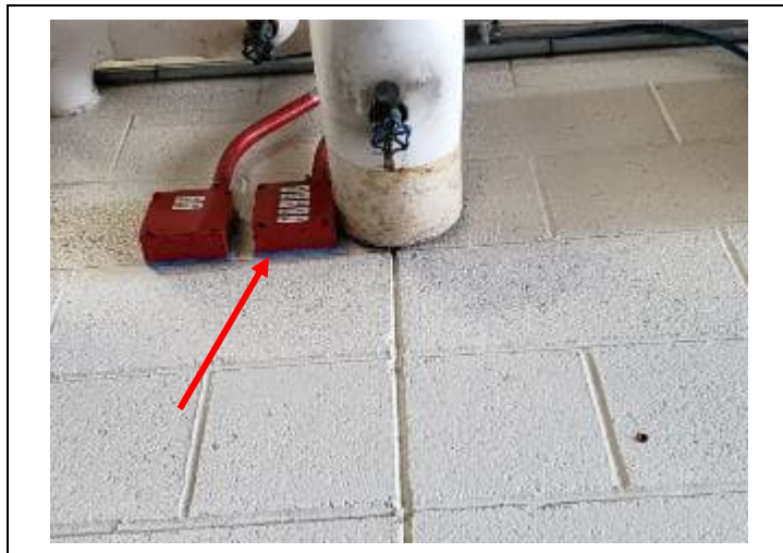
22. Maintenance area 017, blue putty around red electrical boxes. No asbestos detected.
