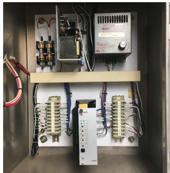
FIGURE 3. CARD AND HOLDER MOUNTING POSITION
