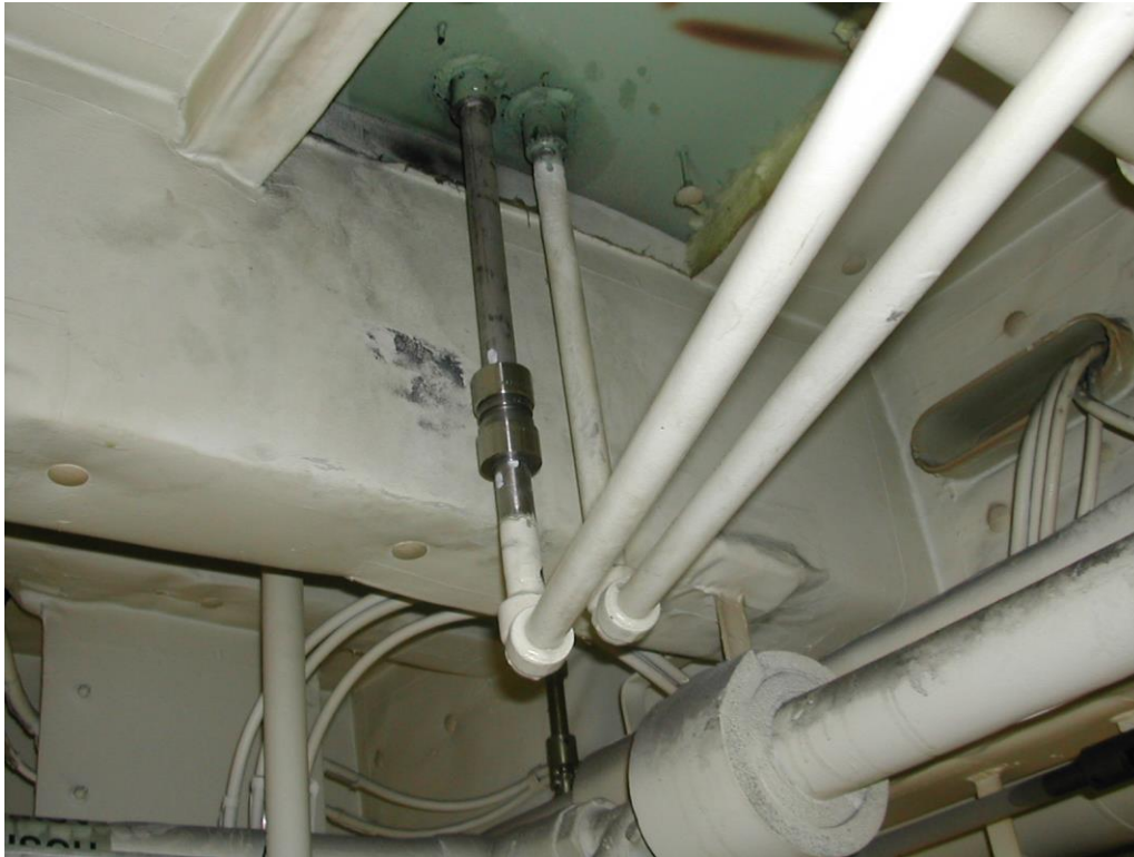
FIGURE, Photograph of Typical LOKRING Union Fitting (used in similar application)
