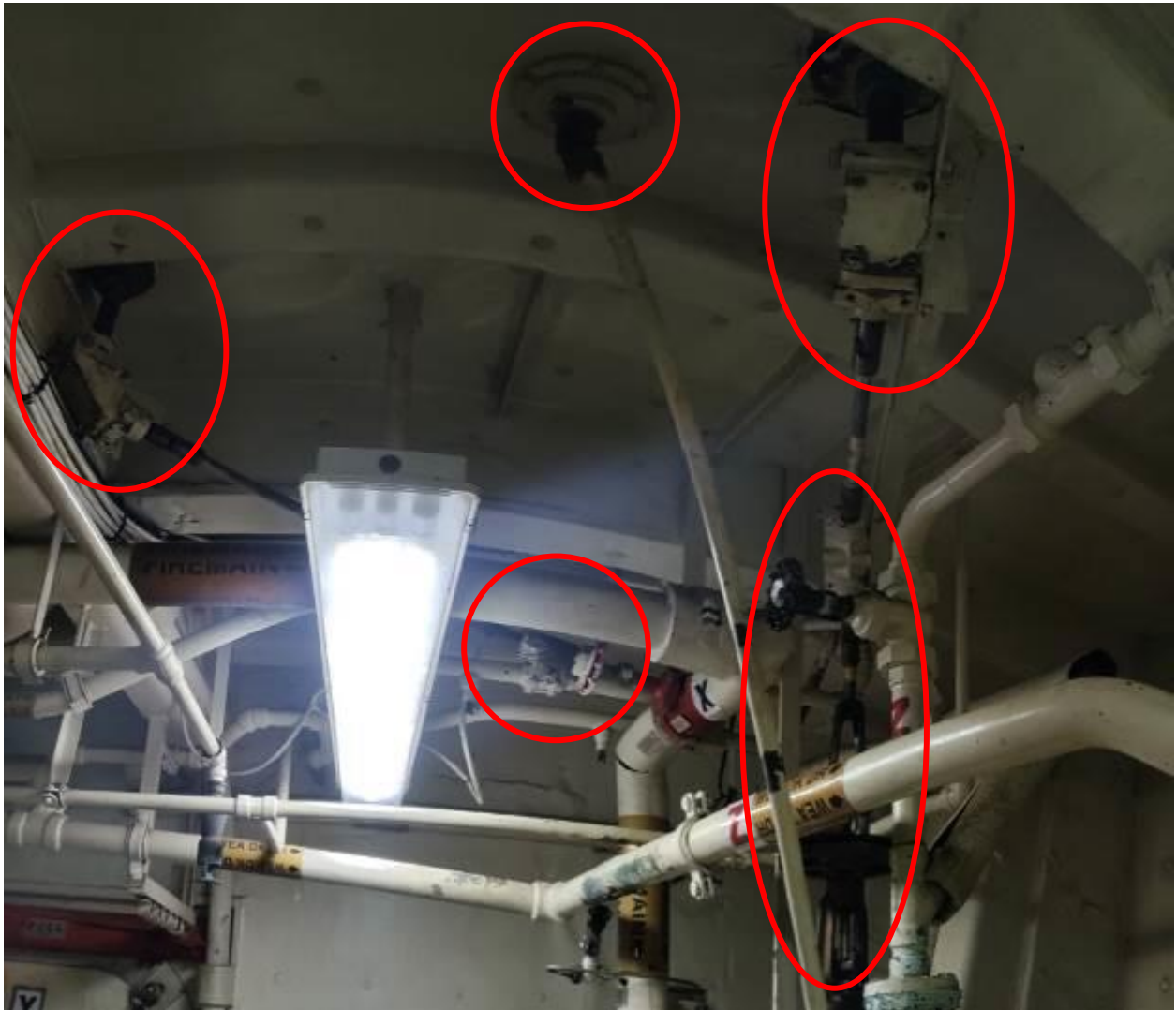
FIGURE 3 – EXAMPLE OF REMOTE VALVE OPERATORS UNDERNEATH BOUY DECK
