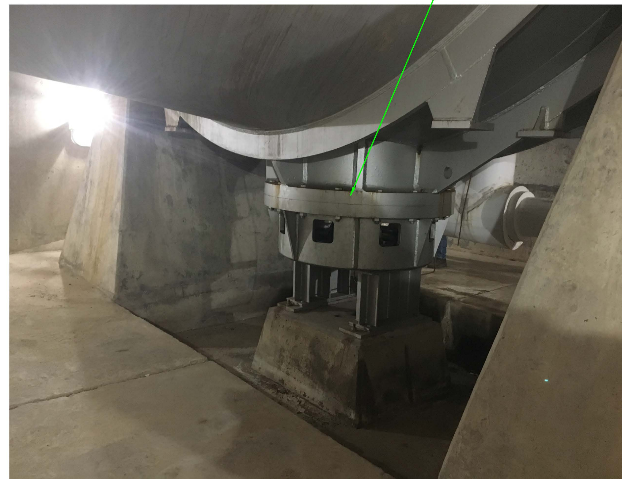
" PICTURE 1 - UNIT 4 BUTTERFLY VALVE LOWER TRUNNION BEARING HOUSING " UPSTREAM VIEW
