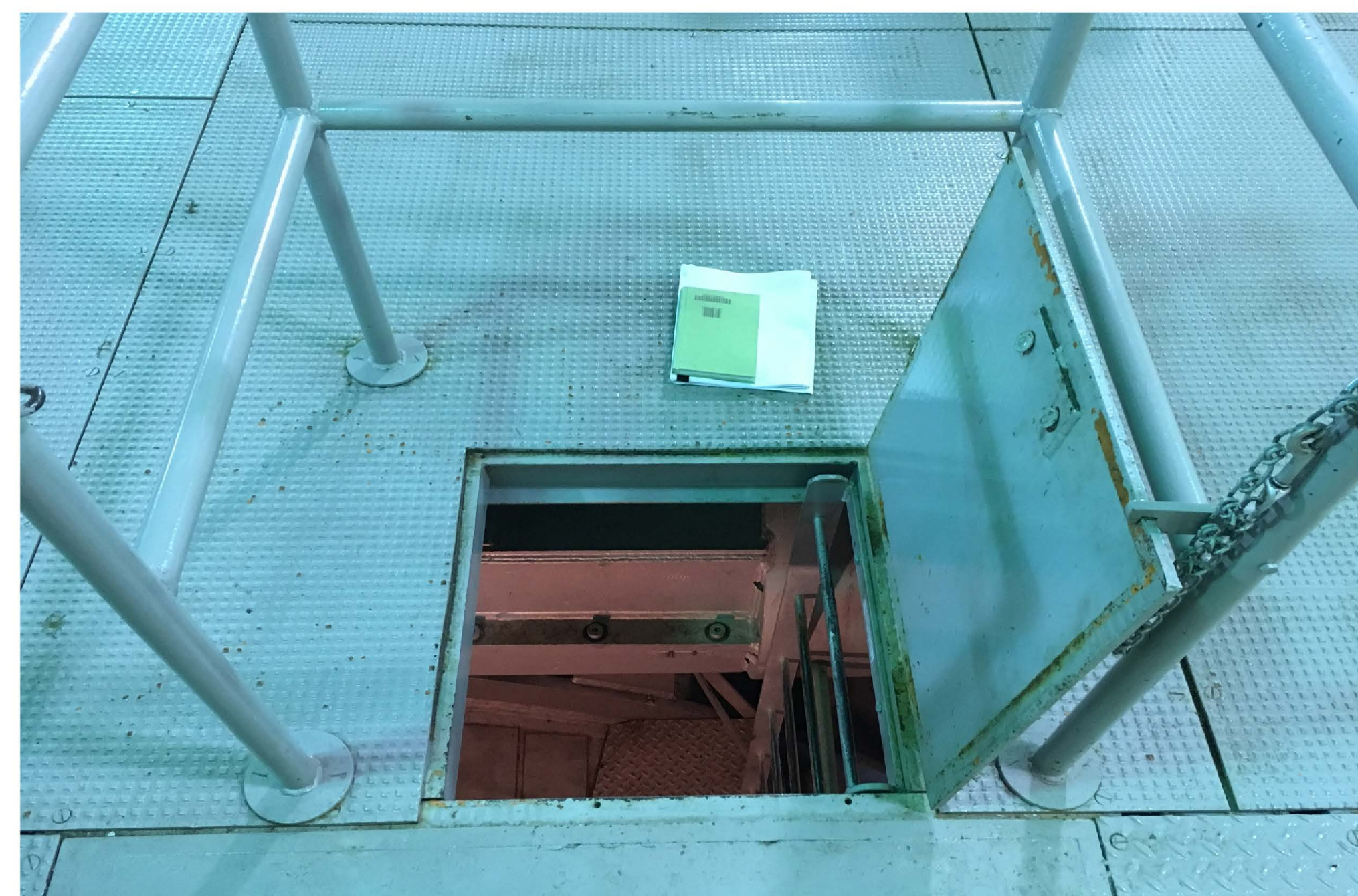
" PICTURE 4 - UNIT 4 BFV MAINTENANCE ACCESS HATCH "
