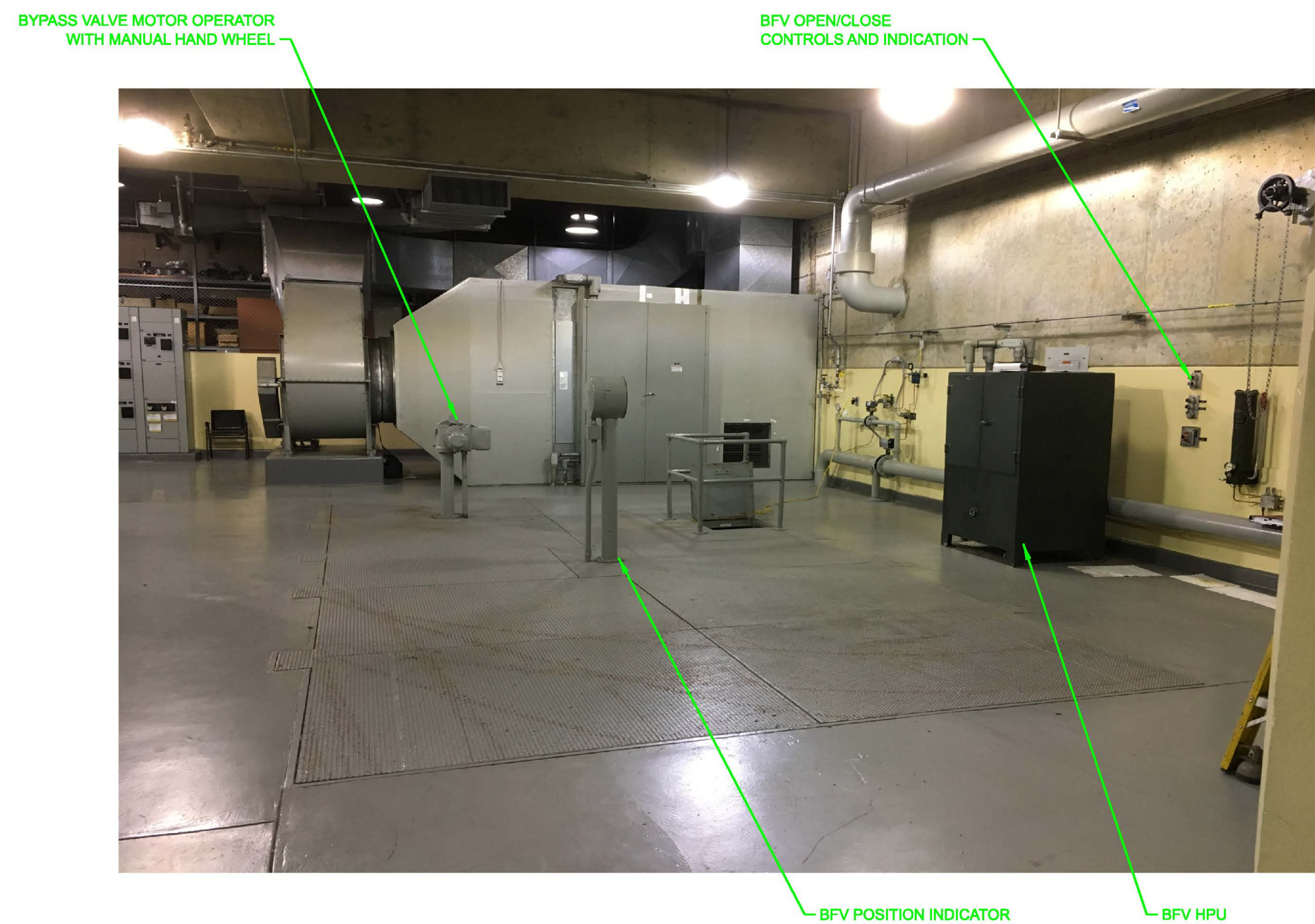
" PICTURE 1 - UNIT 5 PENSTOCK BUTTERFLY VALVE CORRIDOR (EL 2052.00) "
