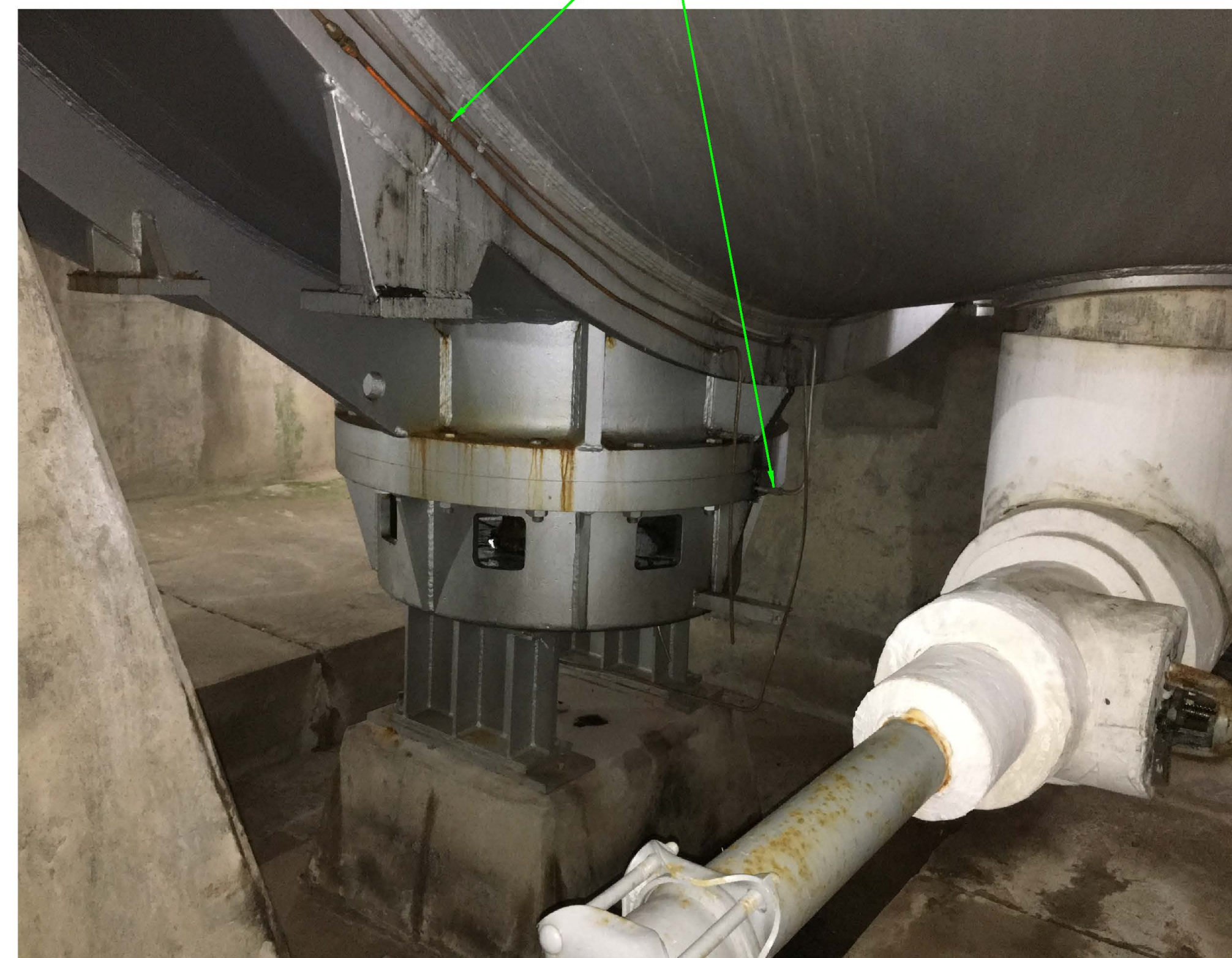
" PICTURE 2 - UNIT 4 BUTTERFLY VALVE LOWER TRUNNION BEARING HOUSING DOWNSTREAM VIEW
