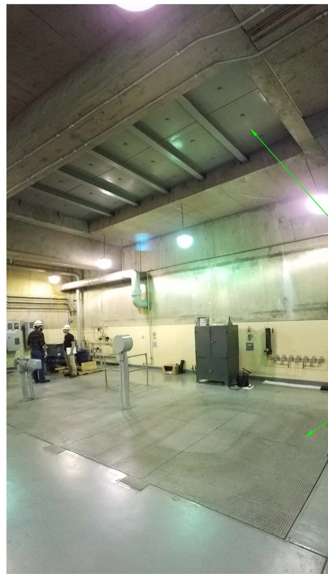
" PICTURE 5 - UNIT 4 BFV HATCHES AT EL 2052 AND 2070 "
