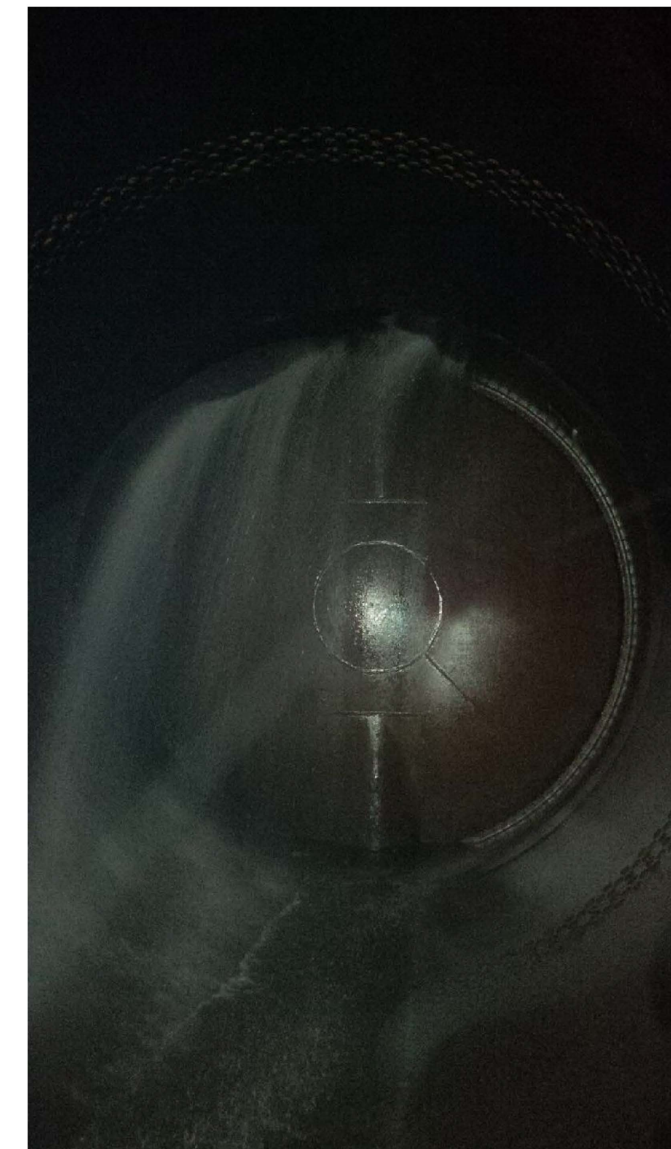
" PICTURE 6 - UNIT 4 BUTTERFLY VALVE CLOSED POSITION EXISTING VALVE LEAKAGE "
