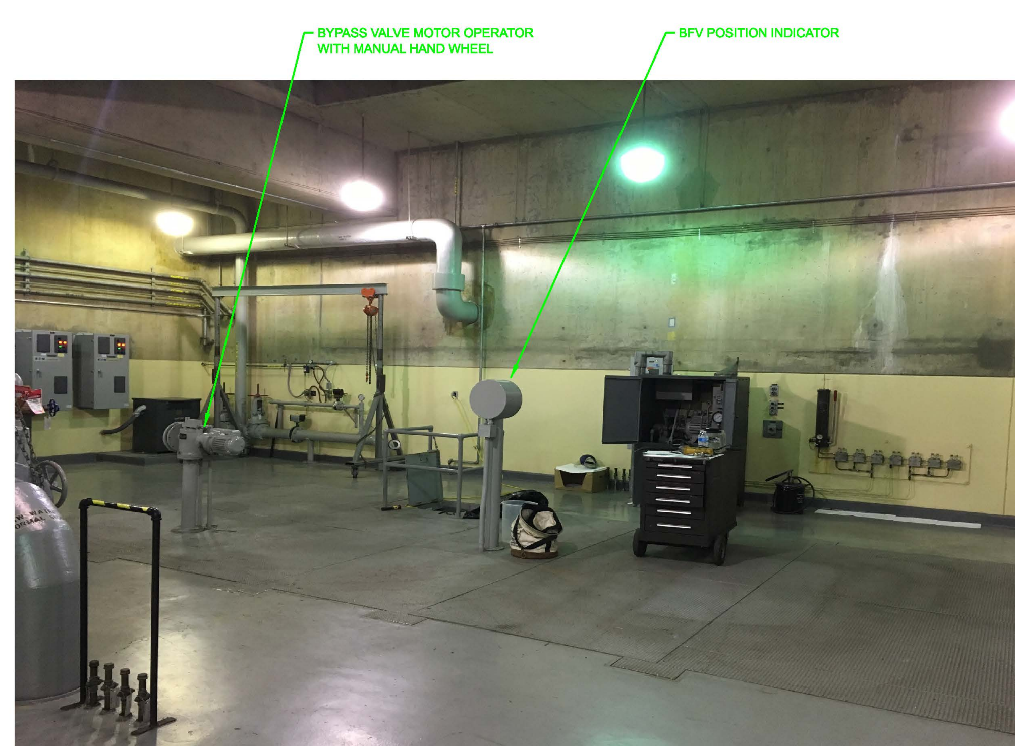
" PICTURE 2 - UNIT 4 BUTTERFLY VALVE CORRIDOR (EL 2052.00) "
