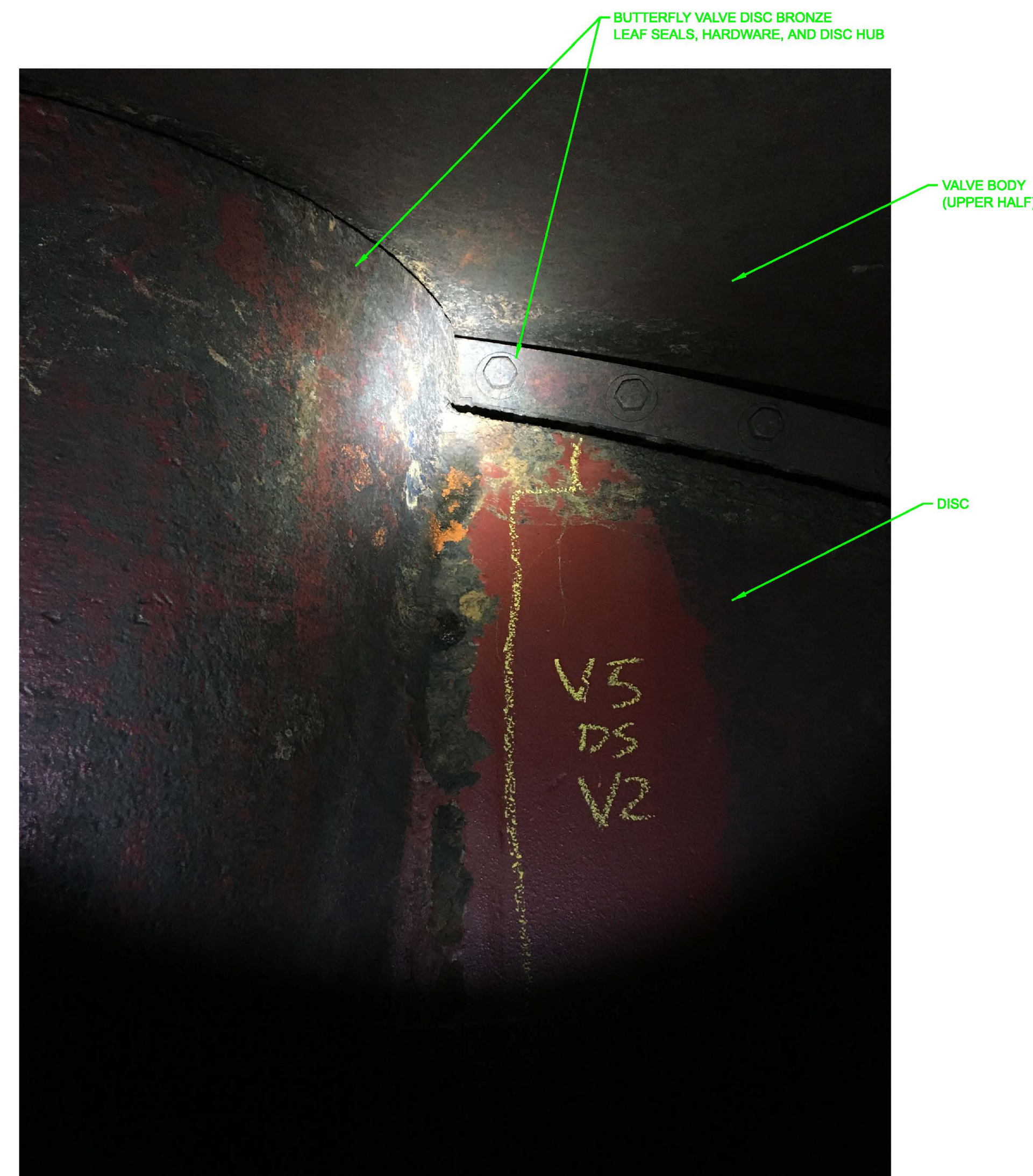
" PICTURE 5 - UNIT 4 BUTTERFLY VALVE DISC "
