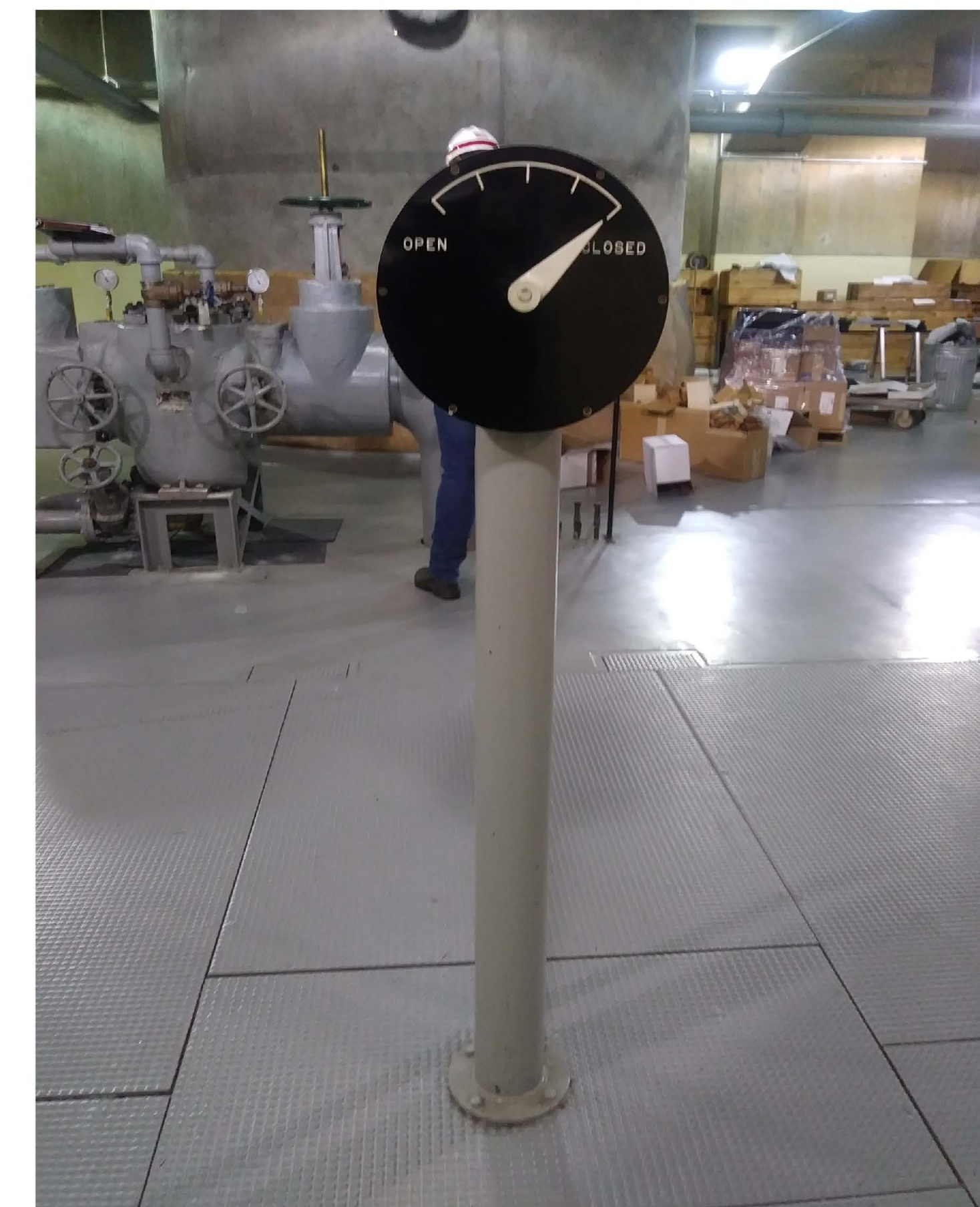
" PICTURE 3 - UNIT 5 BFV POSITION INDICATOR "
