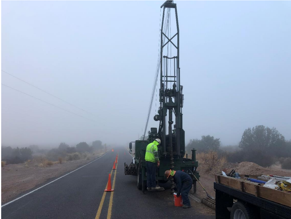
Photo 84: BH21-05, Hollow Stem Auger Drilling
