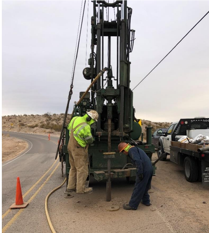
Photo 45: BH21-03, Down Hole Hammer (ODEX) Drilling
