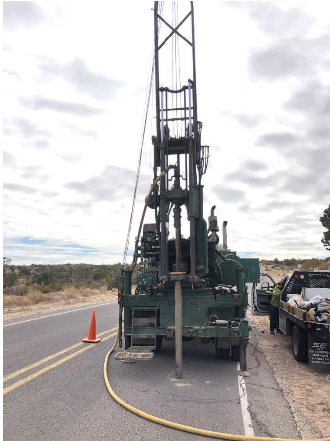
Photo 35: BH21-02, SPT-07 Drilling Set Up
