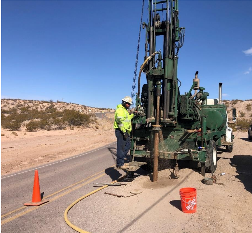
Photo 68: BH21-04, Down Hole Hammer (ODEX) Drilling
