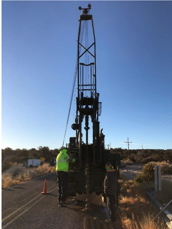
Photo 24: BH21-01, Hollow Stem Auger Drilling
