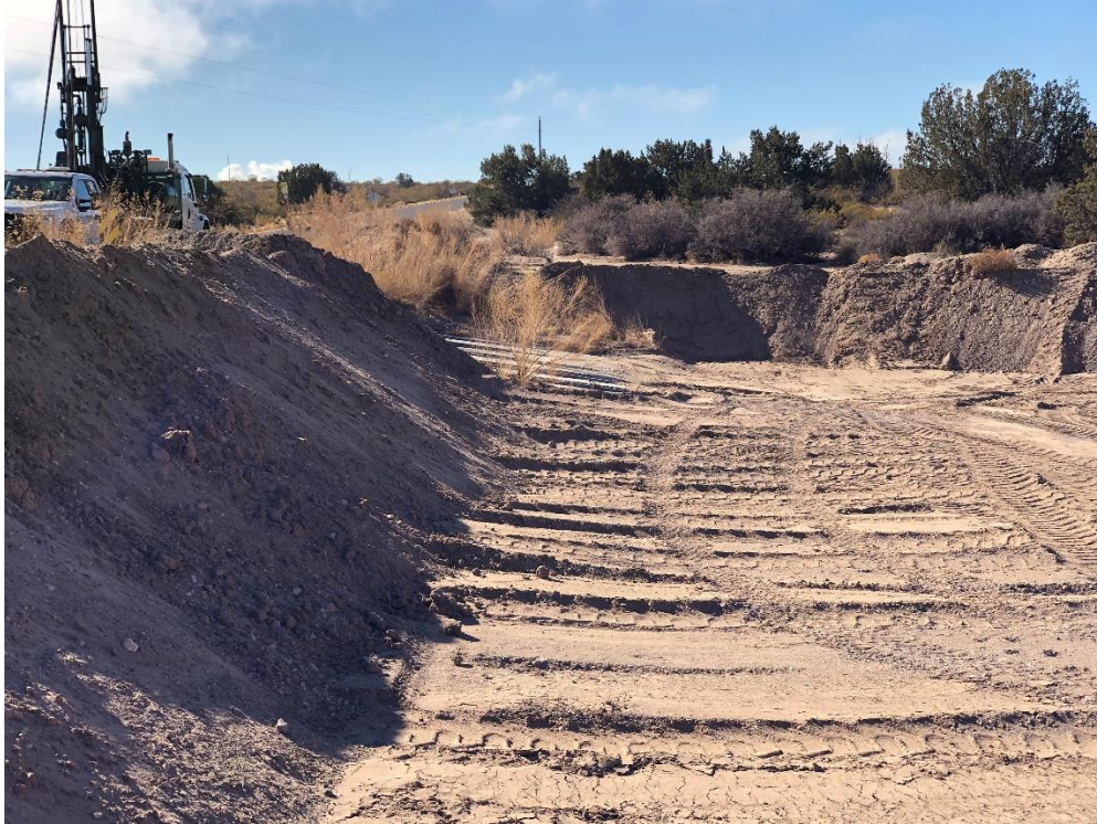
Photo 18: Significant Plowing of Eroded Material
