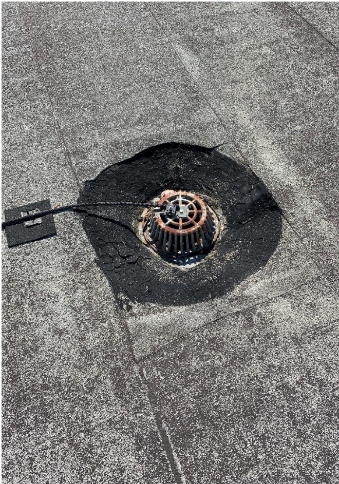
Figure 6: Roof Drain (typical)
