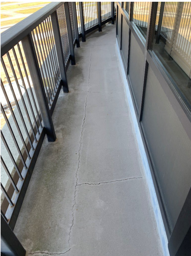
Figure 10: Catwalk Pics (Typical) Cracking in material in some places.
