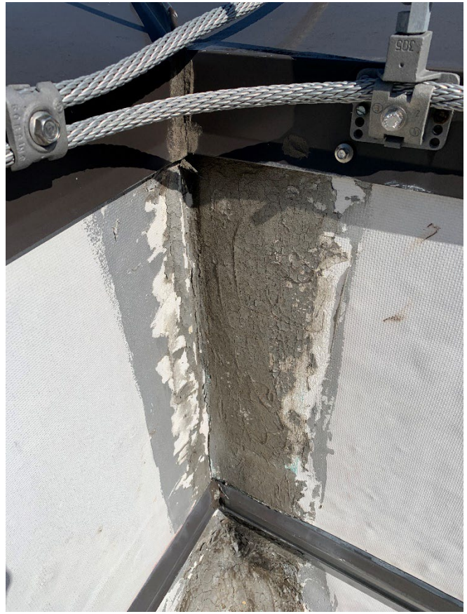
Figure 5: Typical Treatment at upper parapet wall corner
