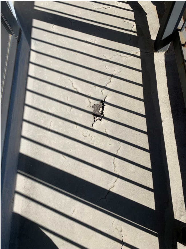
Figure 11: Area where epoxy coating severely cracked. Cutout/Treat. Reseal
