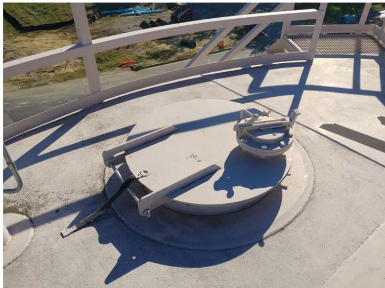
E.66 Roof Nozzle B, 36" Manhole with 8" Manual Gauge Hatch(Not Bolted)
