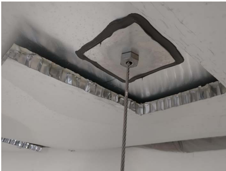
E.83 Anti-Rotational Device
