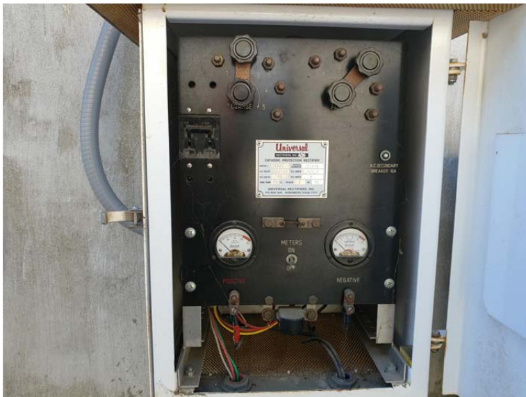
E.51 Cathodic Protection Rectifier
