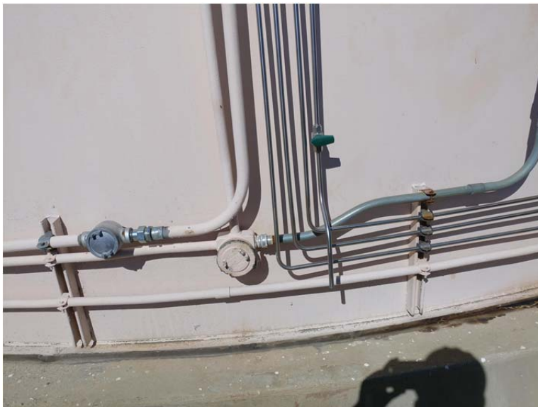
E.26 Junction Box not Properly Sealed
