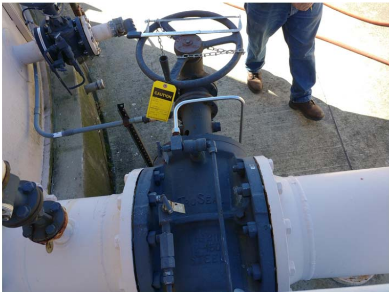
E.42 Coating Failure on 12" Issue
