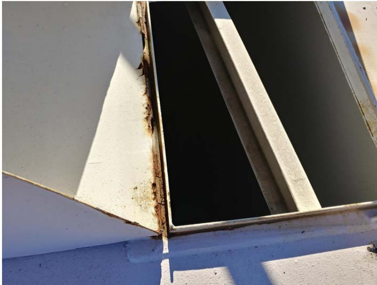
E.58 Coating Failure/Corrosion on Hood
