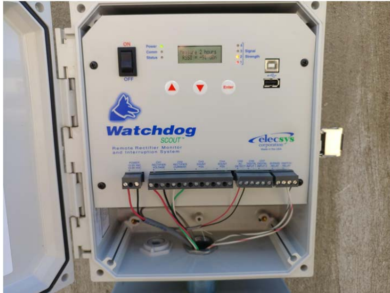
E.52 Cathodic Protection Rectifier Monitor
