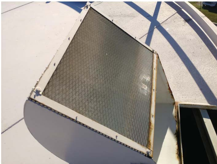
E.59 Inspection Hatch Screen
