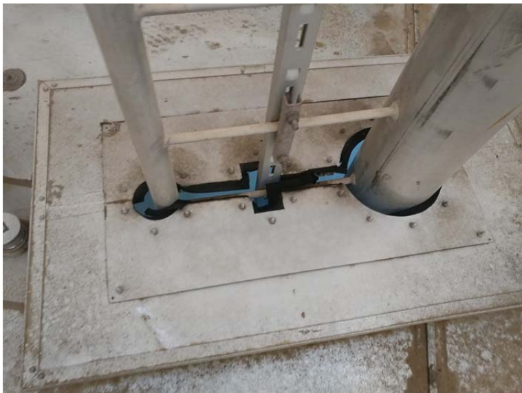
E.96 IFR Ladder Penetration Deteriorated
