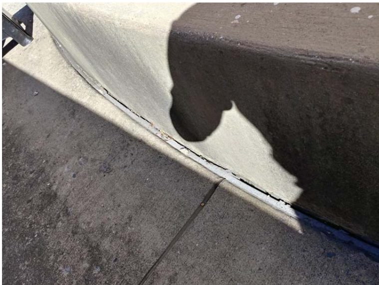
E.15 Failed Ringwall Joint Sealant
