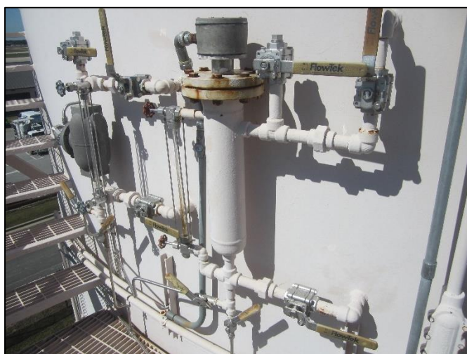
B.11: High Level Alarms and Controls
