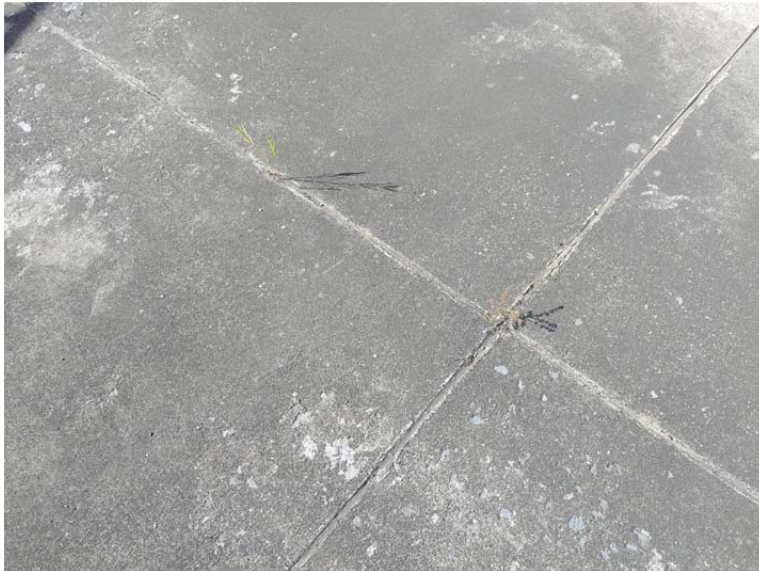
E.8 Vegetation in Secondary Containment Floor
