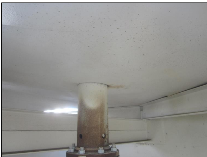
B.17: ATG/Water Bottom Sensor and Well
