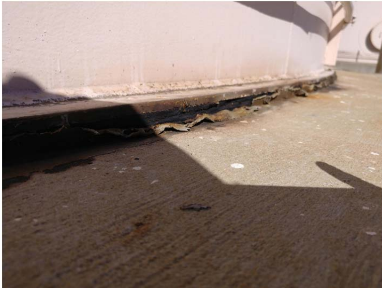
E.16 Ringwall Seal Failure
