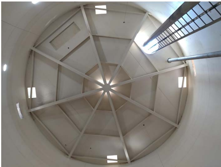
E.95 IFR Roof Rafter Layout
