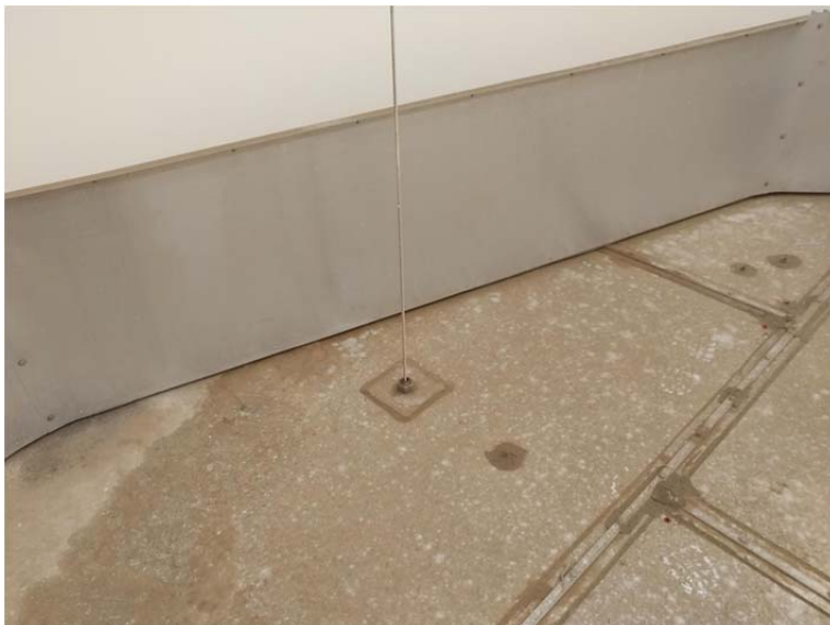
E.99 Anti-Rotation Device (ARD)
