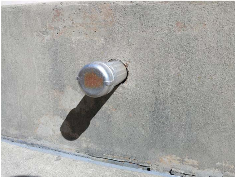
E.5 Leak Detection(Not Sealed)
