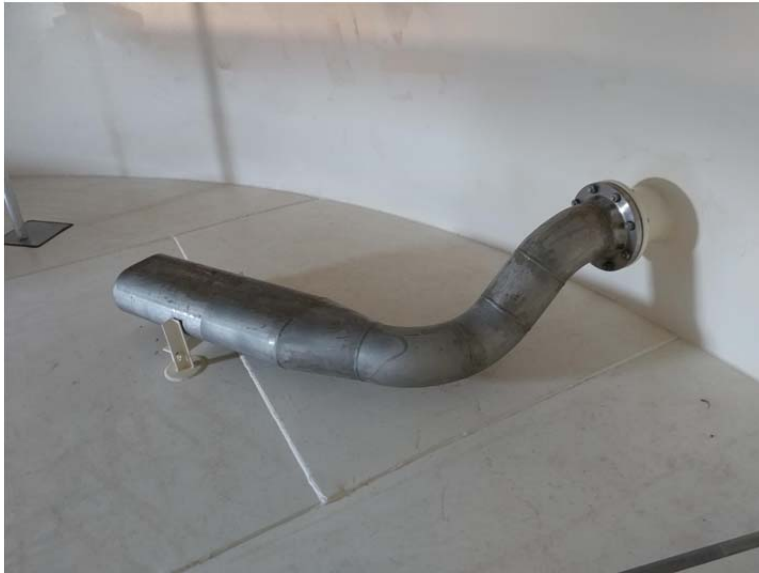
E.91 Carbon Steel Connected to Stainless Steel Flange
