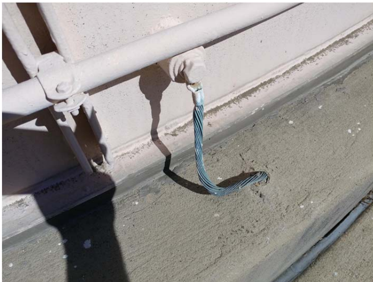
E.17 Unsealed Grounding Cable
