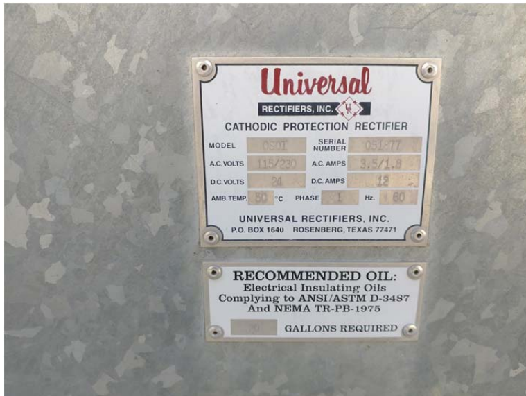
E.50 Cathodic Protection Rectifier
