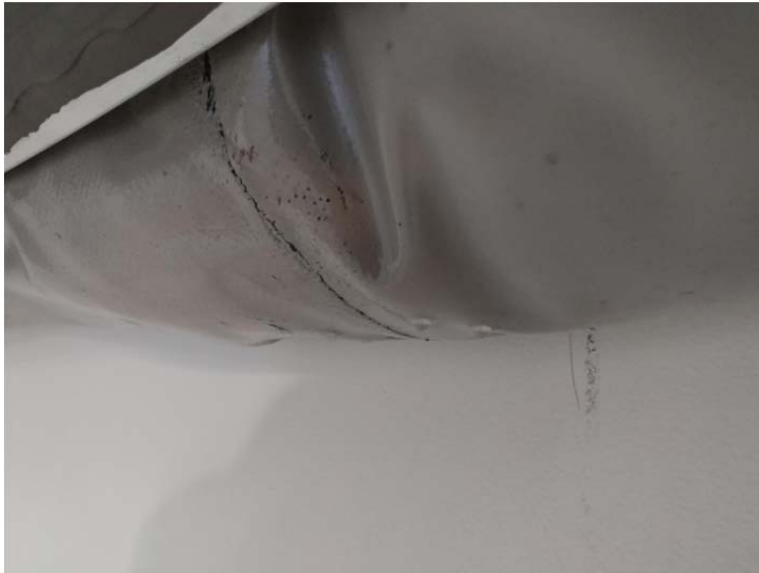
E.79 Foam Seal Saturated and Dripping Fuel
