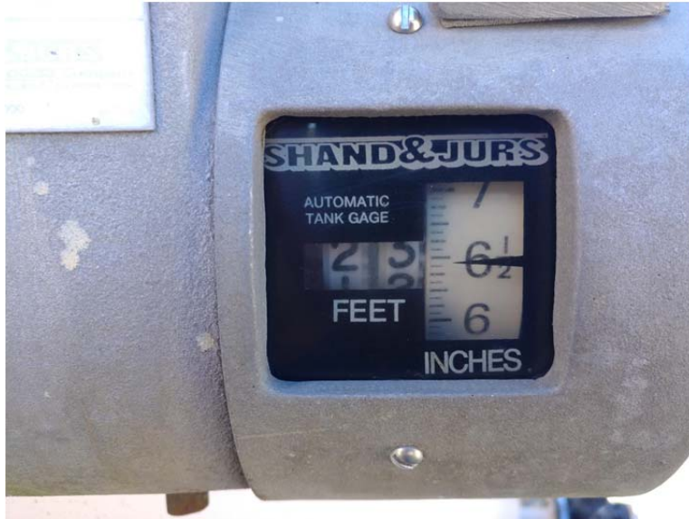
E.40 Mechanical Tape Gauge
