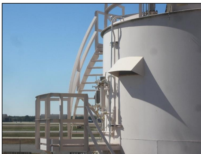
B.12: Shell Overflow, Stairway Landing, and Alarms
