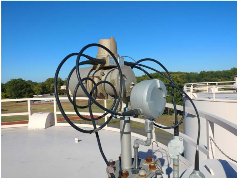
E.62 Roof Nozzle A, 6" Enraf/Vito Stilling Well
