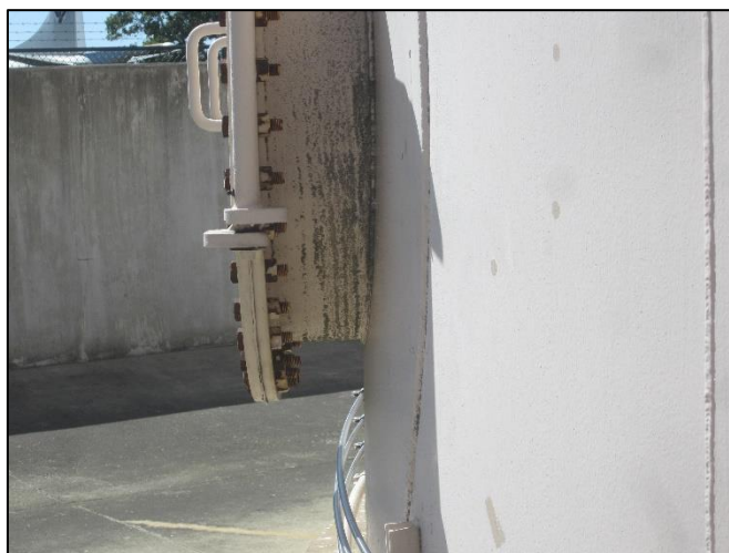
B.10: Mold/Mildew Under Manhole Neck
