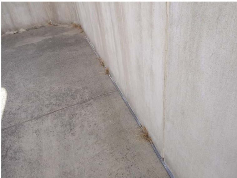
E.9 Vegetation in Secondary Containment
