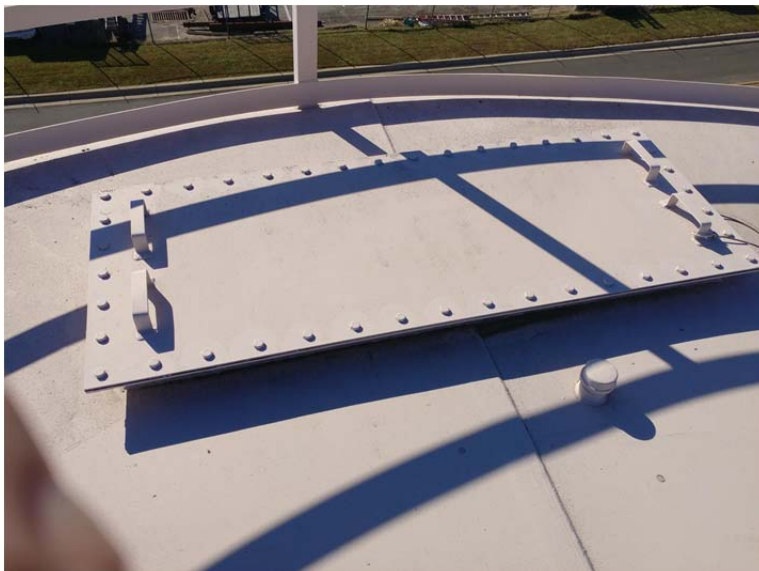
E.72 Roof Nozzle F, 30" x 72" Pan Installation Hatch, Nozzle G, 2 1/2" Cap
