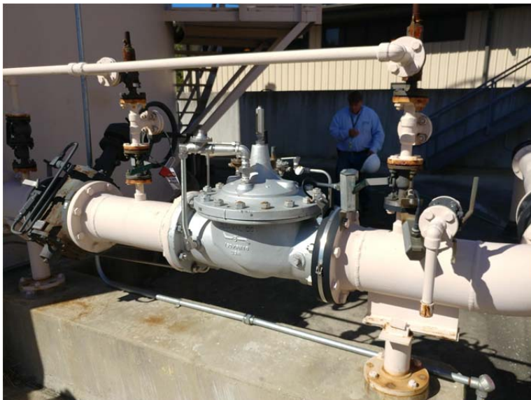
E.33 Coating Failure on 8" Receipt
