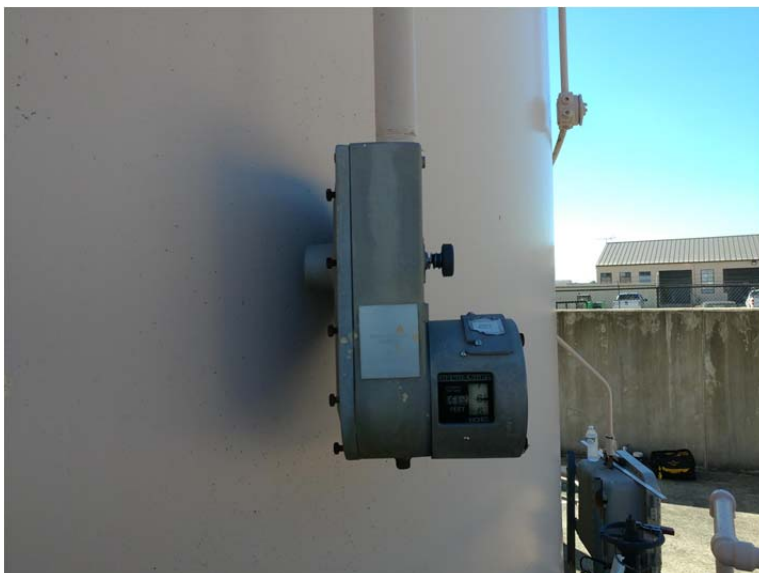
E.39 Mechanical Tape Gauge
