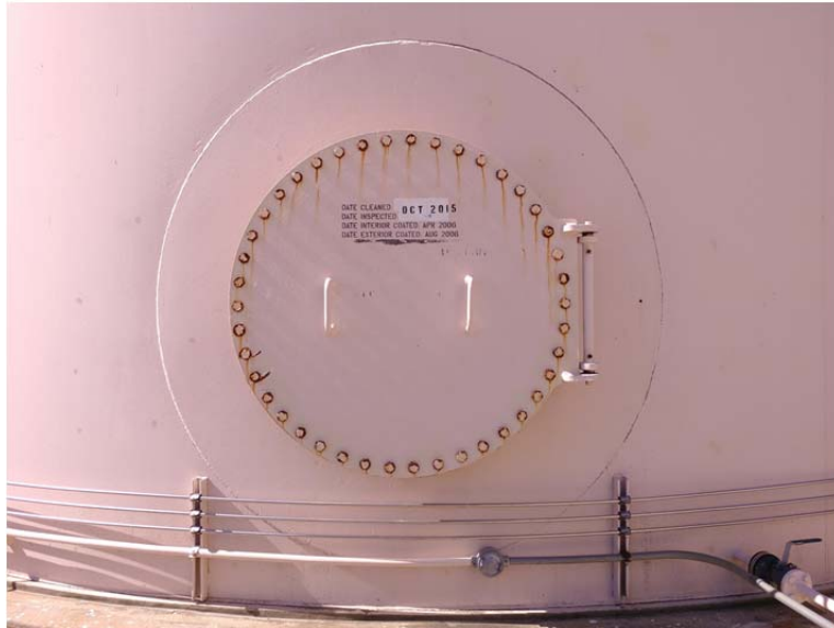
E.28 Nozzle H, 36" Manhole with 74" Repad
