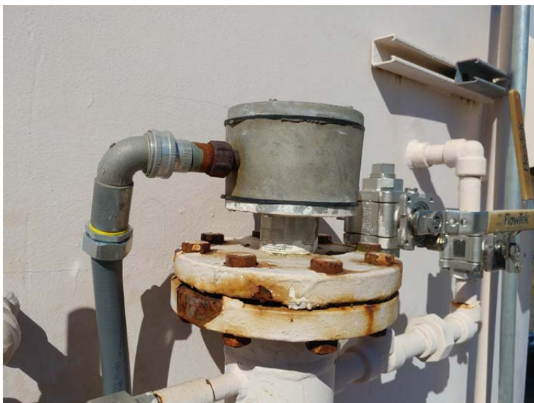
E.24 Coating Failure on Low and High Level Alarms
