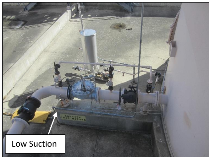
B.5: Receipt Piping Over Swale and Near Drain
