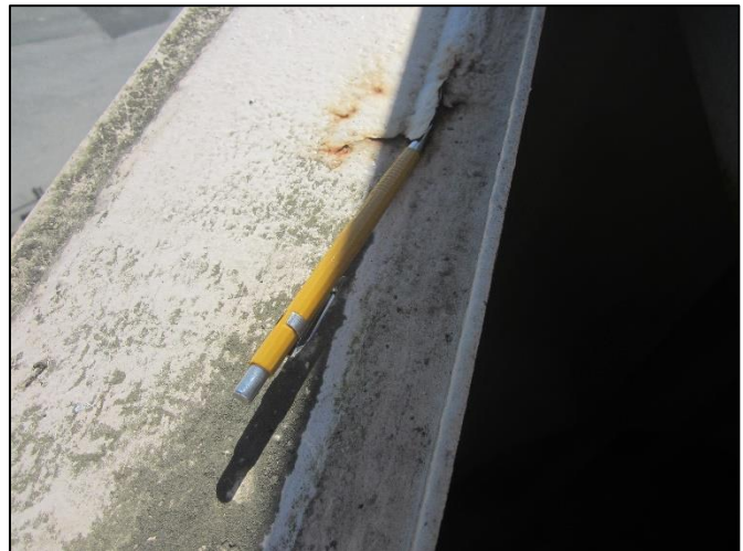
B.16: Coating Failure on Roof at Roof Perimeter Vent
