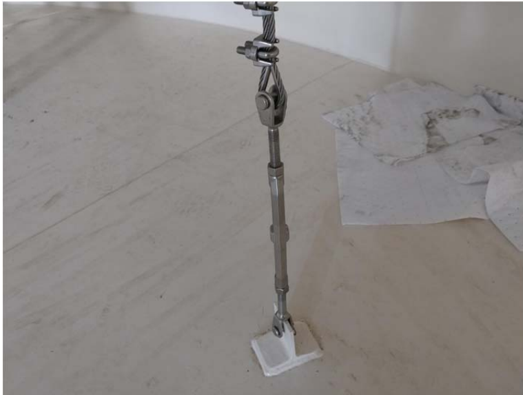
E.82 Anti-Rotational Device
