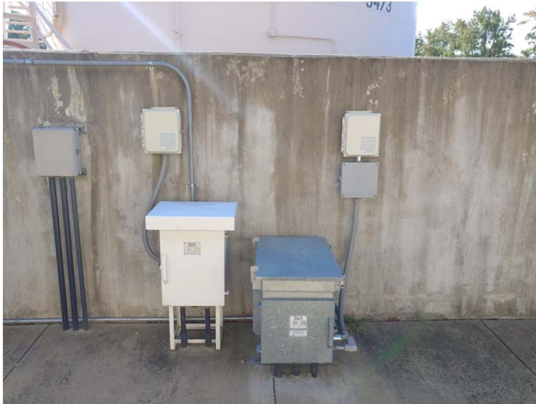
E.49 Cathodic Protection
