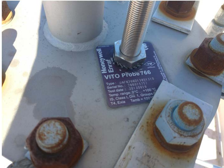
E.64 Roof Nozzle A, 6" Enraf/Vito Stilling Well
