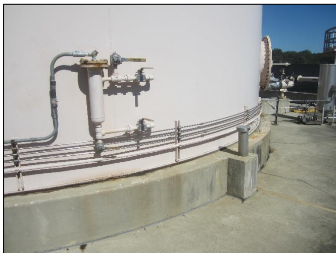
B.7: Low Level Alarm and Leak Detection Well
