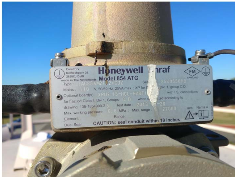
E.65 Roof Nozzle A, 6" Enraf/Vito Stilling Well
