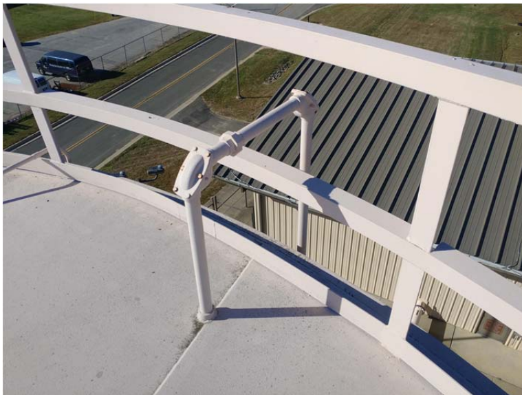
E.74 Roof Nozzle J, 1 1/2" Mechanical Tape Gauge
