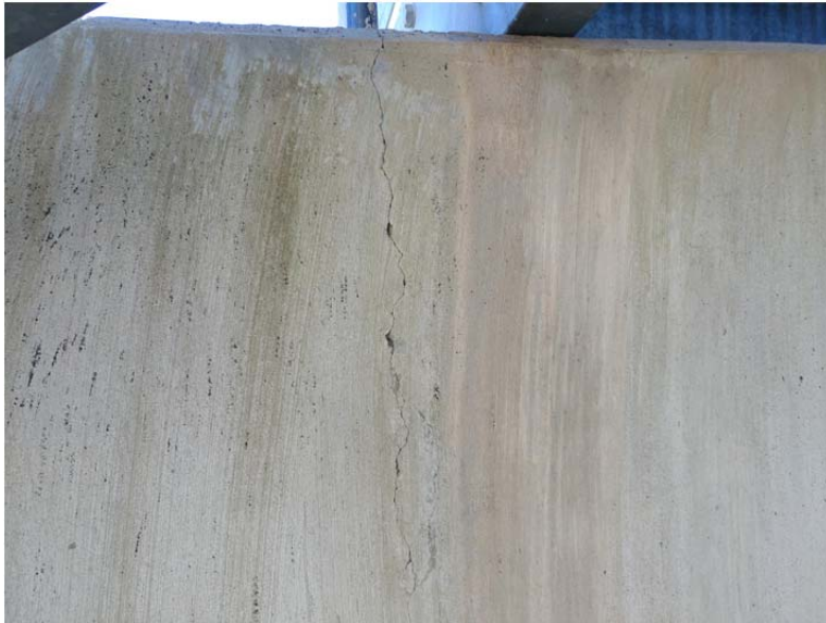
E.10 Crack in Secondary Containment Wall
