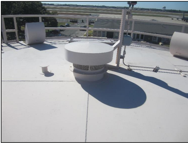
B.13: Roof Center Vent and Scaffold Cable Support
