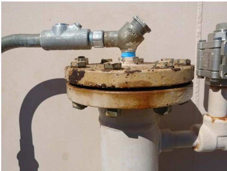
E.27 Coating Failure on Low Level Alarm
