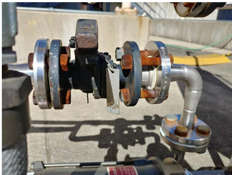
E.30 Water Draw-Off Piping Galvanic Corrosion
