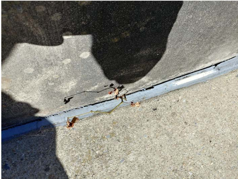
E.13 Failed Joint Sealant in Secondary Containment Floor
