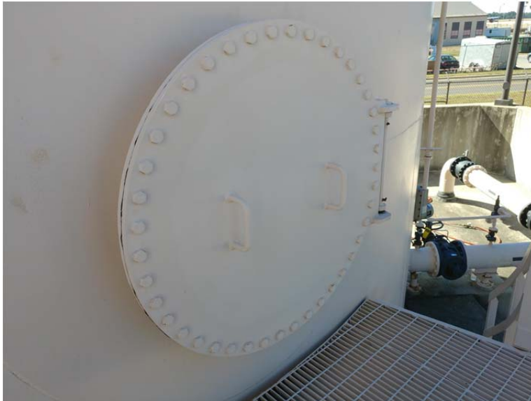
E.37 Nozzle K, 36" Internal Floating Roof Manhole
