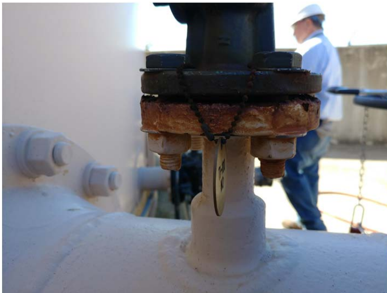
E.44 Coating Failure on Low Suction Flange
