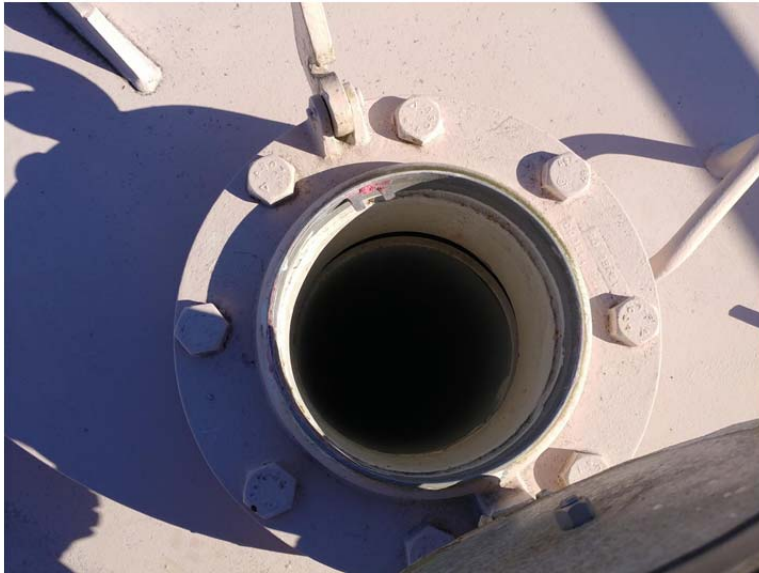
E.67 8" Manual Gauge Hatch
