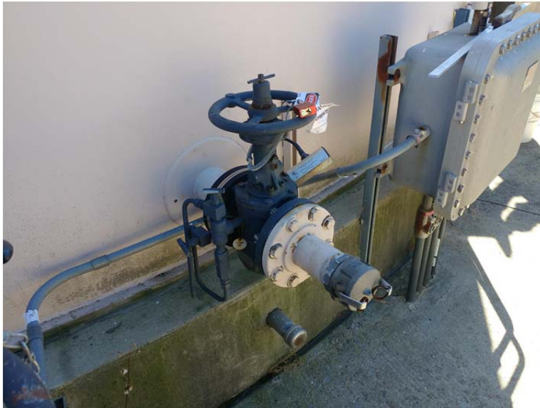
E.43 Nozzle M, 4" Low Suction with 12" Repad
