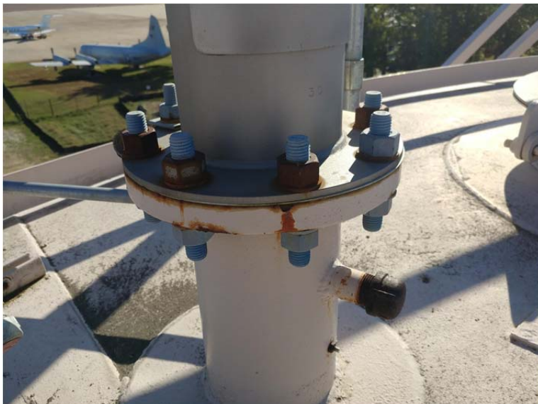
E.63 Roof Nozzle A, 6" Enraf/Vito Stilling Well
