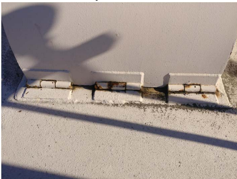
E.60 Coating Failure on Hood Hinge
