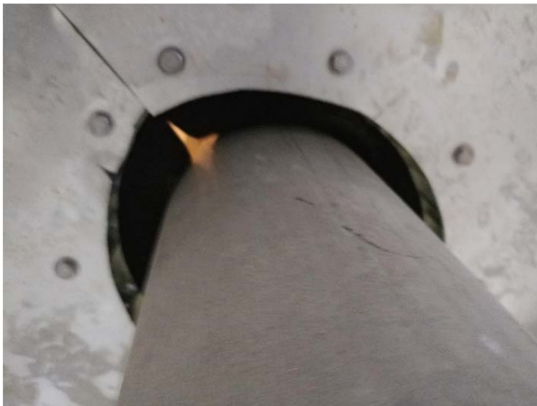
E.80 Penetration Seal Deteriorated
