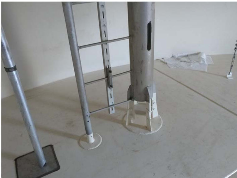
E.78 Bottom Nozzle B, 8" Manual Gauge with Ladder
