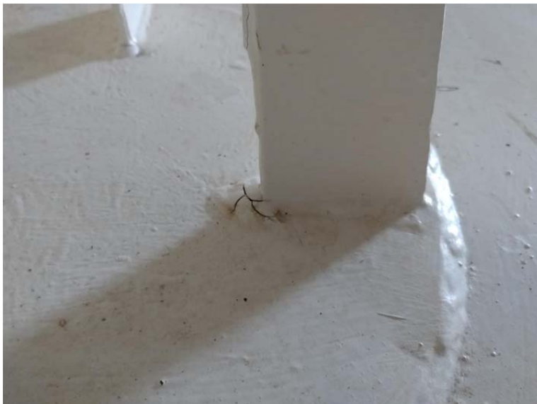
E.81 Minor Coating Failure on Manual Gauge Well Reinforcement Pad
