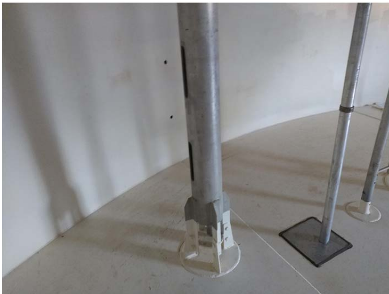
E.77 Bottom Nozzle A, 6" Enraf/Vito Stilling Well
