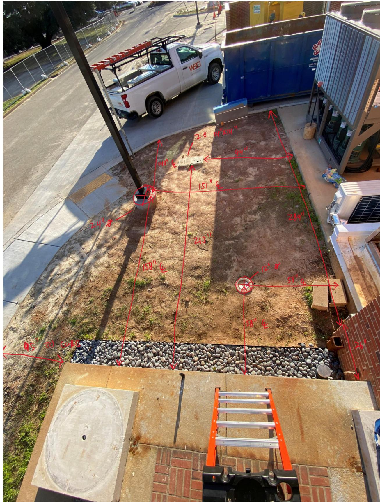
**NOTE: THE FIRE PUMP PACKAGE FOOTPRINT IS FIXED AT 11' (WIDE) X 16' (LONG), NO DEVIATIONS ALLOWED.**
