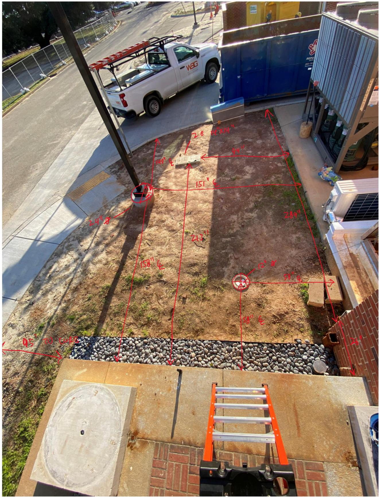
NOTE: THE FIRE PUMP PACKAGE FOOTPRINT IS FIXED AT 11' (WIDE) X 16' (LONG), NO DEVIATIONS ALLOWED.
