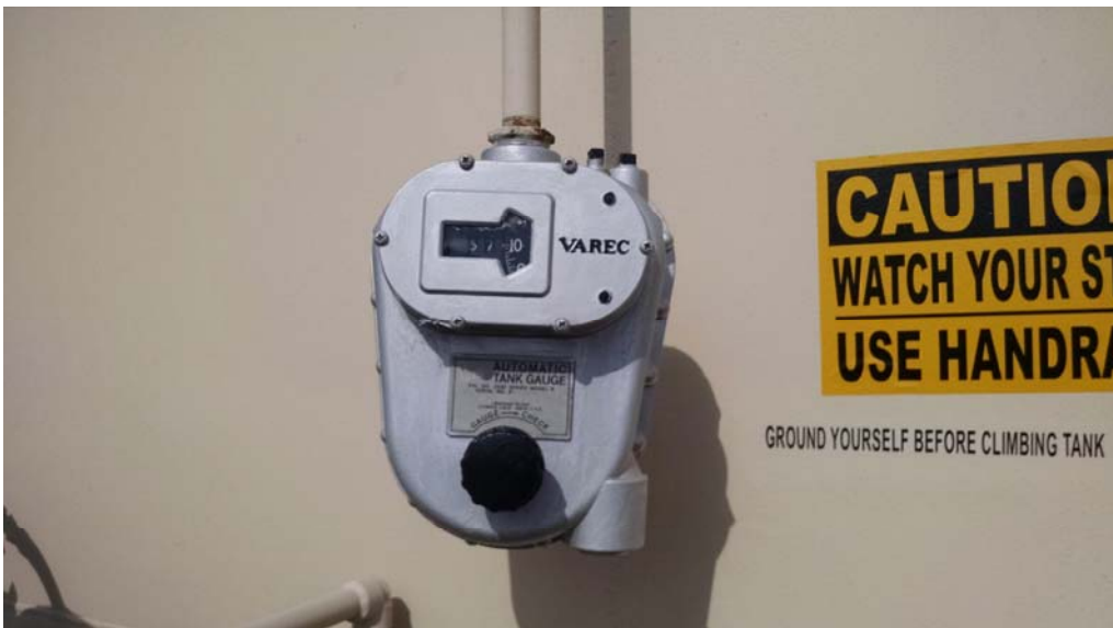
E.17 Mechanical Type Level Gauge
