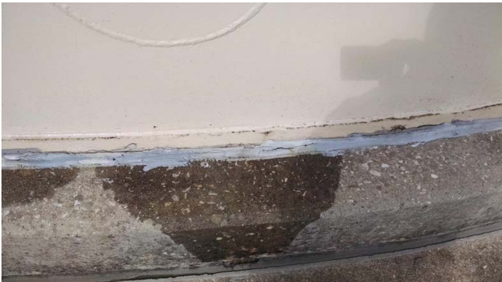
E.21 Failed Area of Bottom-to-Foundation Sealant
