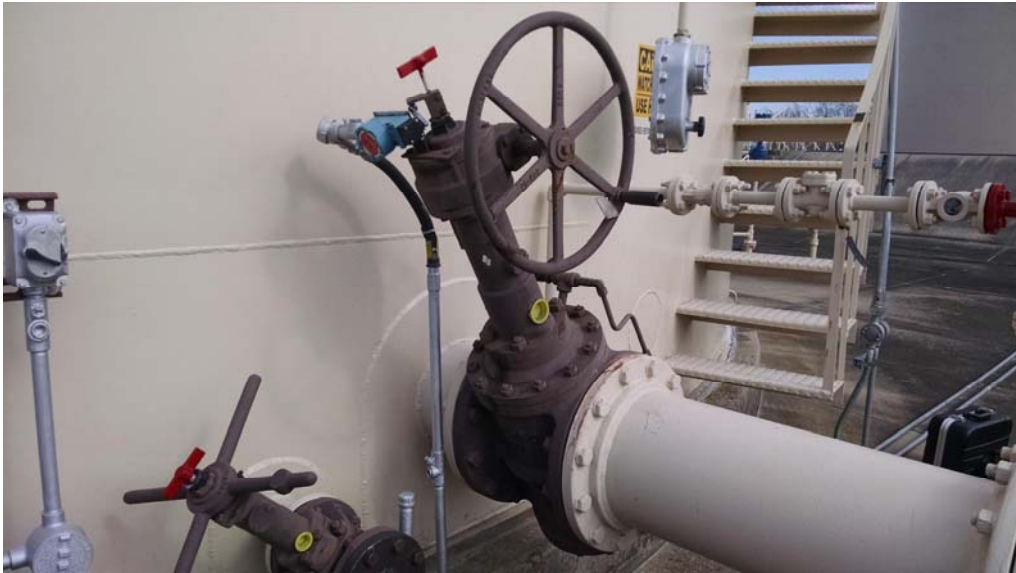
E.10 Shell Nozzle D, 12" Tank Receipt
