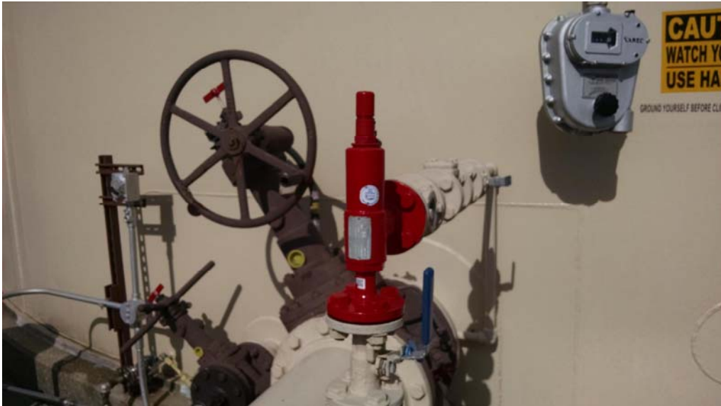
E.13 Thermal Relief System
