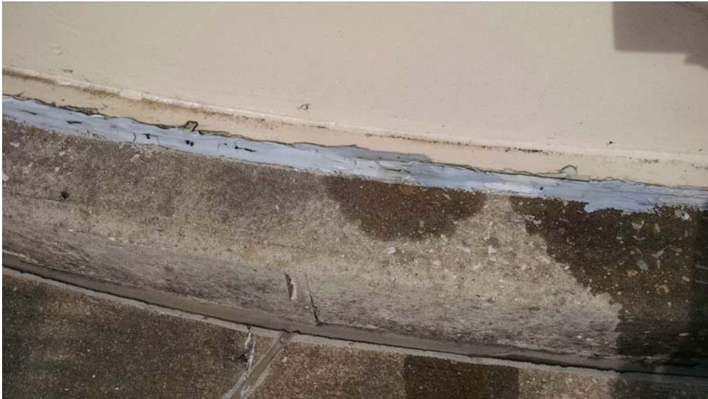
E.22 Failed Area of Bottom-to-Foundation Sealant
