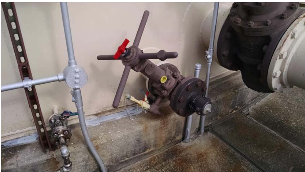
E.9 Shell Nozzle C, 4" Low Point Suction
