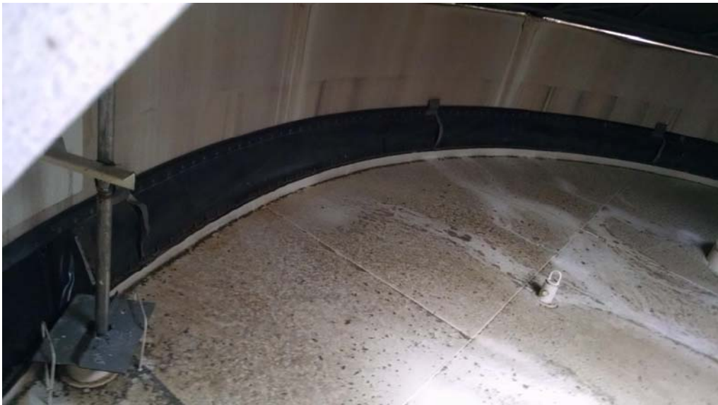
E.44 Internal Seal for IFR
