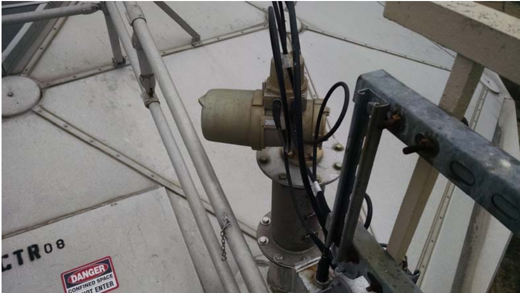
E.37 View of ENRAF Tank Gauging System
