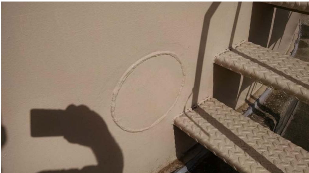
E.15 Replaced Butt-Welded Insert Plate
