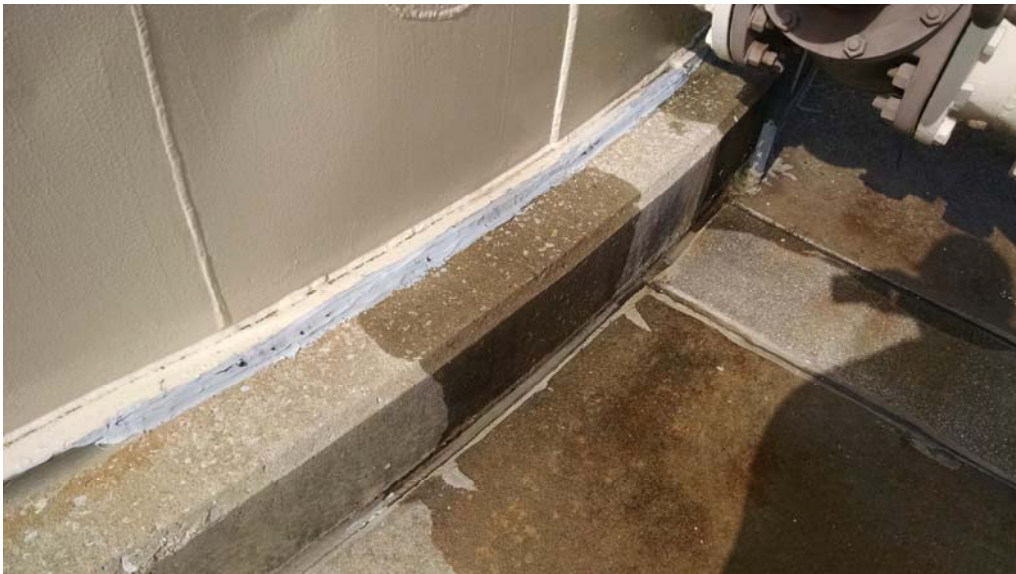
E.23 Failed Area of Bottom-to-Foundation Sealant
