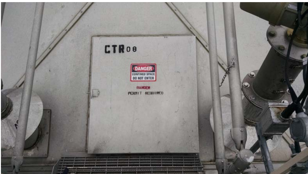
E.39 Hatch to Access Floating Roof
