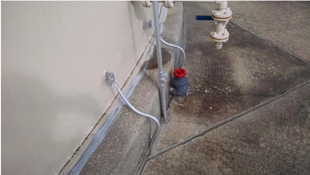
E.25 Tank Grounding and Leak Detection Port
