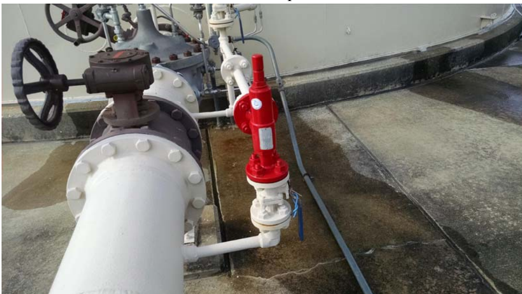
E.30 TRV's Have Current Calibrations
