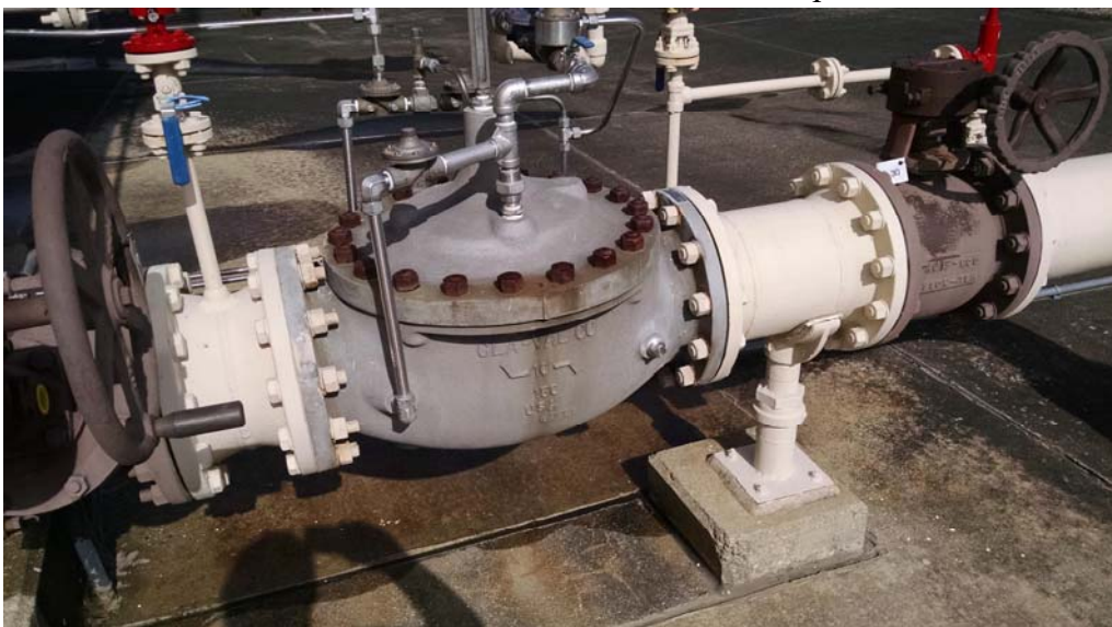
E.27 Automatic Shut-Off Valve
