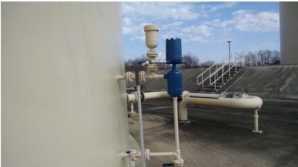
E.24 Shell Nozzles E and F, 1" Low Level Alarm
