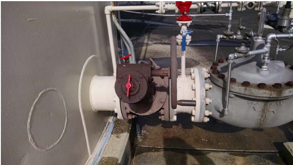
E.26 Shell Nozzle G, 10" Tank Receipt
