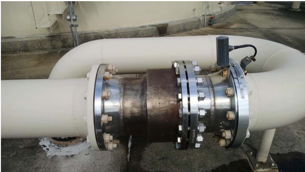
E.11 Expansion Joint in 12" Line
