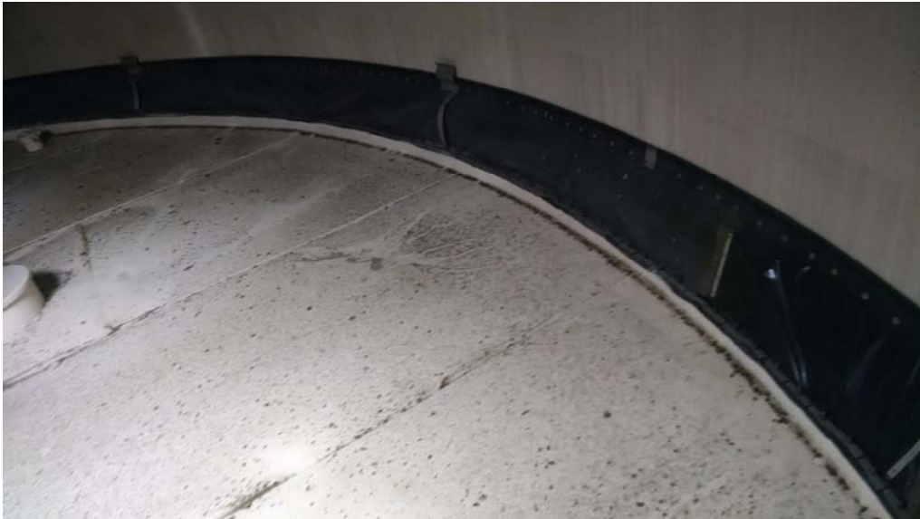
E.43 Internal Seal for IFR
