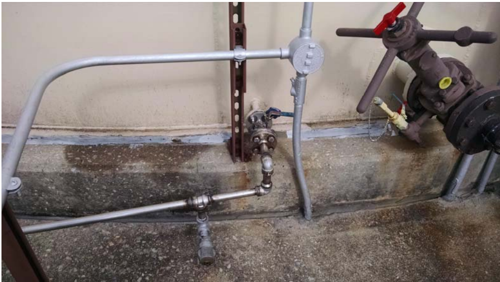
E.8 Shell Nozzle B, 1" Water Draw
