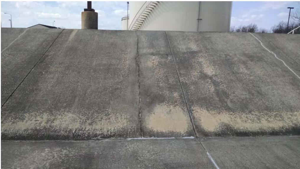
E.32 Large Crack in Containment Wall
