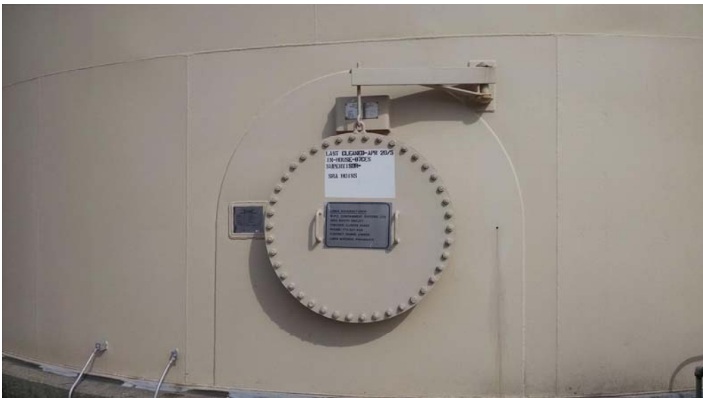
E.2 Shell Nozzle A, 36" Manhole
