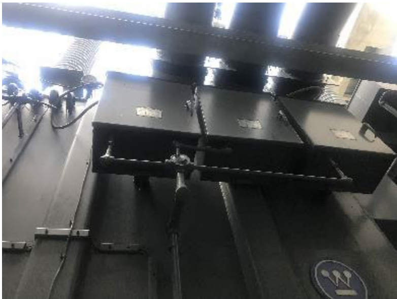
BUSHING POTENTIAL DEVICES (BPD)
