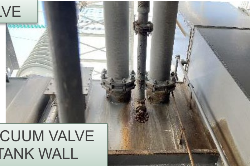
CONSERVATOR TANK OIL PIPING CONNECTION
