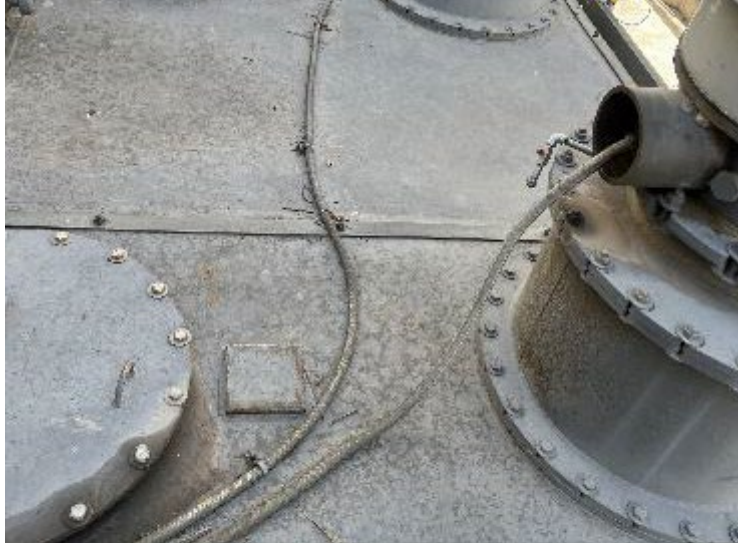
MANHOLE GASKET AND BUSHING POTENTIAL TAP
