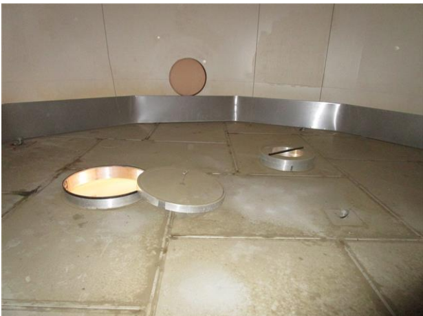
C47: Internal Floating Roof Overview
