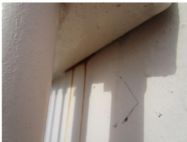
C18: Conduit Support w/ Crevice Corrosion
