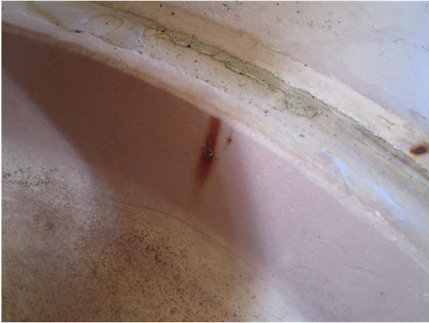
C43: Coating Failure at Center Sump
