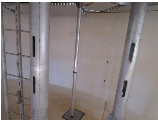
C36: Partially Slotted Stilling Wells
