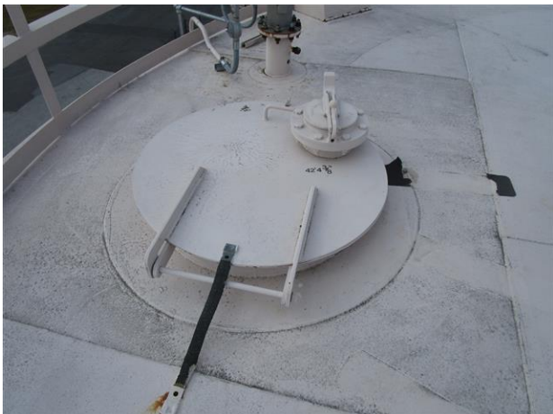
C29: Fixed Roof Manway w/ Access Ladder and Gauging Hatch
