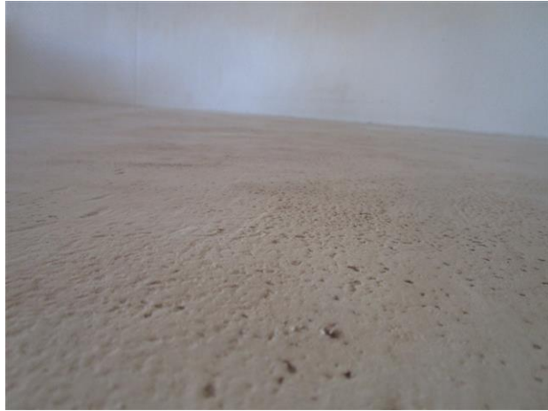
C38: Wide Spread Pitting along the Tank Bottom
