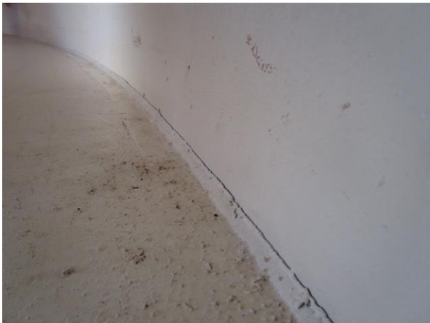
C39: Cracked Coating along the Internal Shell-to-Bottom Weld
