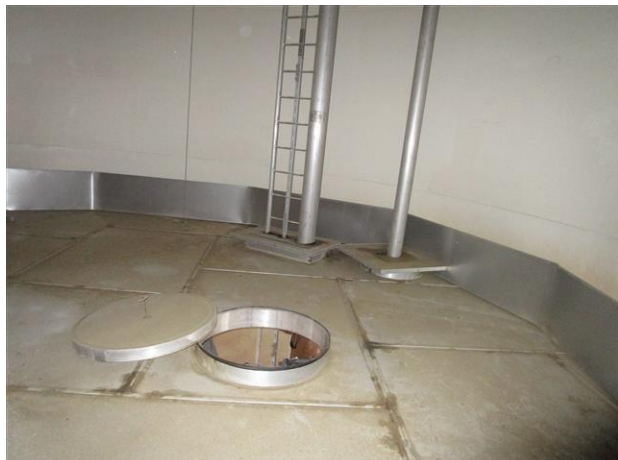
C48: Internal Floating Roof Overview
