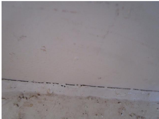
C40: Cracked Coating along the Internal Shell-to-Bottom Weld
