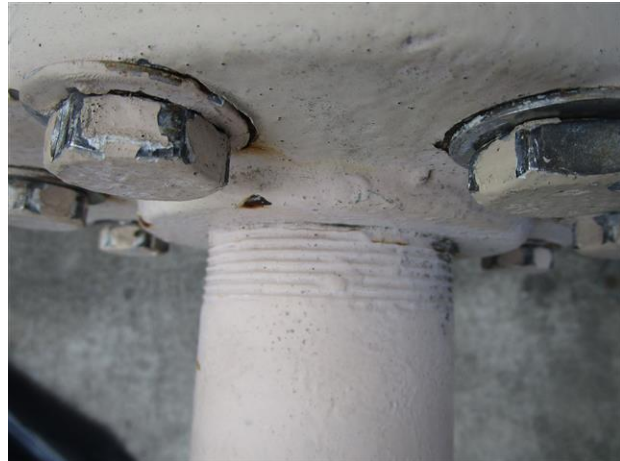
C10: Threaded Connection on Low Suction
