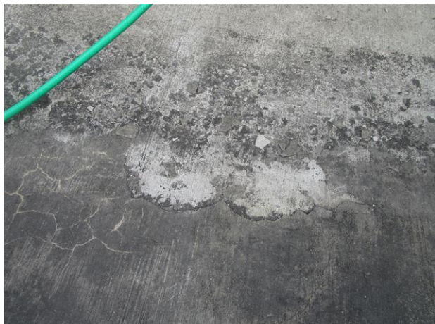
C24: Cracking and Spalling in Containment Dike
