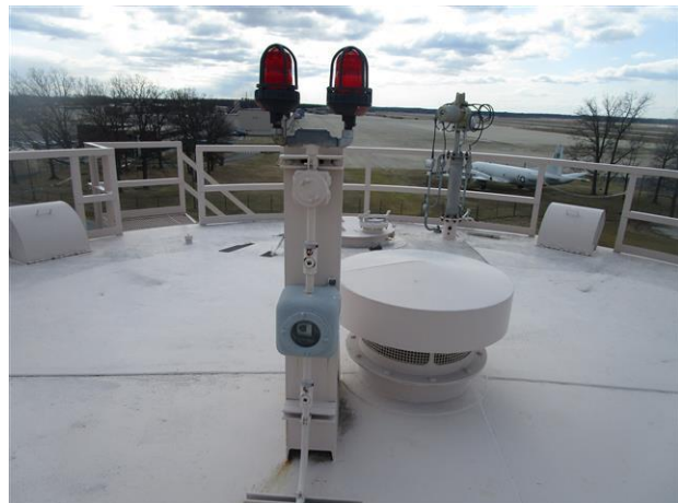
C30: Visible Alarms and Center Vent
