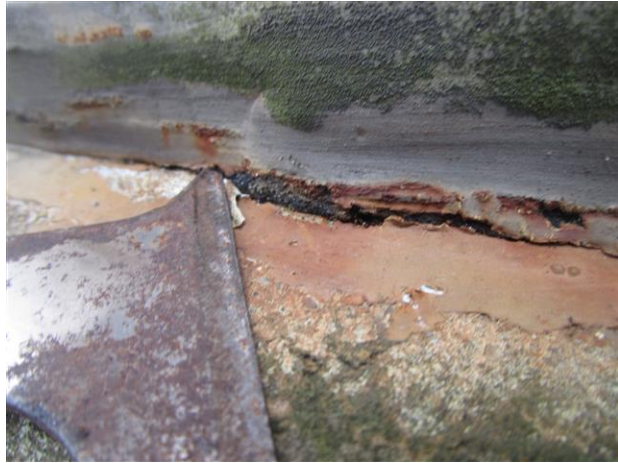
C20: Tank Chime Sealant Failure
