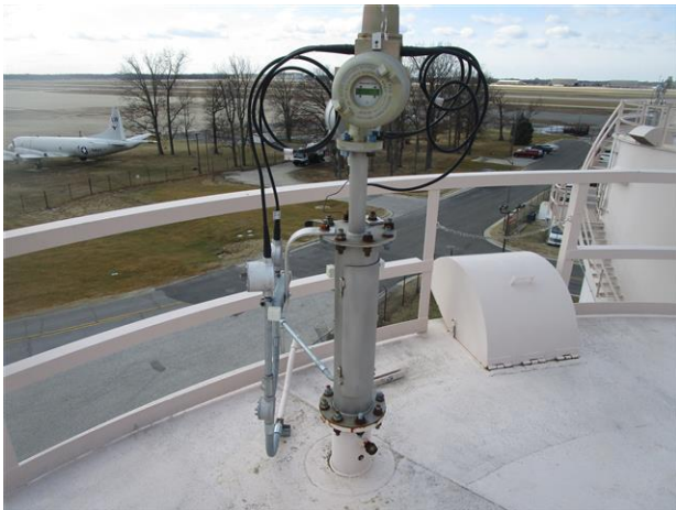
C27: Enraf ATG / VITO Temperature Probe
