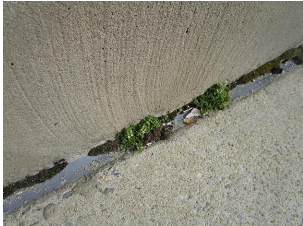
C22: Vegetation in Ring Wall Control Joint
