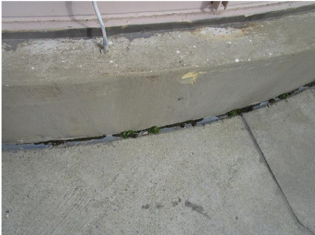
C21: Vegetation in Ring Wall Control Joint
