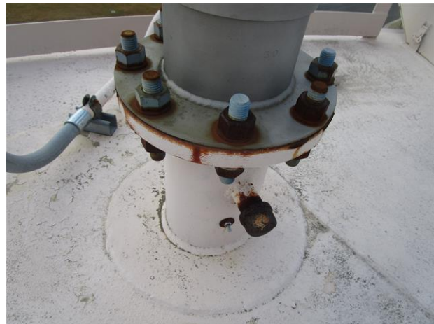
C28: Corroded Fasteners on Enraf ATG
