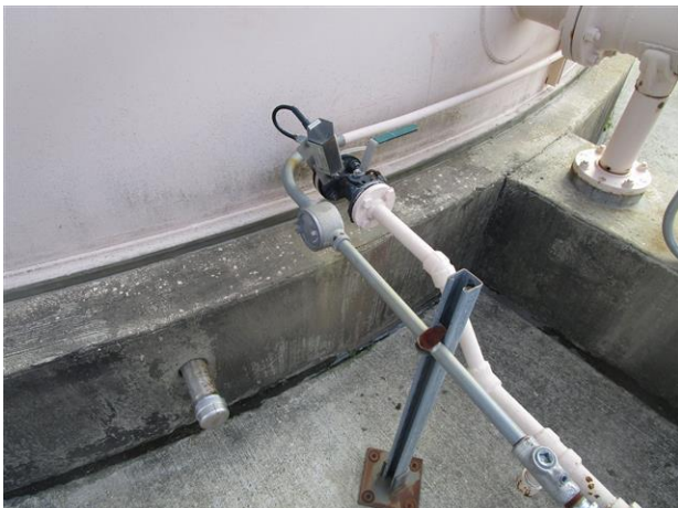
C11: Water Draw-Off with Ball Valve
