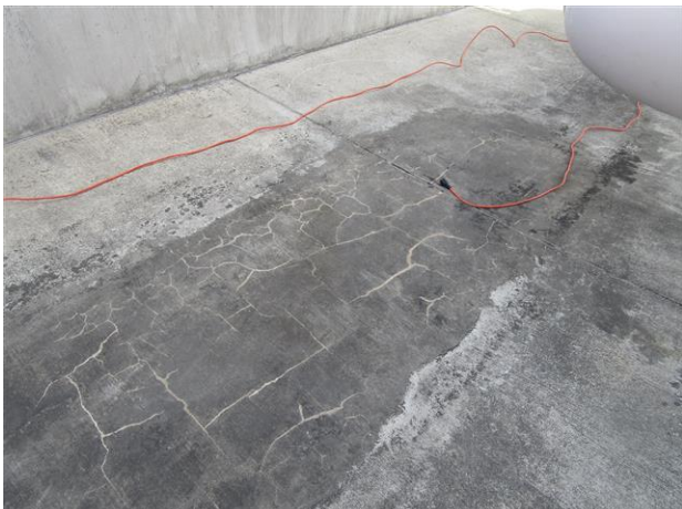
C23: Cracking in Containment Dike
