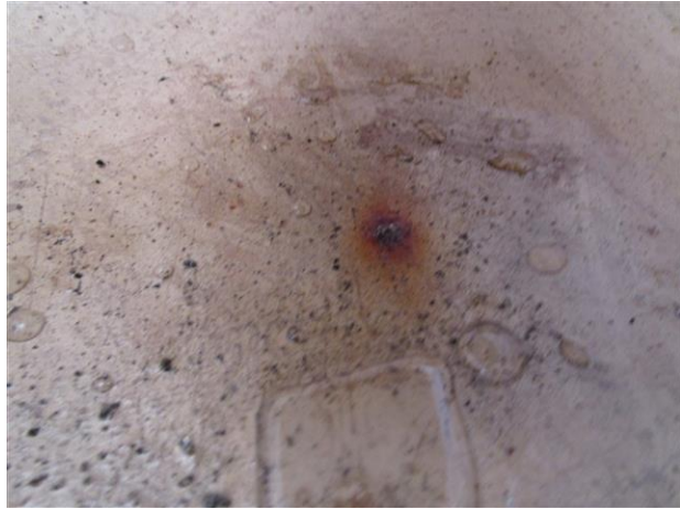
C44: Coating Failure at Center Sump
