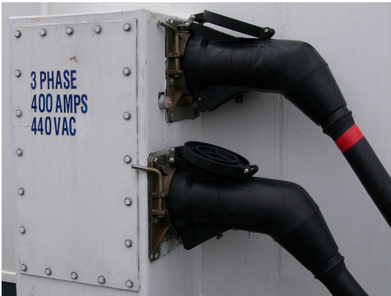
Below: Angled plugs, factory vulcanized
