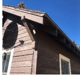
Exposed Rafter Tails to be covered
