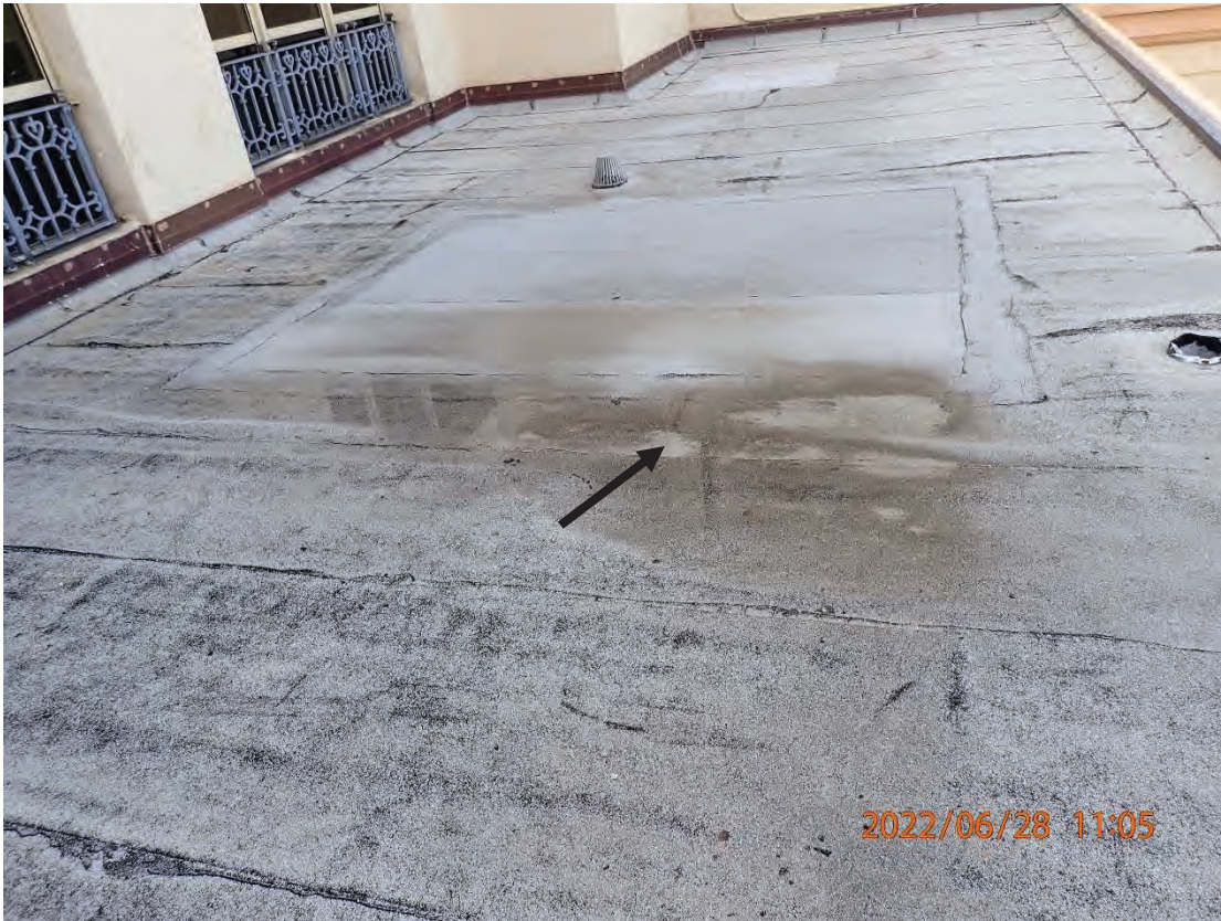
Figure 11: Overview of IR Anomaly at Area A Loading Dock Roof (arrow)
