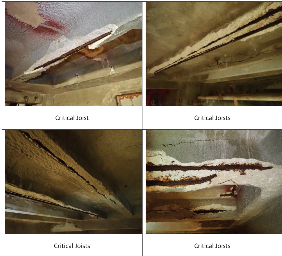
Figure 3: Critical joists bound by columns 167-180-181-172-172A-168-167 in Crawlspace B
