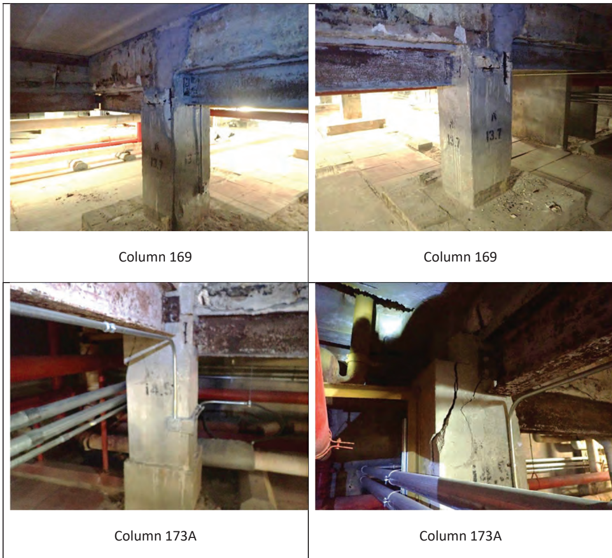
Figure 2: Critical columns 169 and 173A in Crawlspace B
