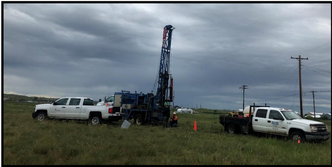
Drilling Boring B-6 – View North – Mobile B-59 Truck-Mounted Drill Rig
