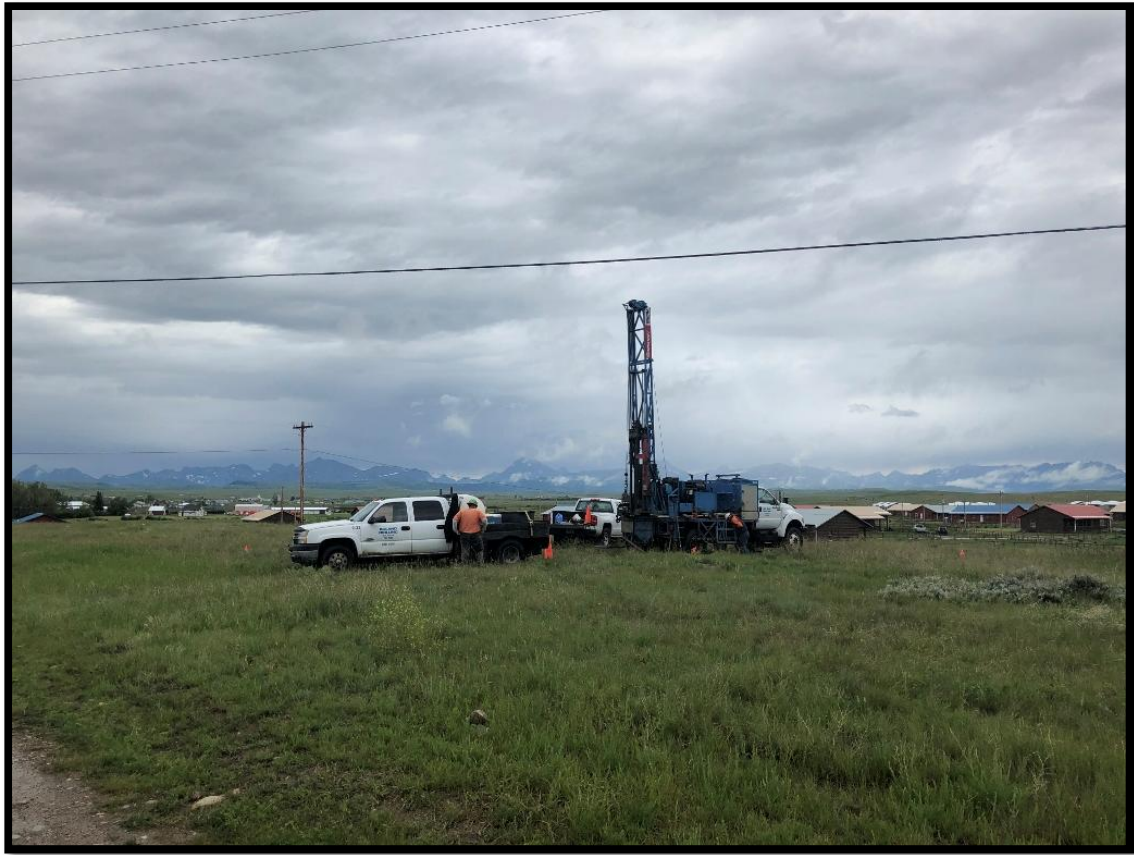
Drilling Boring B-6 – View Southwest – Mobile B-59 Truck-Mounted Drill Rig
