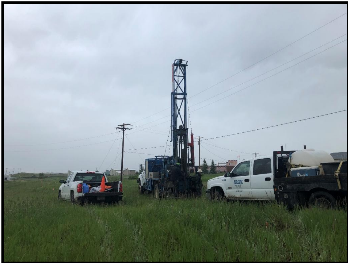
Drilling Boring B-5 – View North – Mobile B-59 Truck-Mounted Drill Rig
