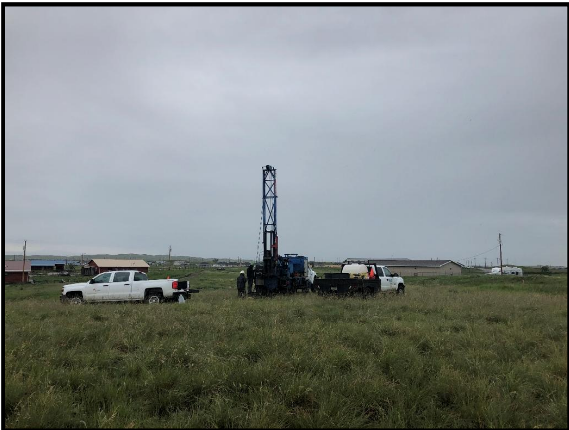
Drilling Boring B-3 – View Northwest – Mobile B-59 Truck-Mounted Drill Rig
