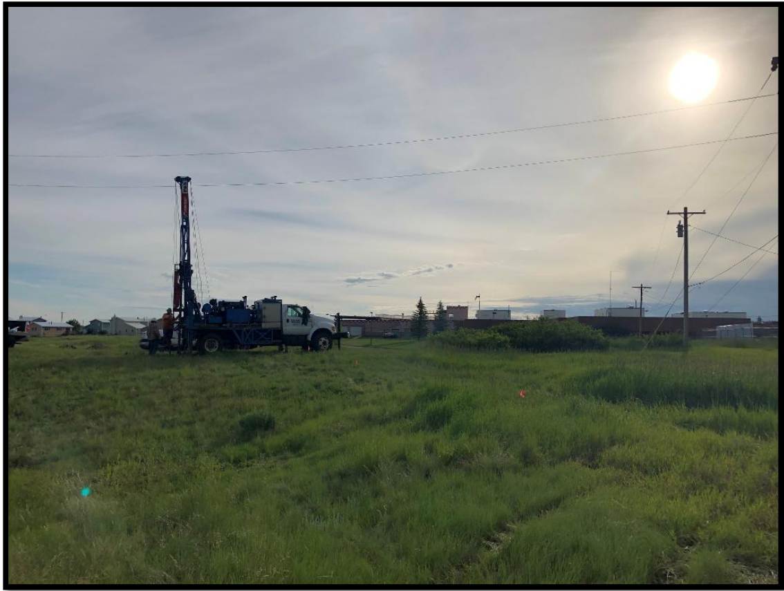
Drilling Boring B-1 – View Northeast – Mobile B-59 Truck-Mounted Drill Rig
