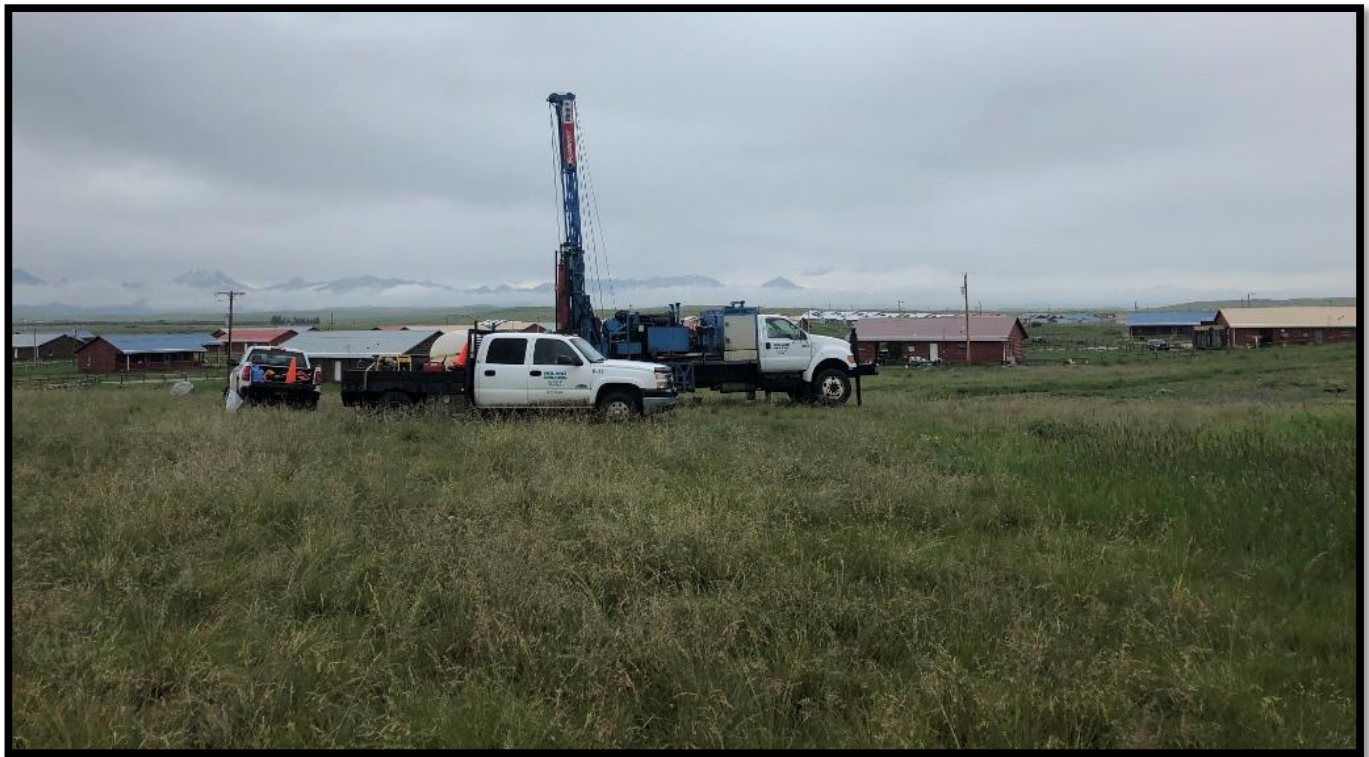
Drilling Boring B-3 – View West – Mobile B-59 Truck-Mounted Drill Rig
