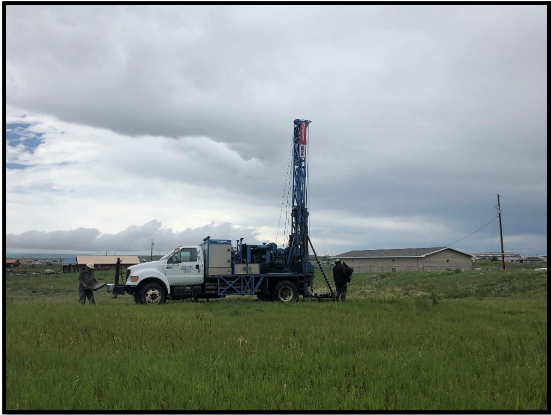
Drilling Boring B-2 – View Northwest – Mobile B-59 Truck-Mounted Drill Rig
