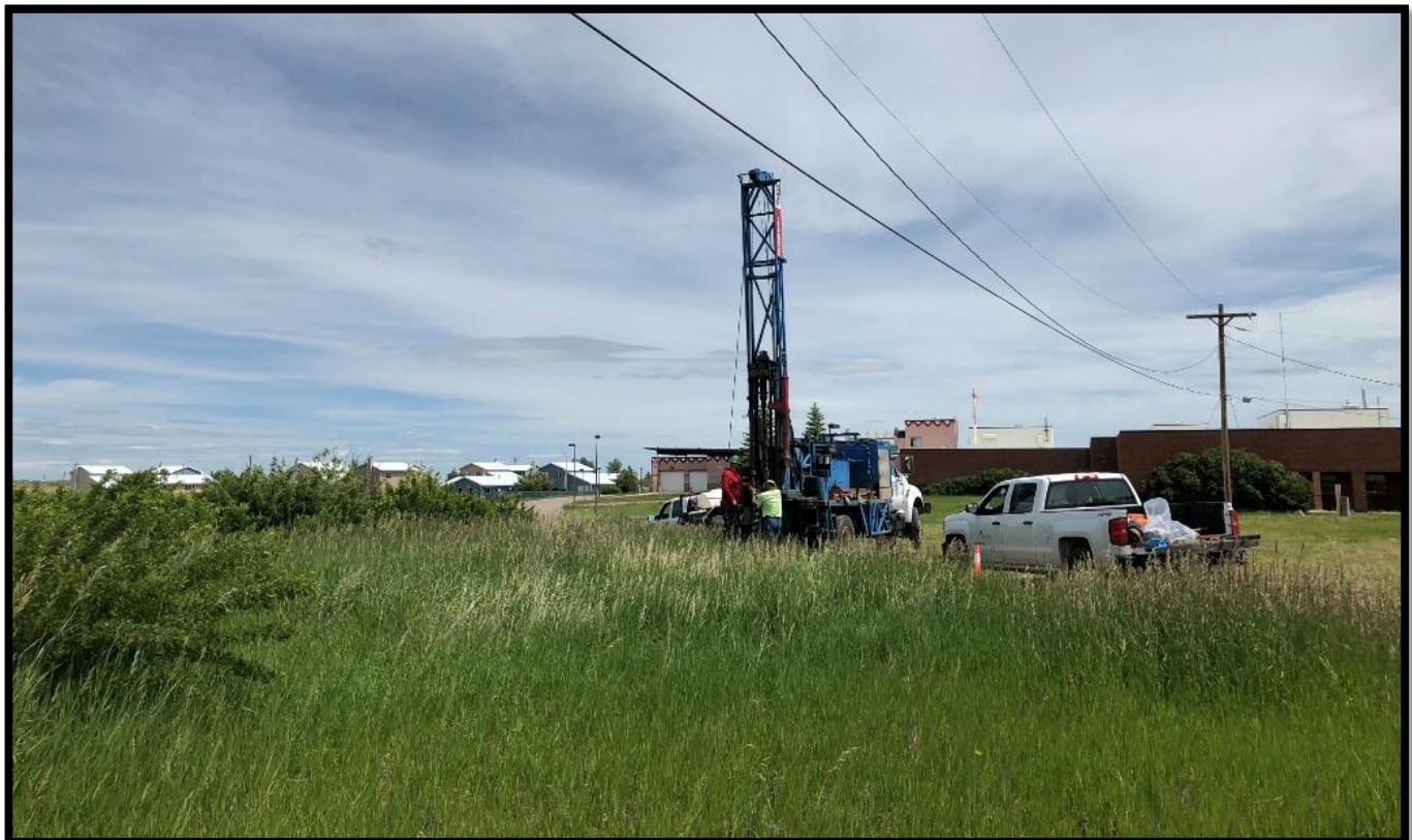
Drilling Boring B-7 – View Northeast – Mobile B-59 Truck-Mounted Drill Rig
