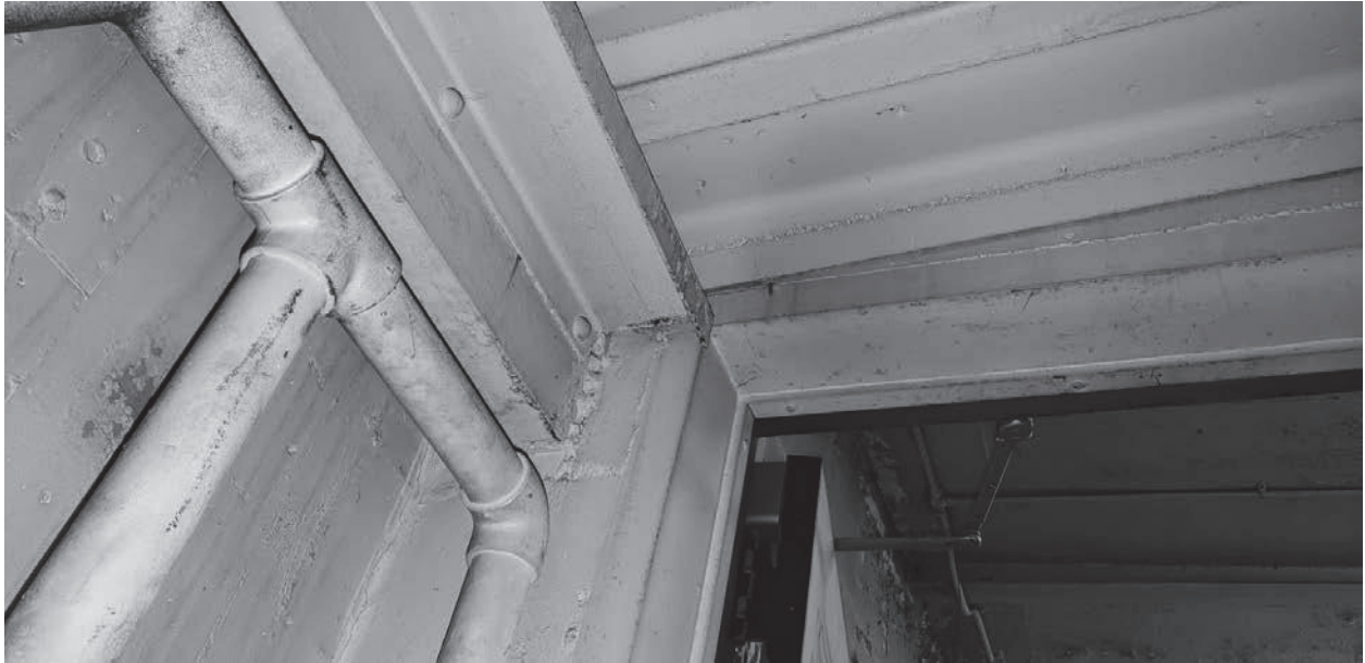
Photograph 26 – Assume all structural steel is positive for lead paint.
