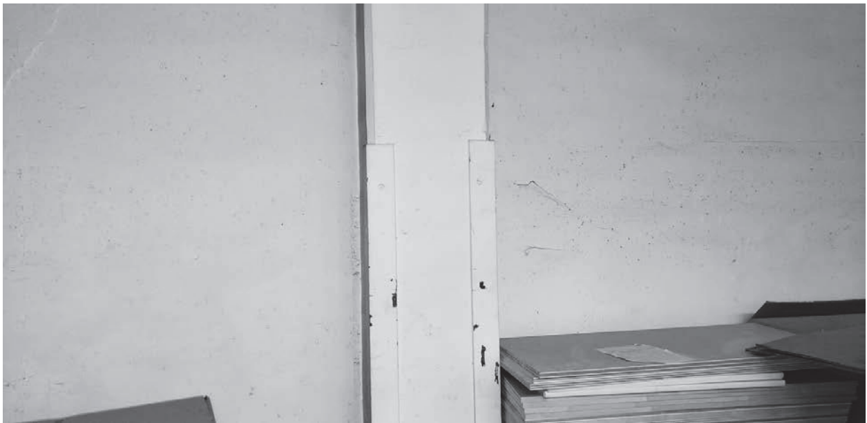
Photograph 16 - Column is negative for lead paint.
