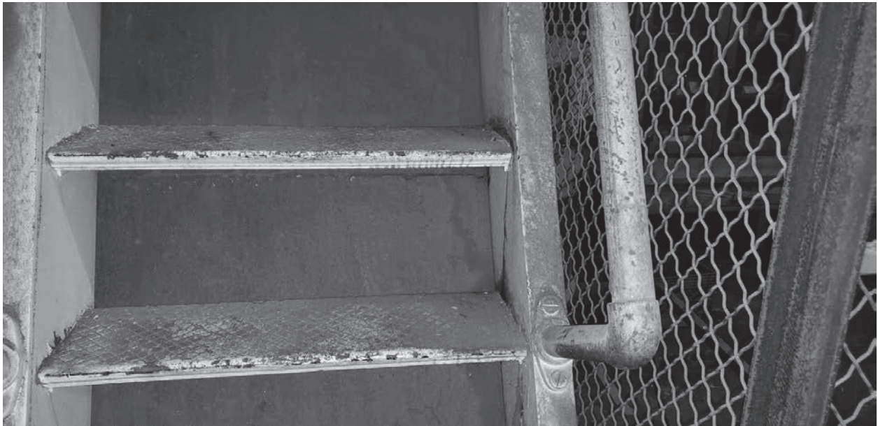
Photograph 4 - North wall staircase with factory applied lead primer on rails, treads, and stringer.
