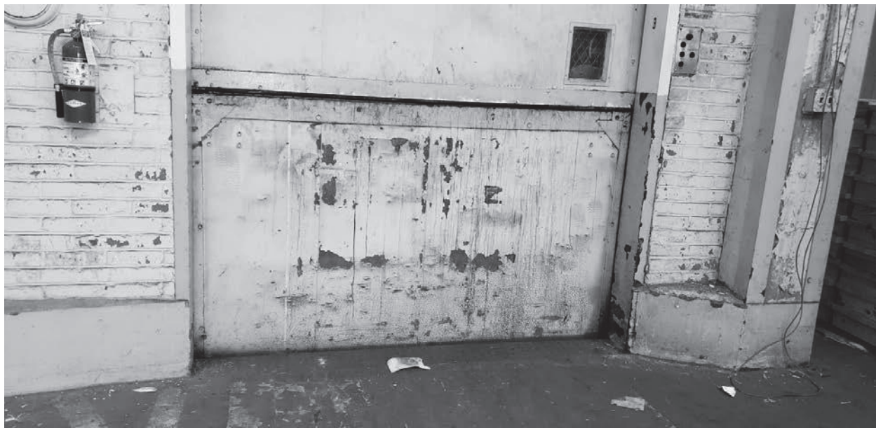
Photograph 17 – Consider all these components are positive for lead paint.
