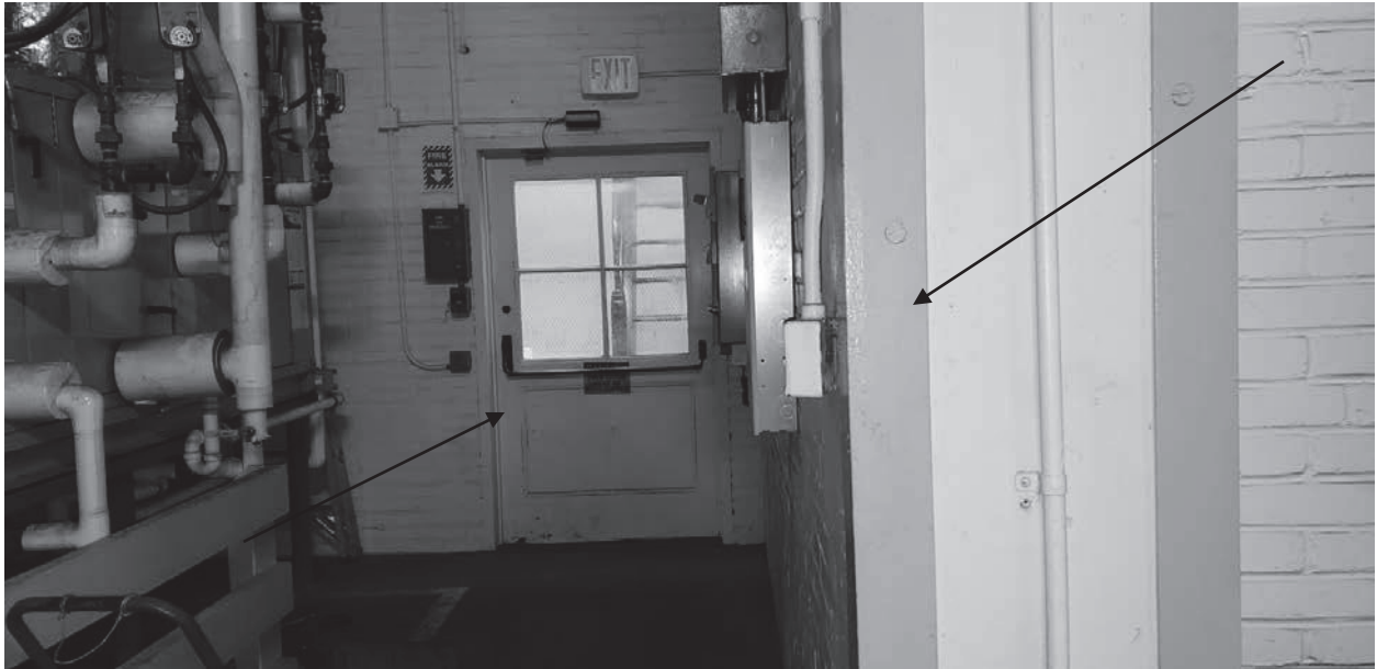
Photograph 1 – Corner on right is positive for LBP (Lead Based Paint). Door to stairs is positive.
