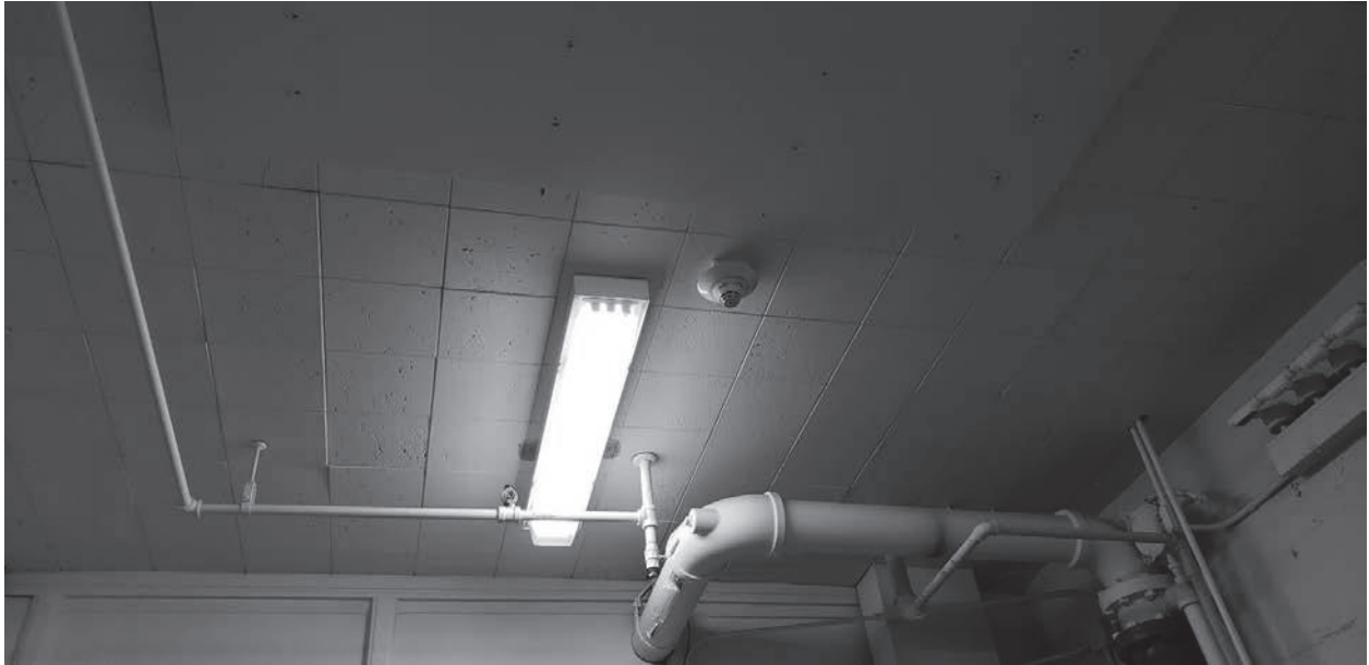
Photograph 19 – Small office off north wall with 12” ceiling tile (negative) for asbestos.
