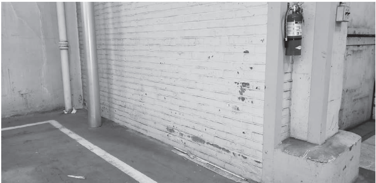
Photograph 12 - South Elevator wall is painted brick with latex. No LBP.
