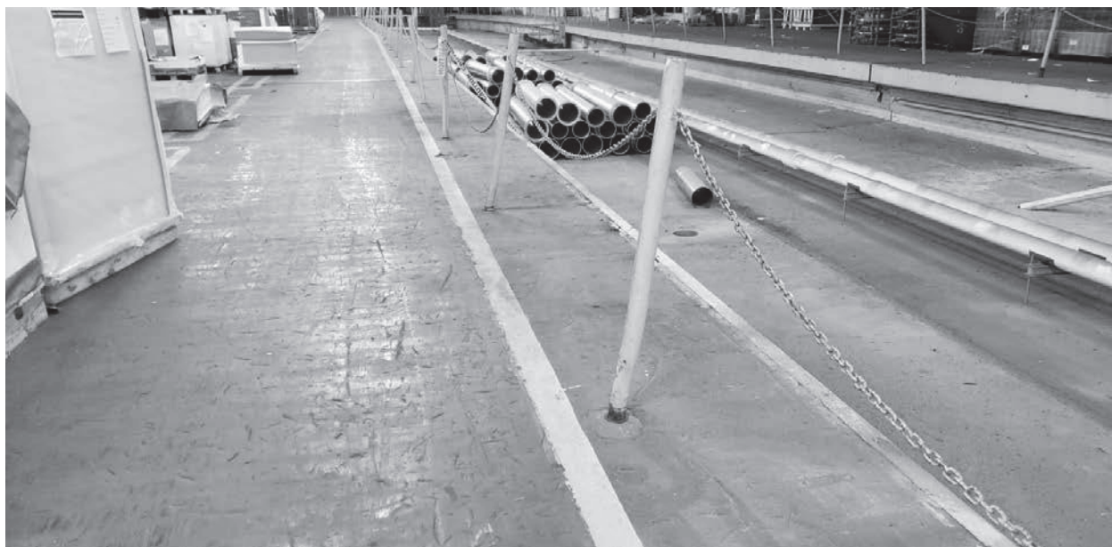
Photograph 10 - Painted rubber floor is positive but yellow post is negative.
