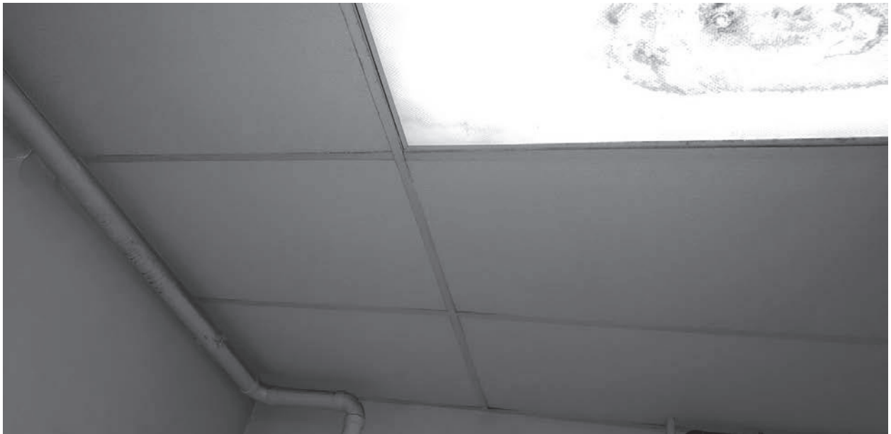
Photograph 22 - Ceiling tile in men's room of Photograph 23 – was negative for asbestos.
