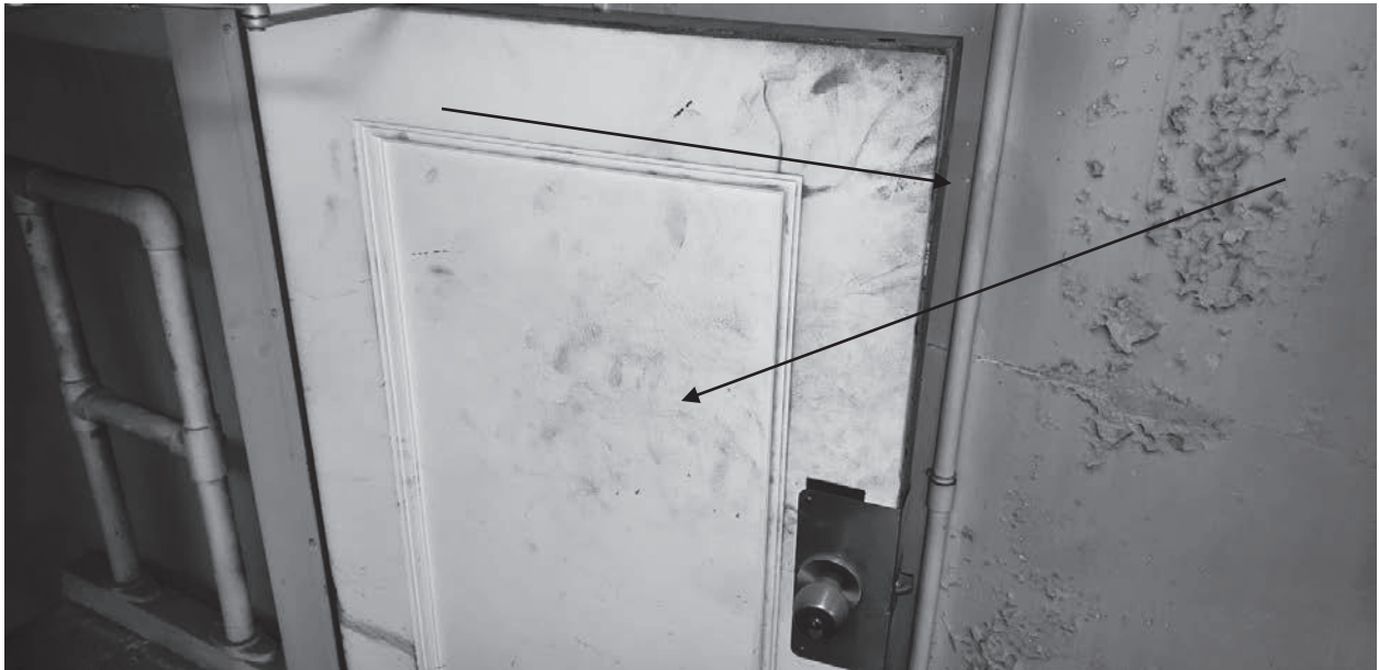
Photograph 8 - Double door & frame is positive for LBP. ( 2' X 3')
