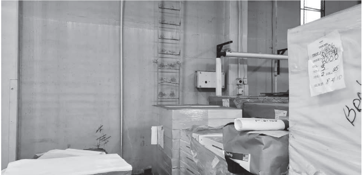
Photograph 11 – North wall ship ladder is factory applied and positive.
