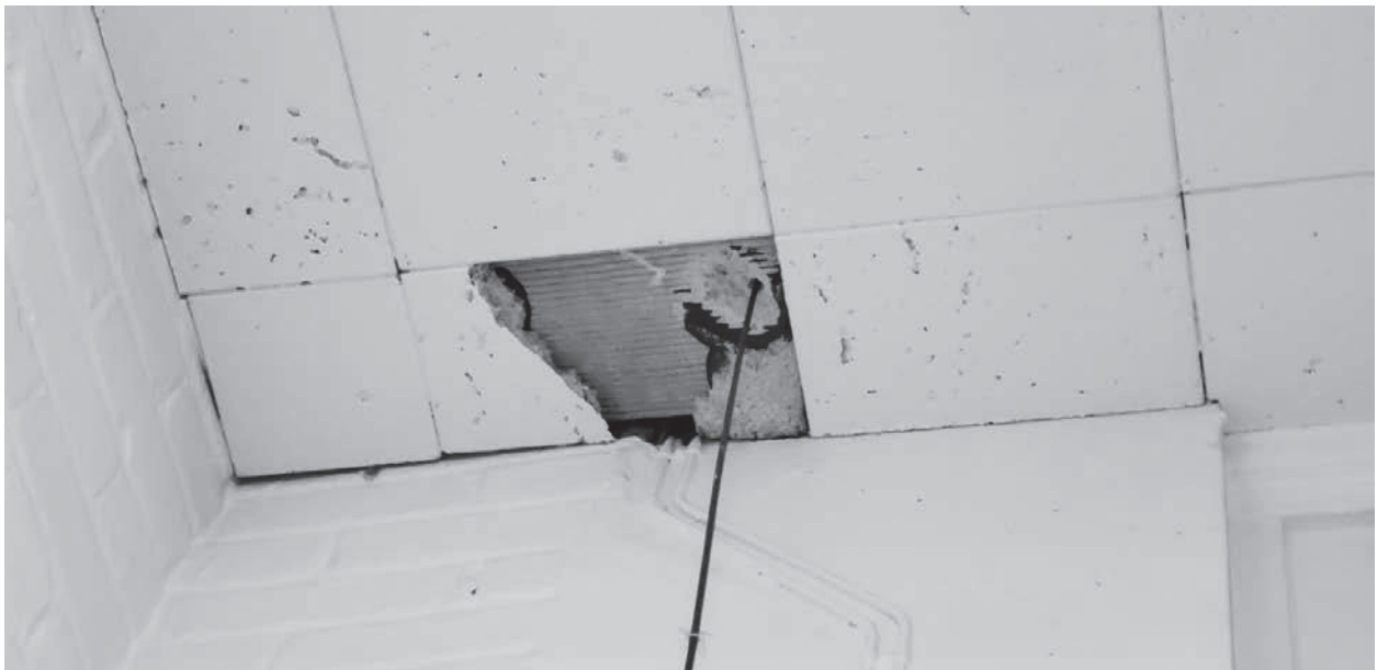
Photograph 20 - Same office with 12” ceiling spline tile – negative for asbestos
