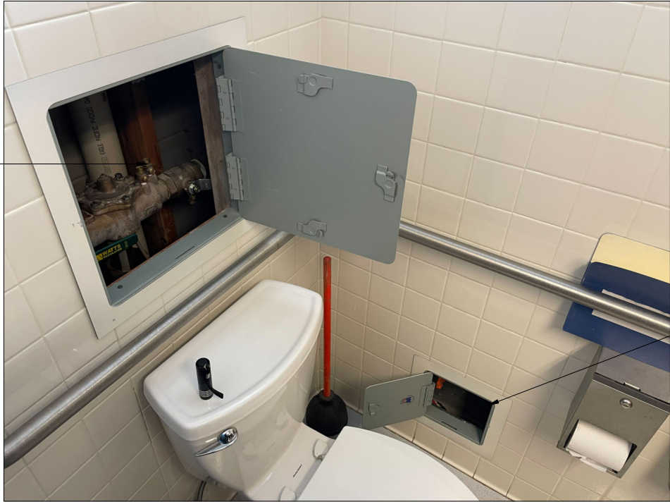
OFFICE (BLDG #D2004) EXISTING WATER SERVICE
