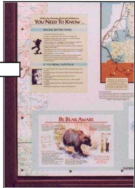
Figure 10B-28—The digital laminate sign is attached to MDO by adhesive and metal screws.
