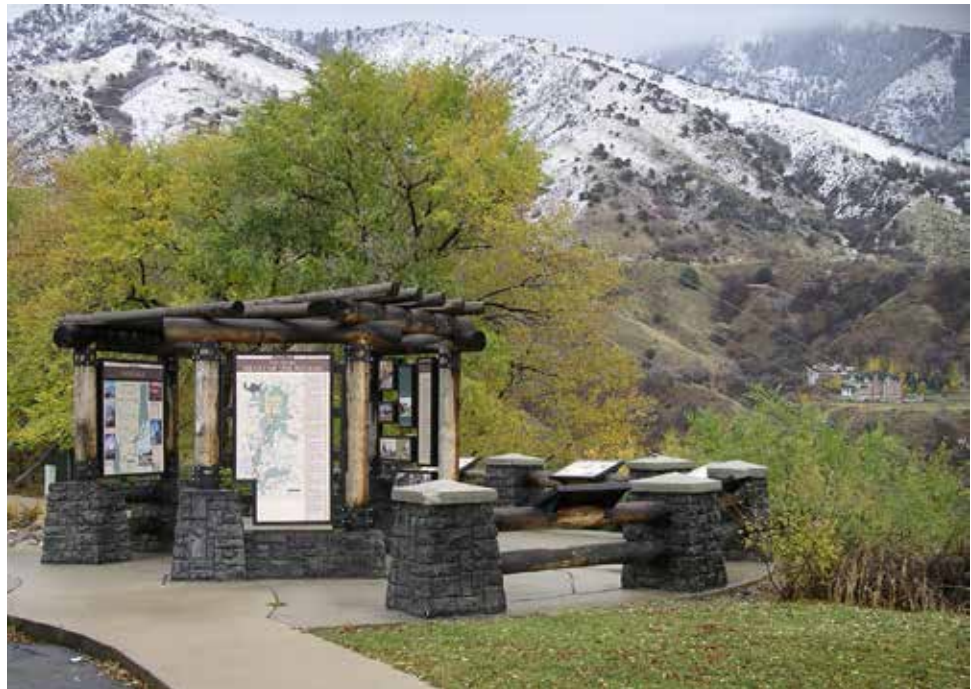
Figure 10A-25—Local stone and timbers were used to build this kiosk and overlook. Logan Canyon Scenic Byway, Wasatch-Cache National Forest. Rocky Mountain BEIG Province.
