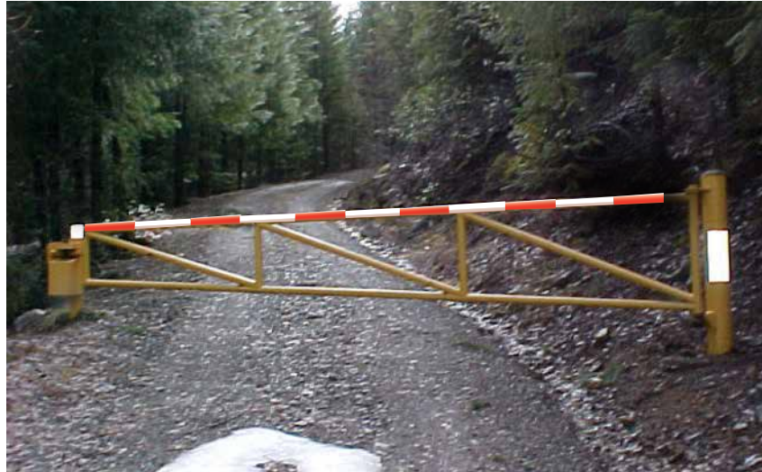
Figure 3B-1—Retroreflective tape on gate arm.
