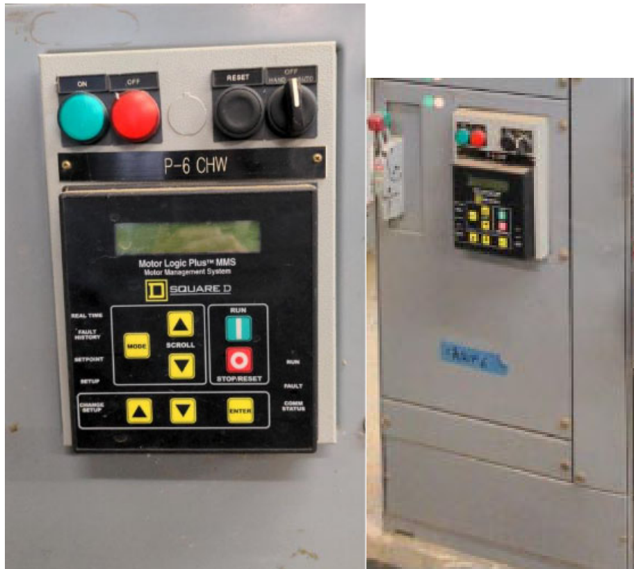
Existing MCC disconnect and starter for CWHP-6
