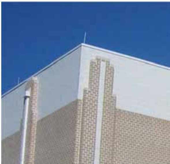
Pilaster details are prevalent on high bay buildings, usually aligned with scuppers and downspouts;
