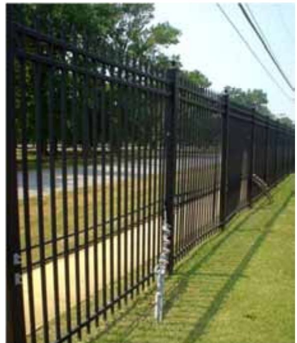
This fence design uses exposed cable reinforcing
