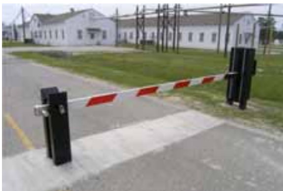
Crash-rated vehicle barrier across service driveway. If this type of barrier is required, it should be tied into a system of barriers which prevent by-pass.
