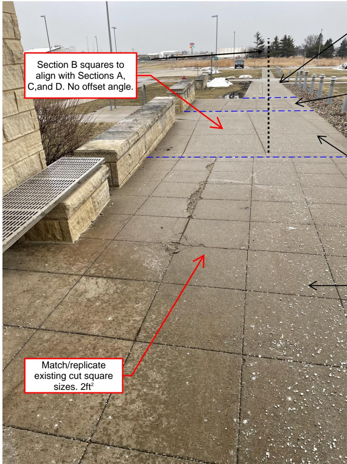
Section B squares to align with Sections A, C, and D. No offset angle.
