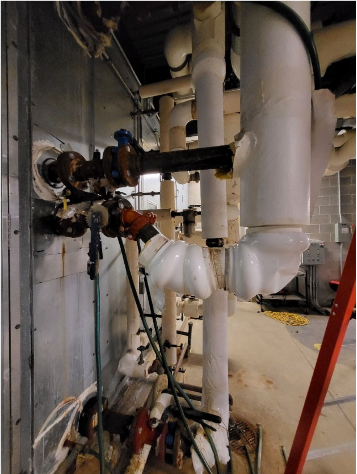
Photograph 3: View of chilled water supply piping connections to upper and lower coils at AHU-1.
