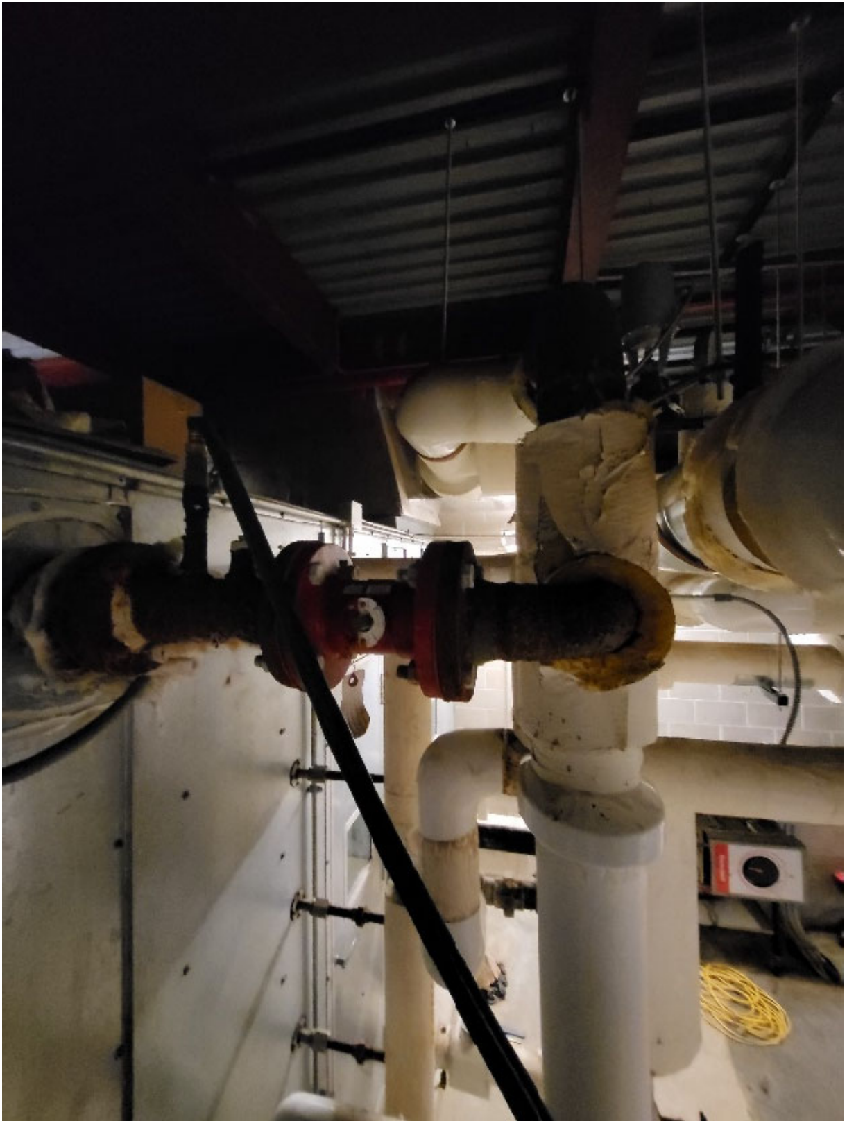
Photograph 4: View of chilled water return connection to upper coil at AHU-1.
