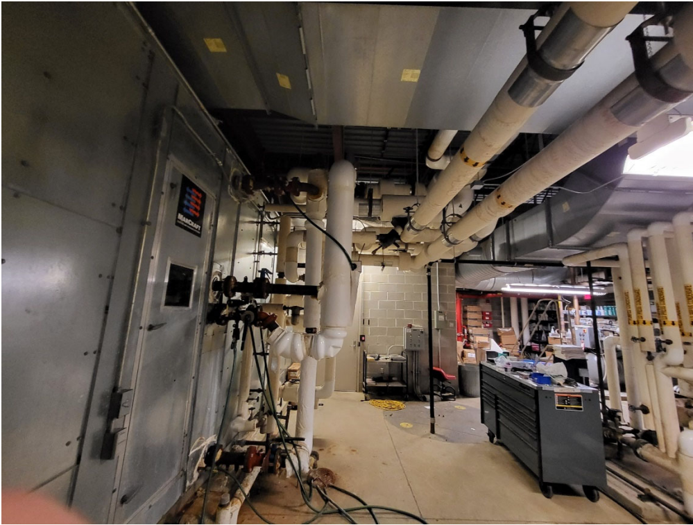
Photograph 1: View of chilled water piping connections to coils at AHU-1.
