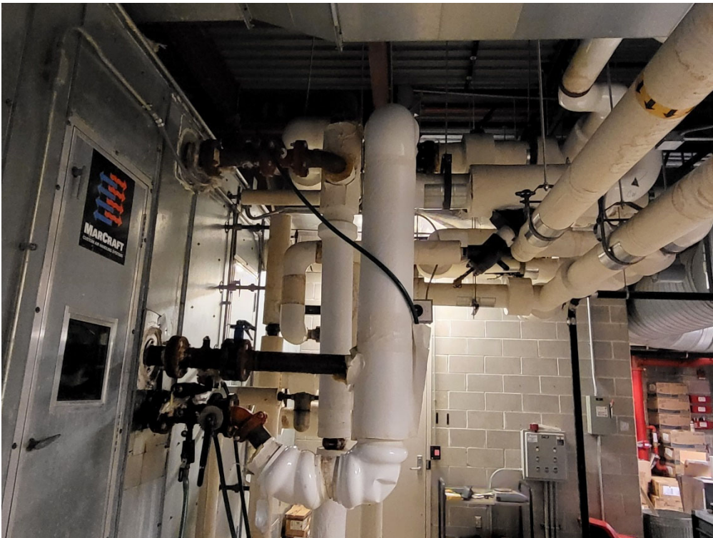
Photograph 2: View of chilled water piping connections to coils at AHU-1.
