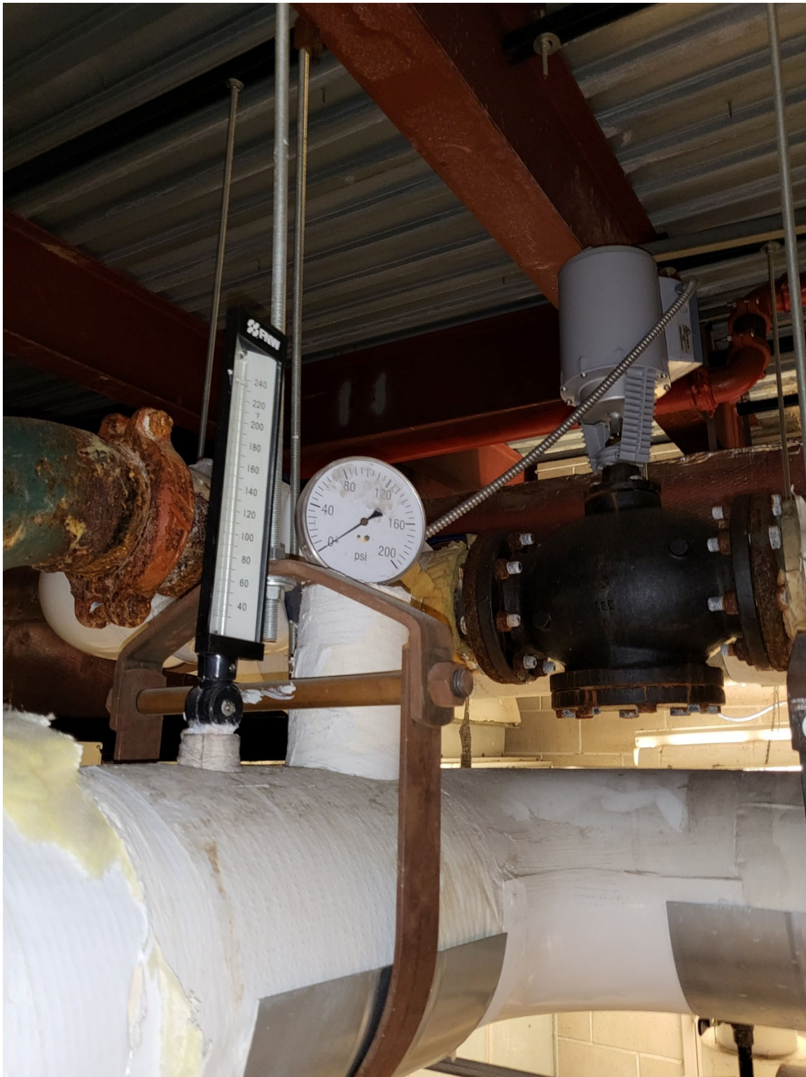
Photograph 6: View of control valve on 6" return line to AHU-1.
