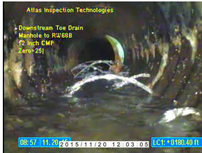
Figure 1-10: Left abutment relief well collector system pressurized area by RW-68B T-outfall
