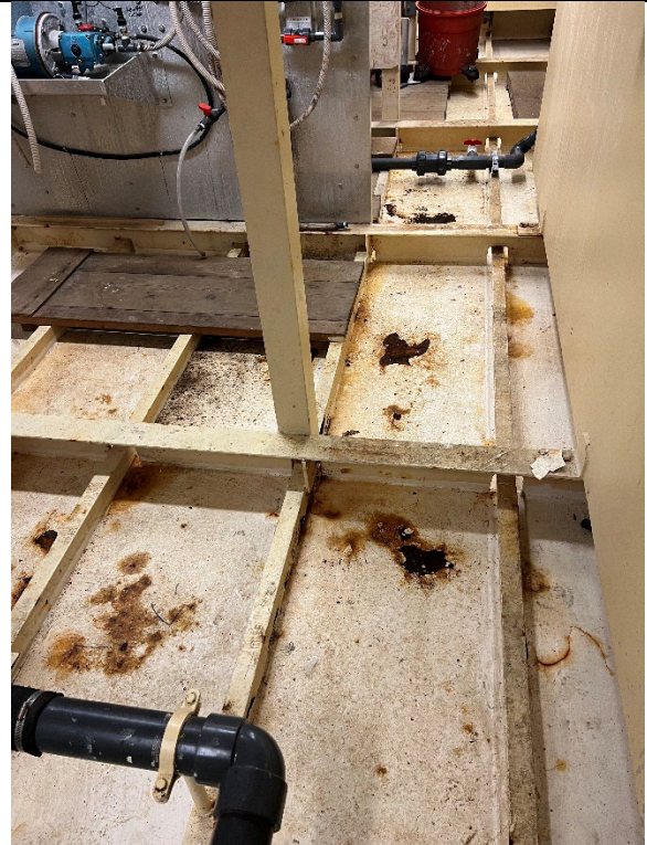
Spot paint areas of rust in main compartment
