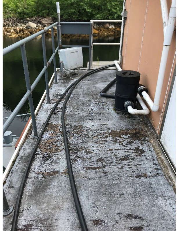
Forward rotting plywood deck
