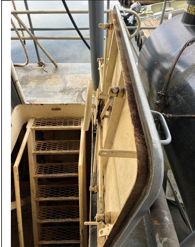
Main Hatch has rust around lip observed
