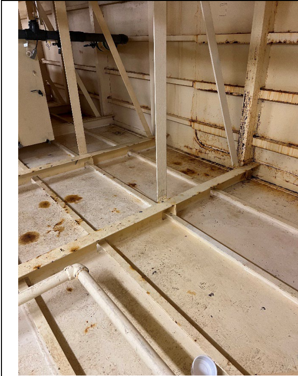
Spot paint areas of rust in main compartment
