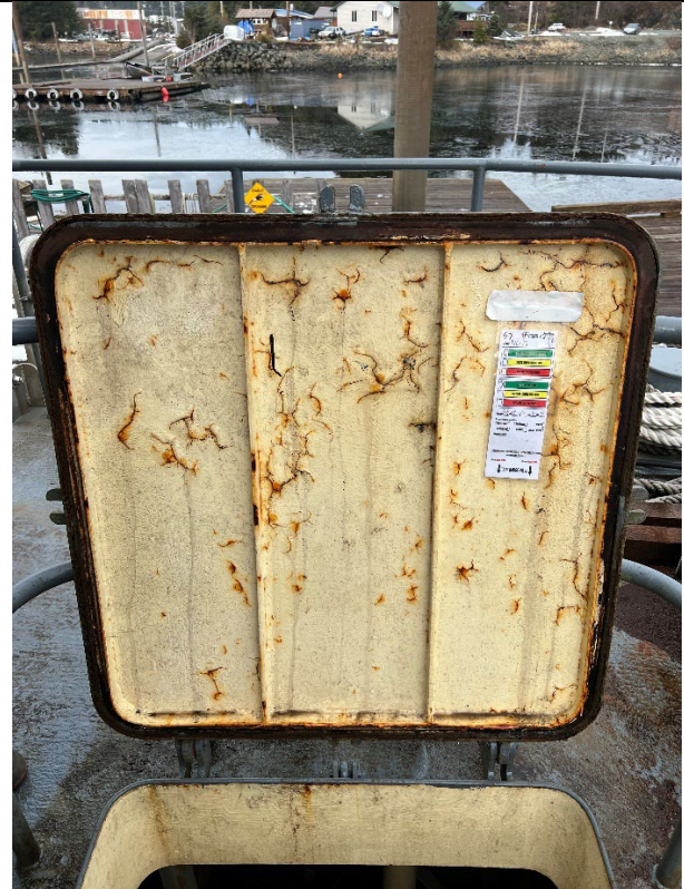
Hatch lid to be repainted and seal replaced
