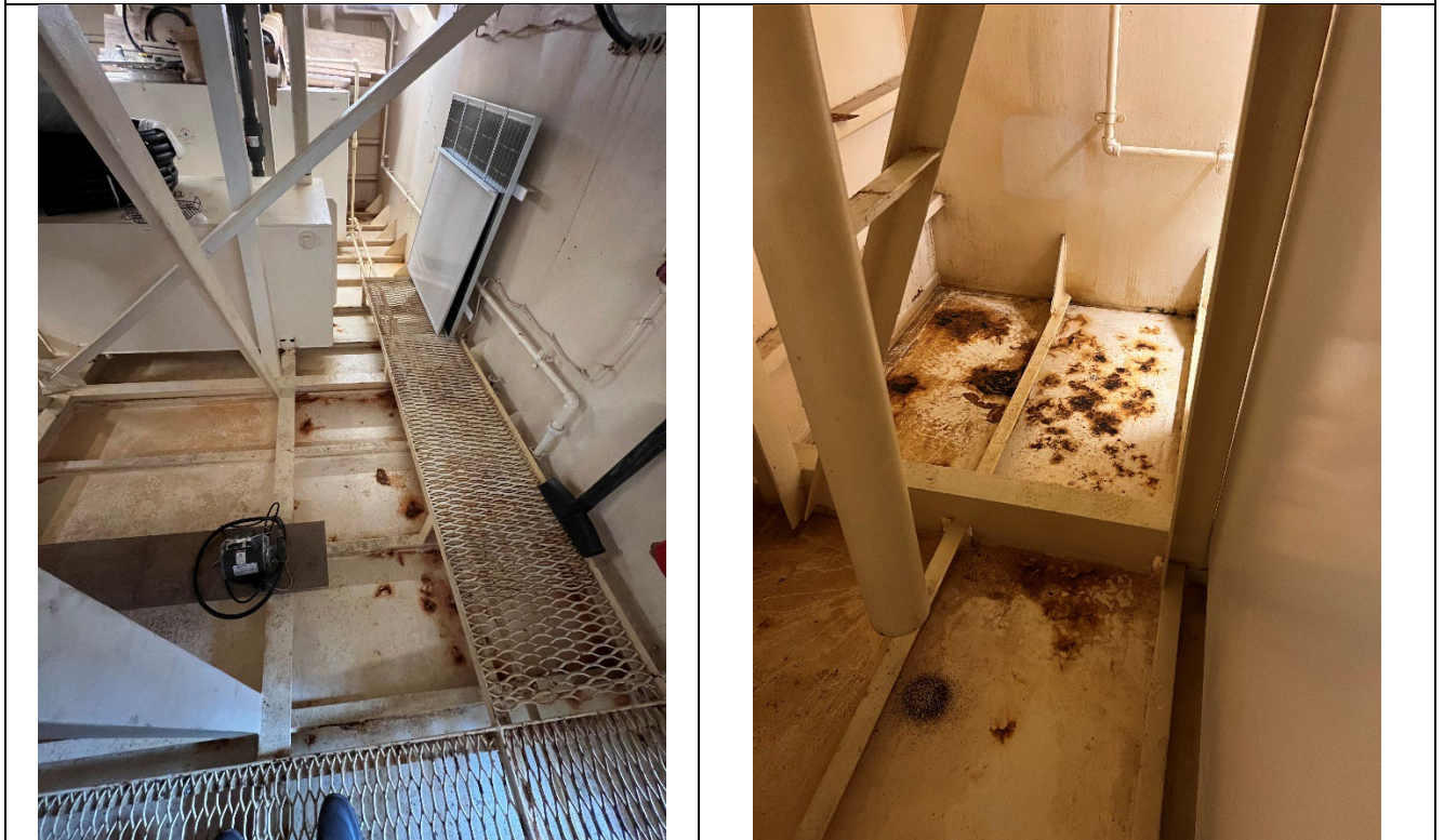
Spot paint areas of rust in main compartment
