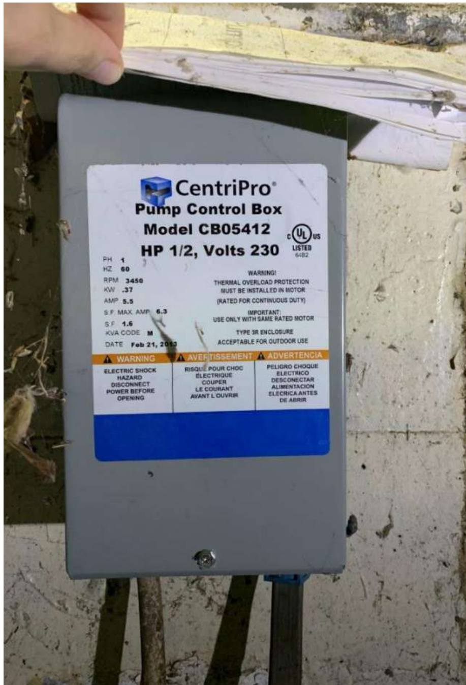
Figure 25 – Existing Pump Control Box (to be demolished)
