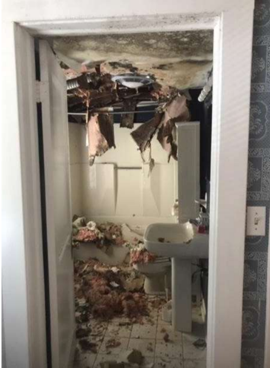
Figure 14 – 2 nd Floor Restroom (water damage)
