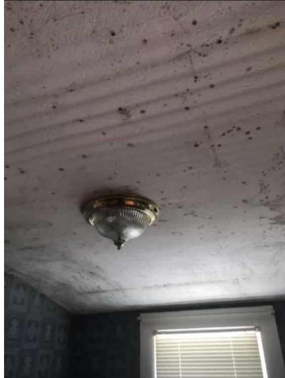
Figure 15 – 2 nd Floor Ceiling (black mold)
