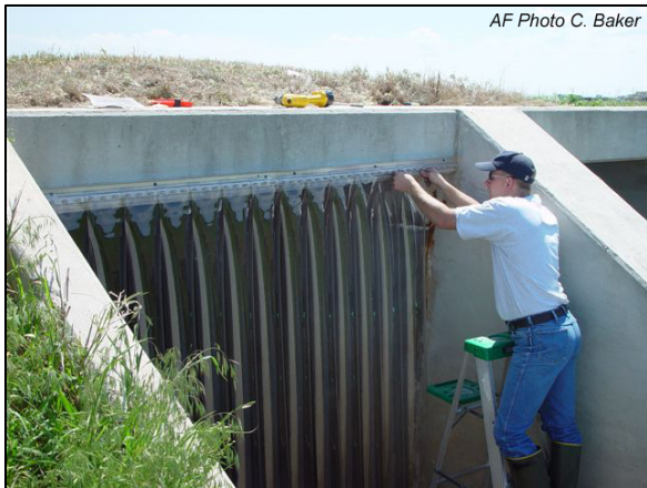
Vinyl curtains installed on culvert opening to discourage entrance and nesting by swallows (effective)
