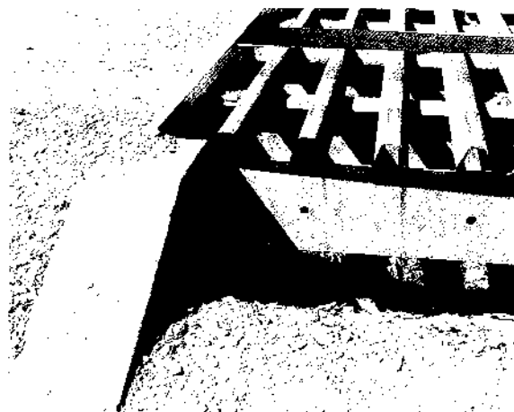
Concrete foundation cattleguard (detail).
