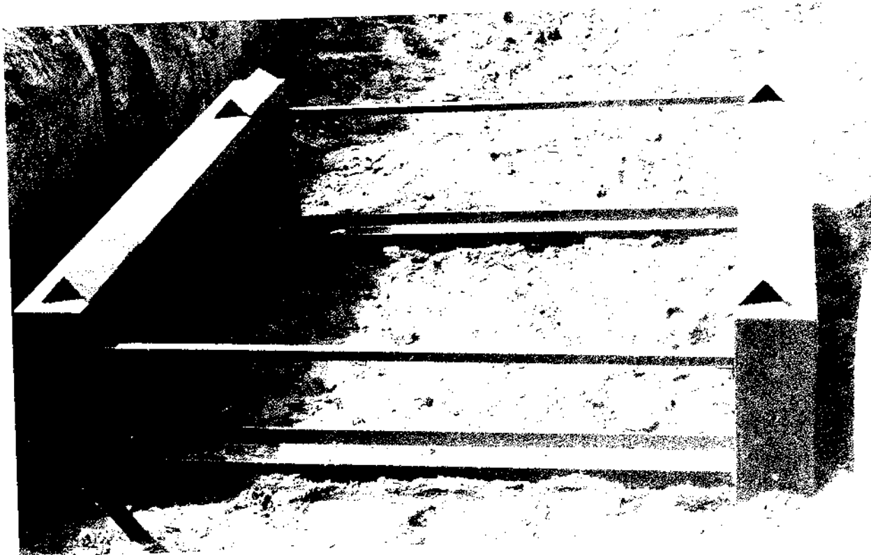
Typical steel foundation cattleguard under construction.
