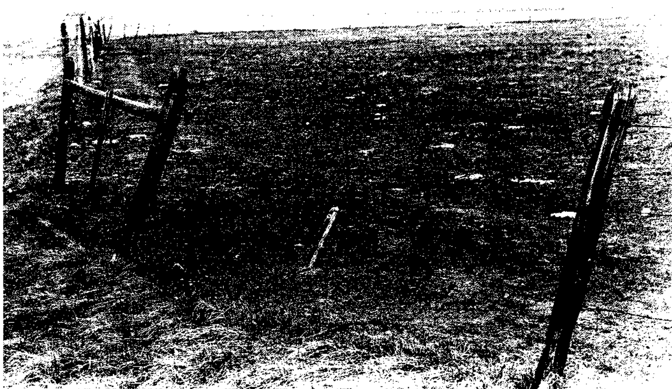
Dog leg failure.
