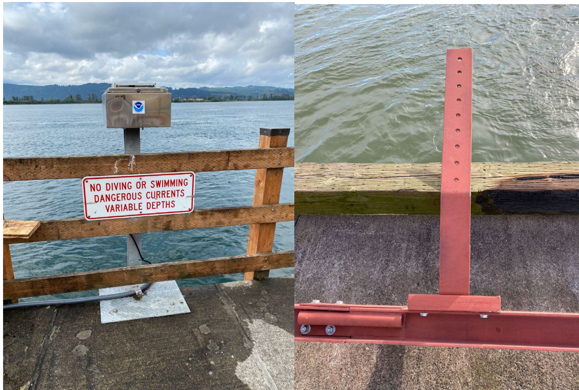
Figure 10 CLR 2217 Cathlamet City Dock, right panel shows an underwater bracket attached to an I-beam before installation.
