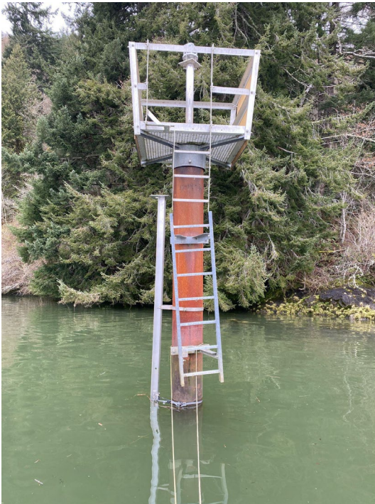
Figure 5 CLR 2211 Rockland Light 27 with I-Beam installed. Brackets are visible at the waterline and behind the ladder. Third bracket is below the waterline.
