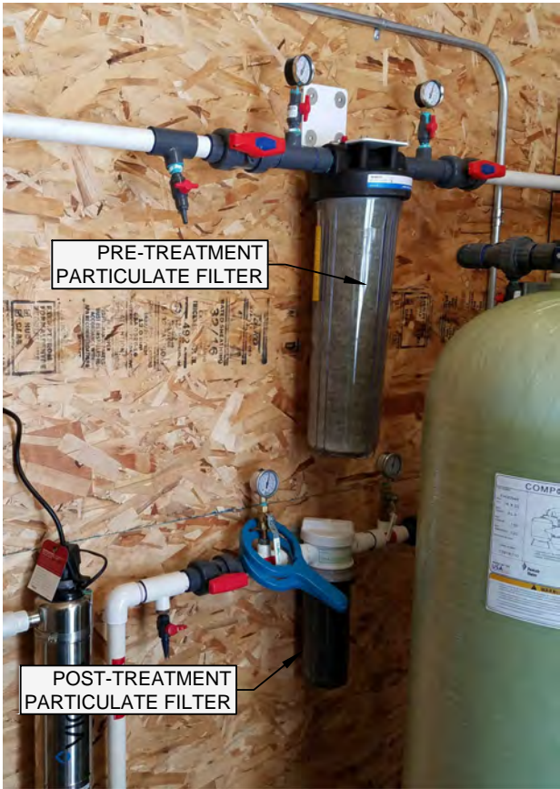
TREATMENT SYSTEM MANIFOLD.
