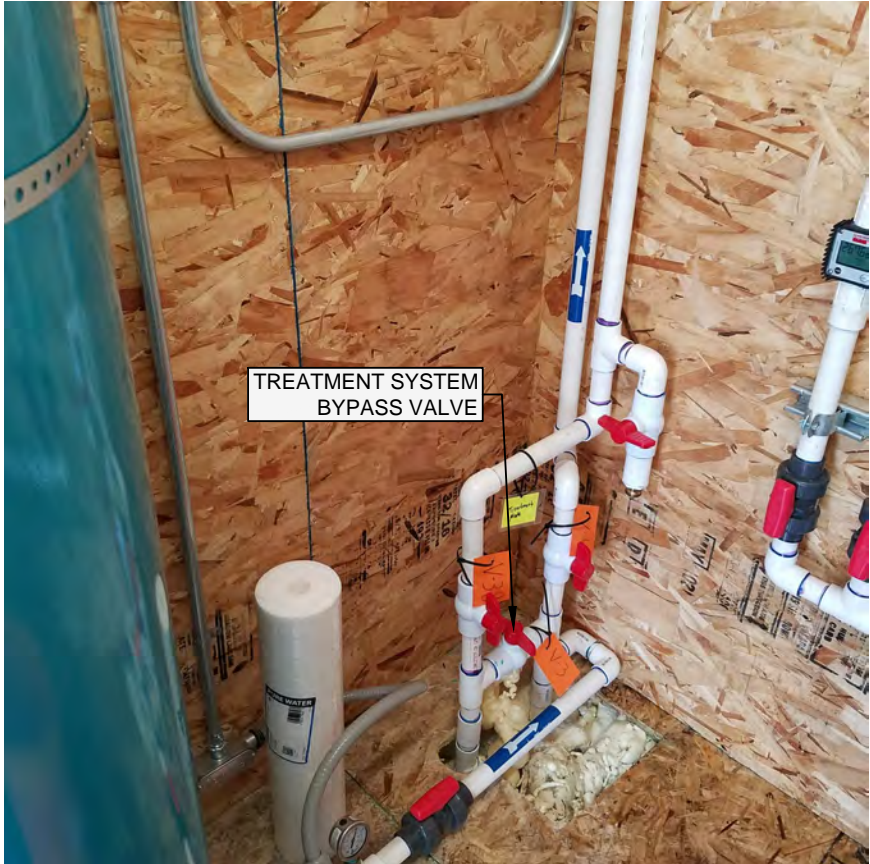
TREATMENT SYSTEM BYPASS MANIFOLD.
