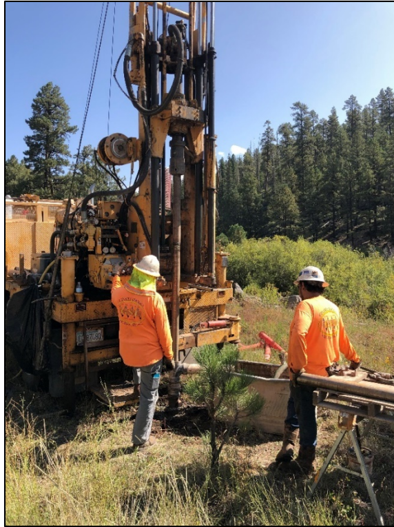
Photo 14: Rock Coring, Boring BH20-01
