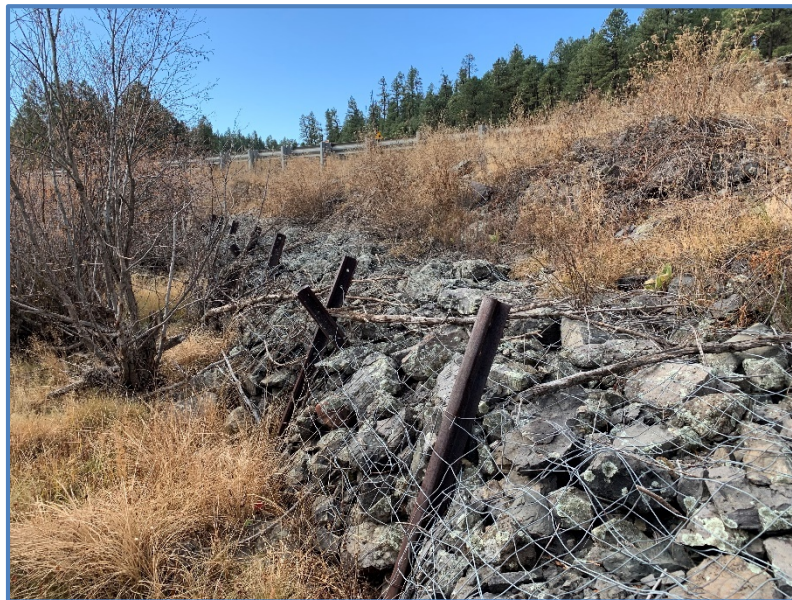
Figure 1 - Existing Rock Basket Structure
