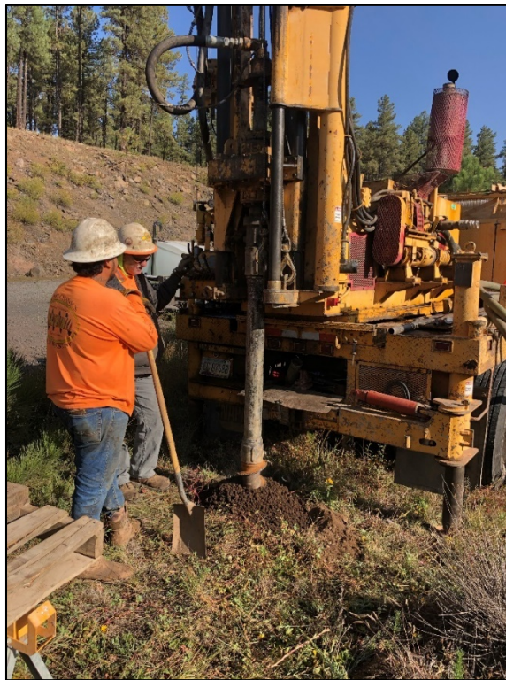
Photo 13: Hollow Stem Auger Drilling, Boring BH20-01
