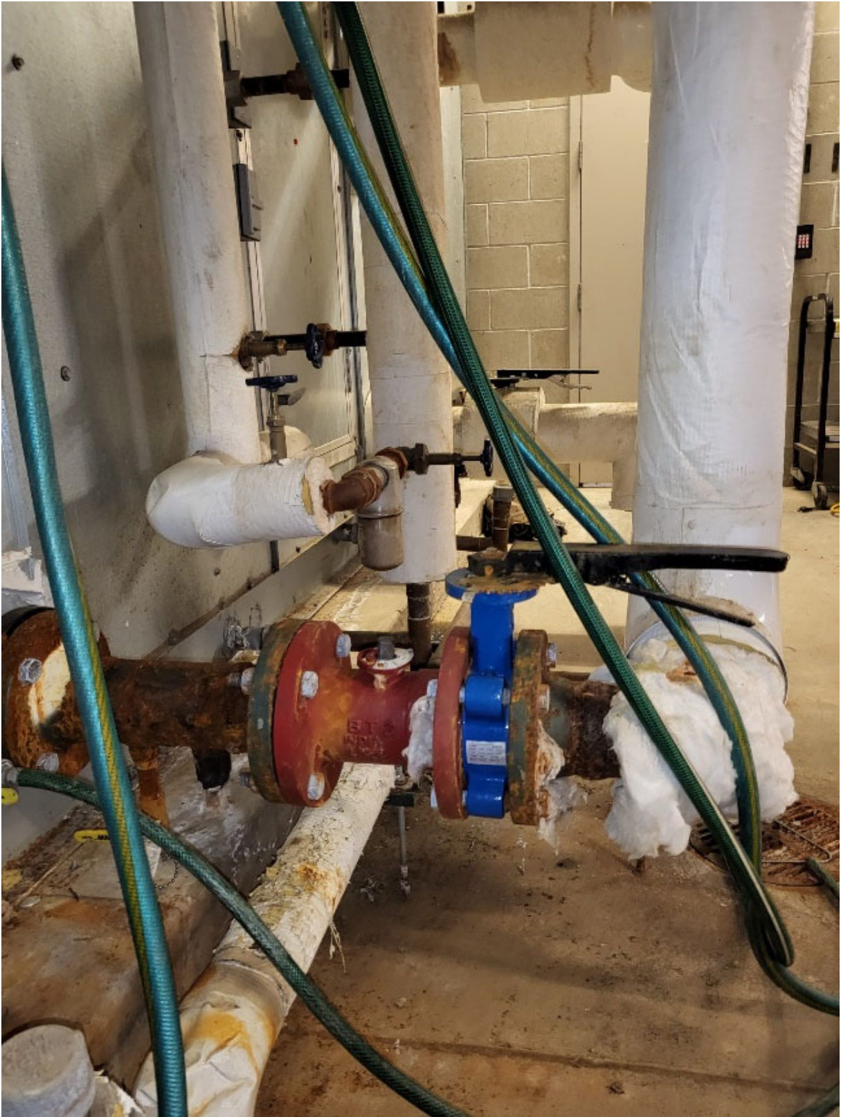
Photograph 5: View of chilled water return connection to lower coil at AHU-1.
