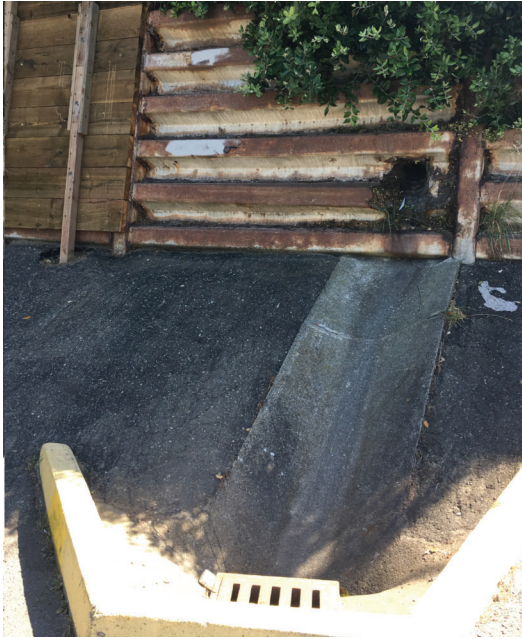
Figure 3.2: Parking Lot Runoff Outfall and Downstream Inlet
