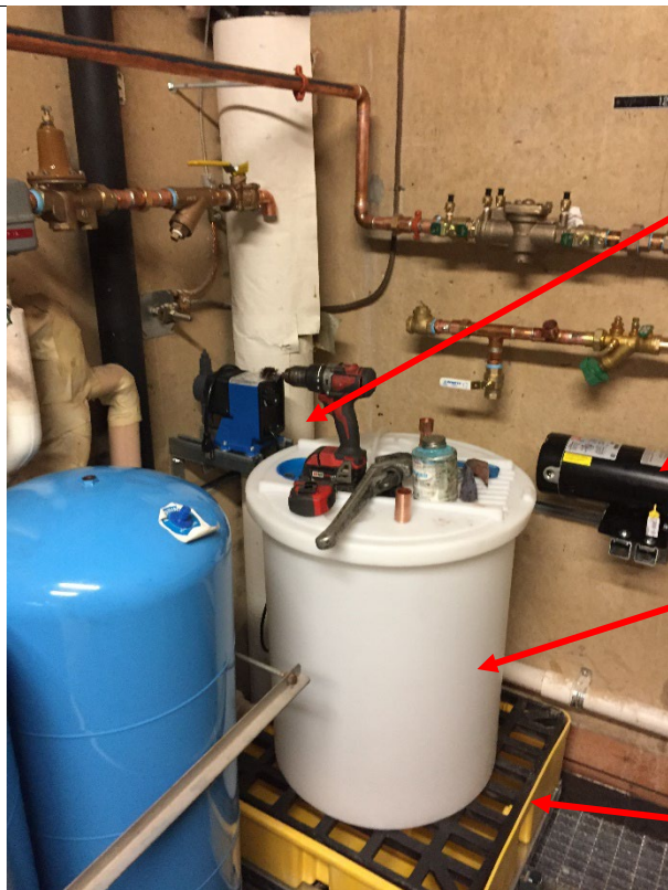
Figure 2: Chemical Storage Tank Setup on Containment (This is from another location) Setup may not be exactly the same.
