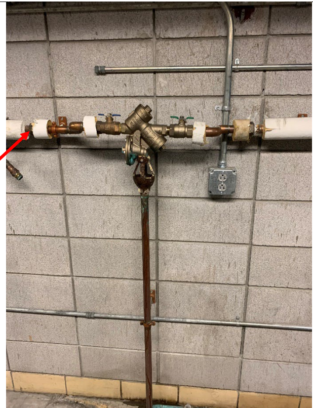
Figure 9: Existing Backflow Preventer (To be removed and Replaced)
