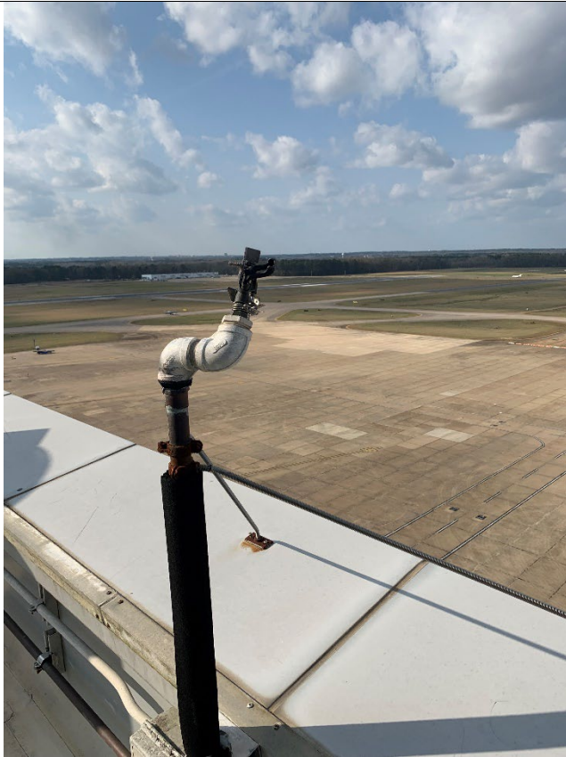
Figure 3: Typical Sprinkler Head to be Removed and Replaced (Typ. XX Locations)
