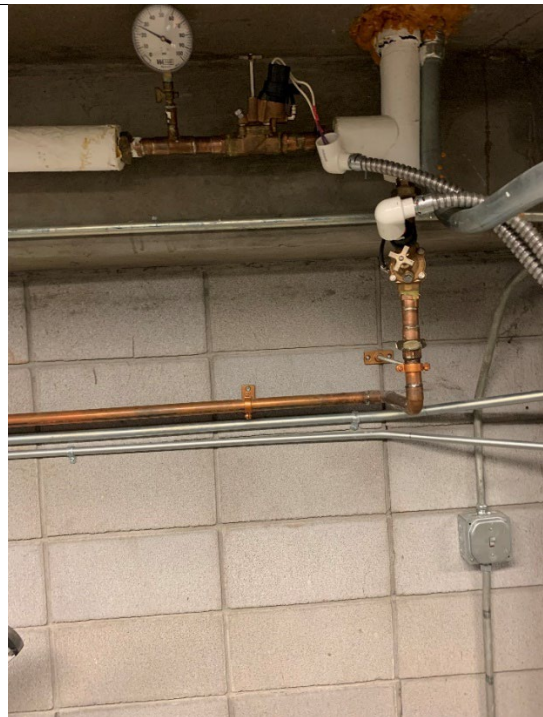
Figure 4: Typical Arrangement of Exterior Copper Piping and Sprinkler Solenoid. T Split in piping is for two heads on one zone. All new Piping shall be insulated and covered with Aluminum Jacket. Electrical Junction boxes may be reused, however all new liquidtight metal flex shall be used.
