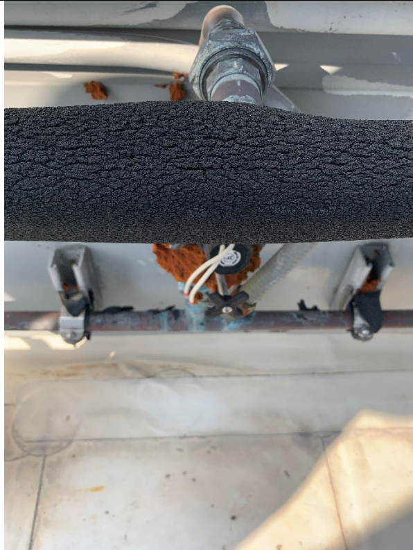
Figure 15: Typical View of water line on Roof area, and solenoid. (To be Replaced)
