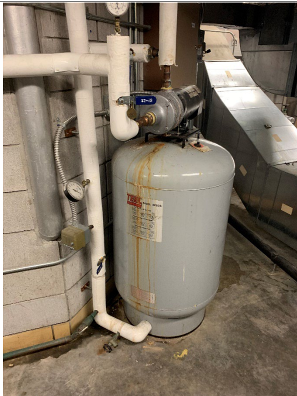
Figure 1: Existing Pump and Bladder Tank Assembly to be Removed and Replaced.
