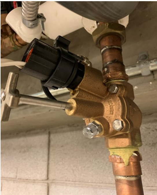
Figure 5: Typical Solenoid Valves in Window Wetting Pump Area to Be Removed/Replaced.
