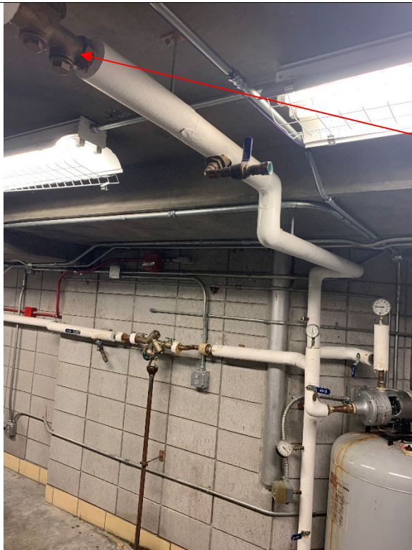
Figure 10: View of incoming cold water supply and existing water tank (T-2) to be removed/replaced. View of water line overhead crossing room. (To be replaced)
