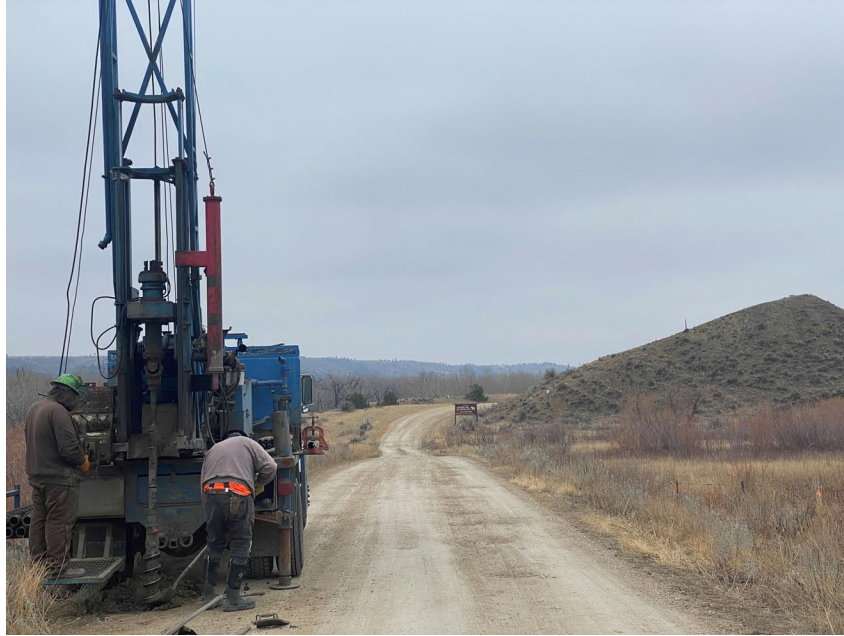
Site 1- Siparyann Creek Crossing; Boring B-02 looking west, note depression in roadway near planned concrete ford location Sta. 19+50 to 20+50
