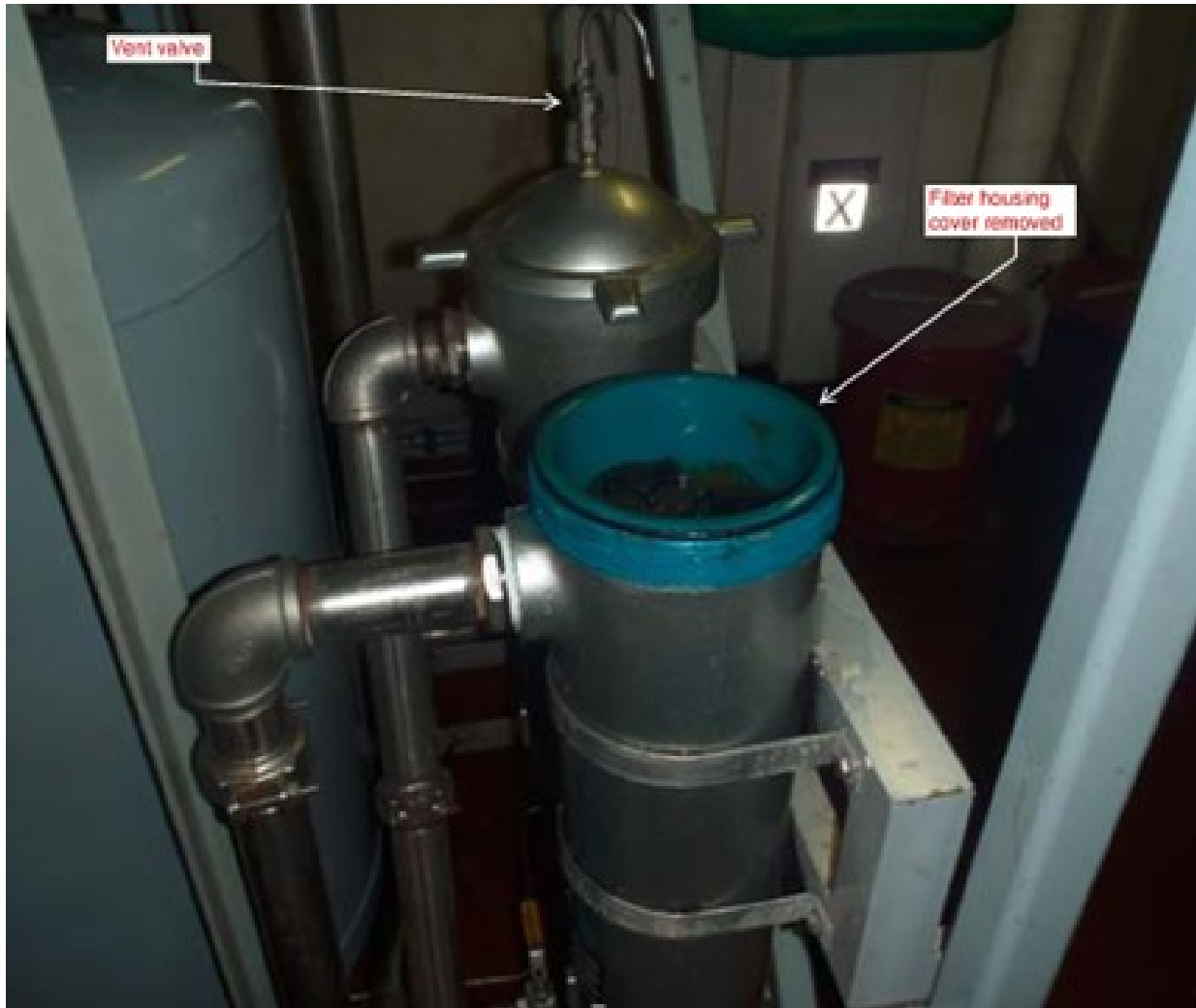
FIGURE 3. 5 MICRON AND 20 MICRON FILTER HOUSINGS
